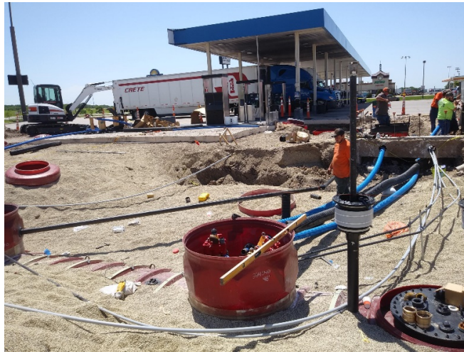
Figure I.7-2. The 24-7 Travel Store in Salina, Kansas installed underground tanks for bio-diesel storage (Photo Credit: Tami Alexander)
