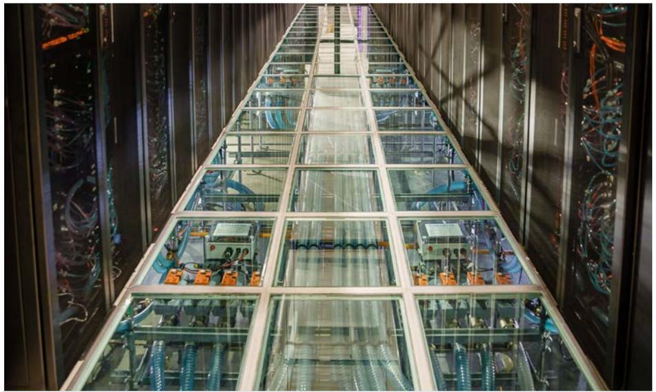
Water flows through flexible tubes and pipes visible through glass panels above two rows of Attaway's compute racks. At the end of the racks, cooling distribution units control water flow and rates. *Image Credit: Sandia.*
