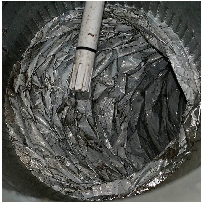
Figure 27. Photo of inside of X_1 duct from test home 3 (representative of the X_1 duct in other homes)
