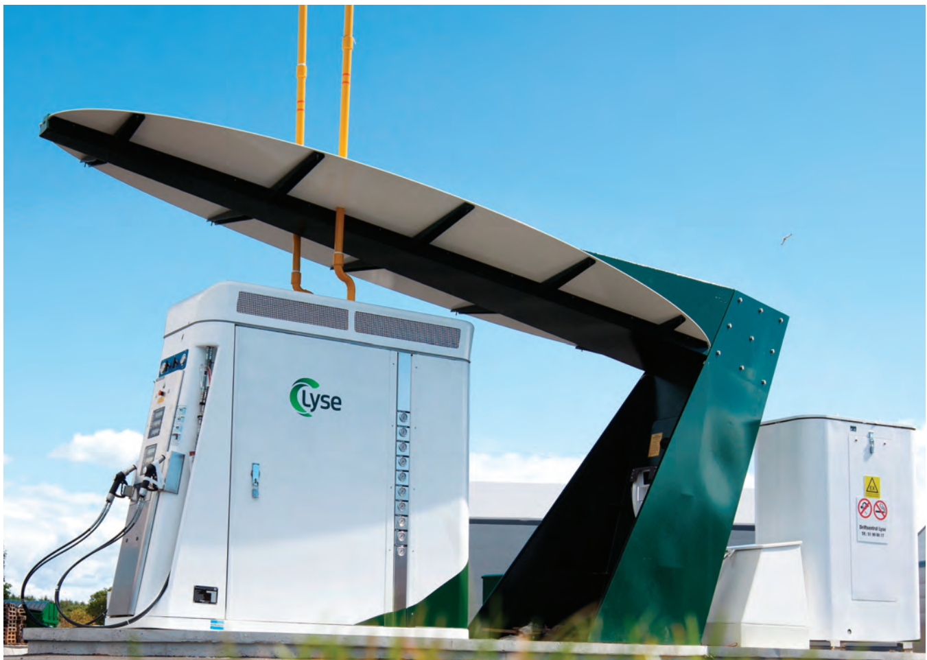
Figure 14-9. Modular CNG Dispensing Unit
