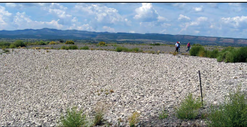
Bluewater, New Mexico, Disposal Site.
