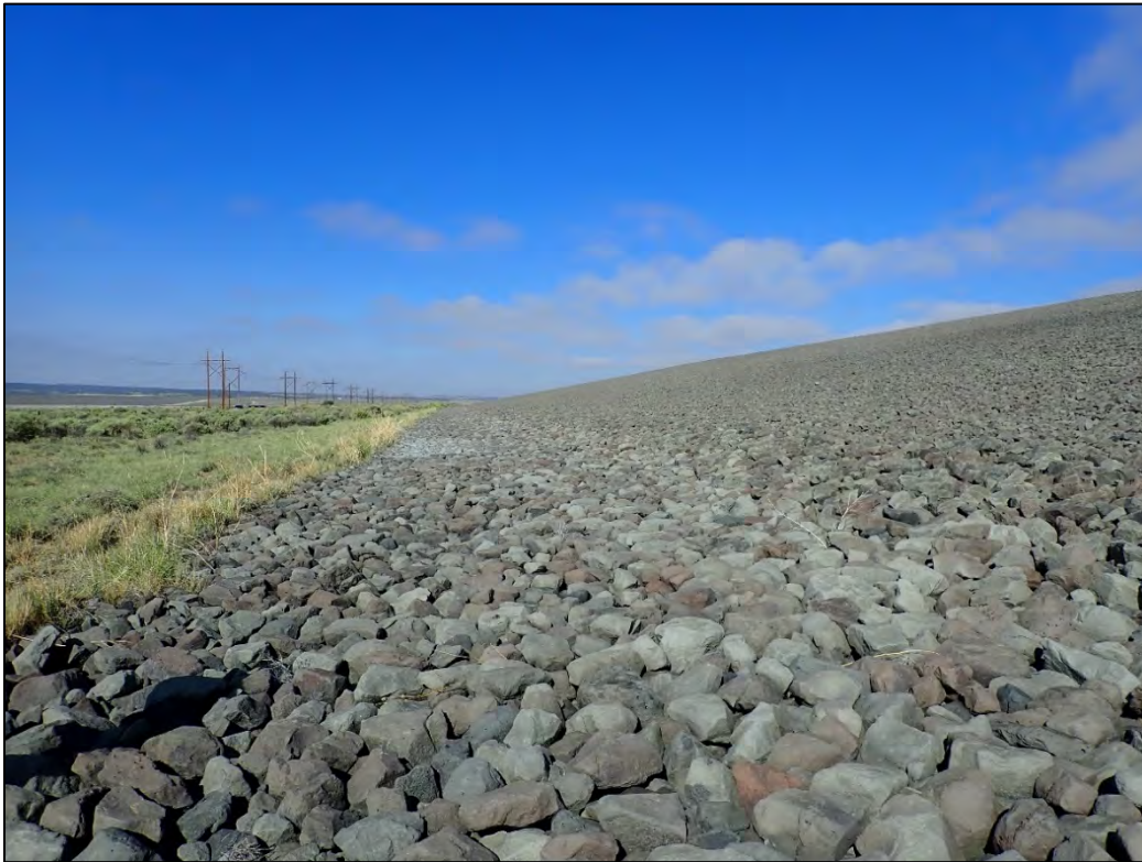
PL-9. Base of South Side Slope of the Disposal Cell
