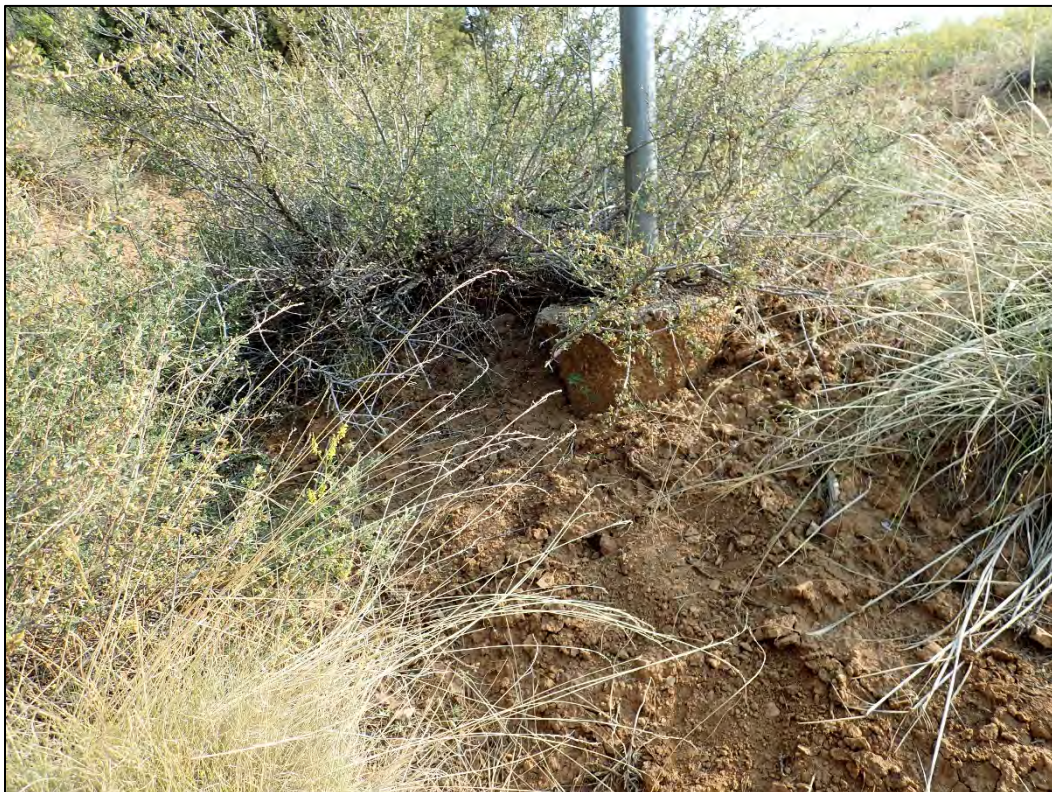
PL-2. Perimeter Sign P79 Undercut by Erosion
