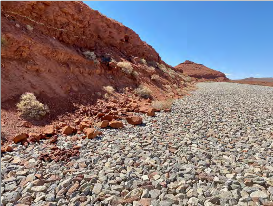
PL-9. Sloughed Rock Area on South Apron
