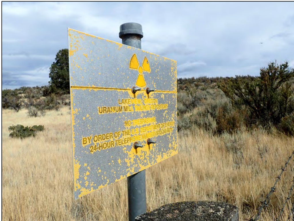
PL-2. Faded Perimeter Sign P11
