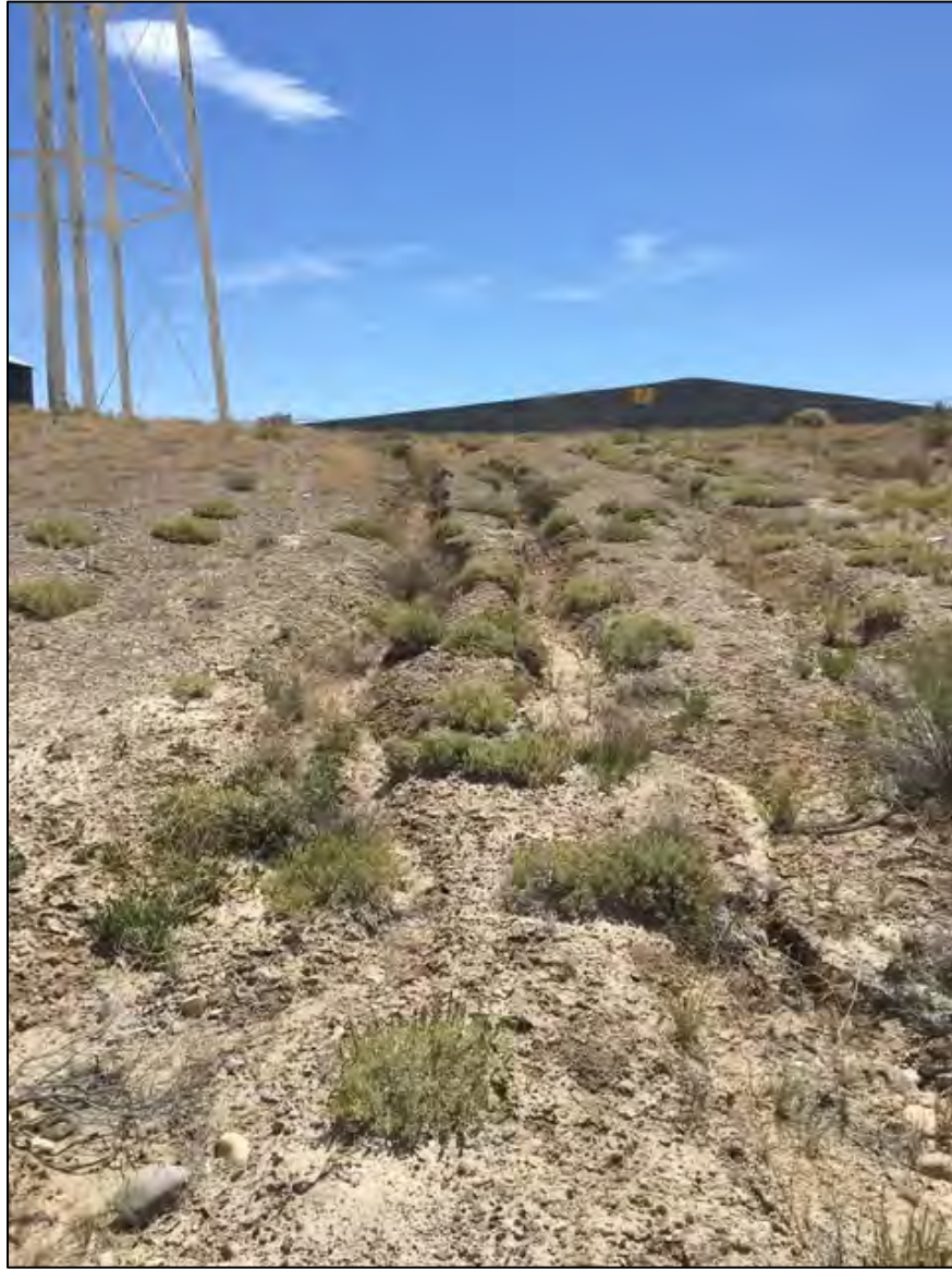
PL-11. Gullies Downslope of Water Tower (Offsite)
