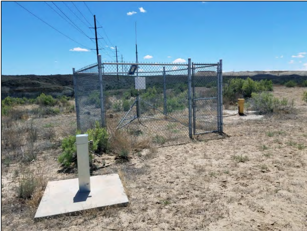
PL-6. Monitoring Wells 0194 and 0582 (with the System Operation and Analysis at Remote Sites [SOARS] Station in Background)
