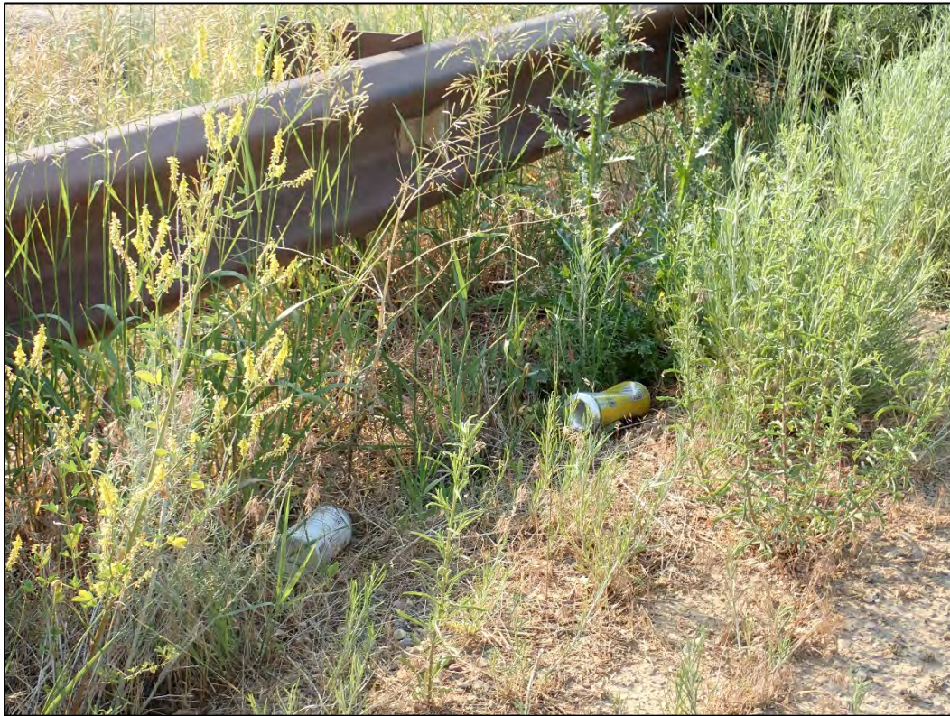
PL-12. Trash Dumped Near Site Entrance
