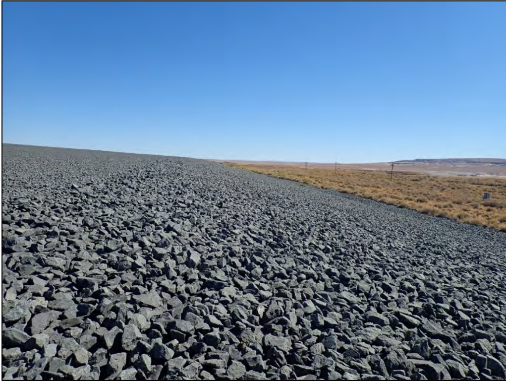
PL-7. Disposal Cell Top and Side Slope
