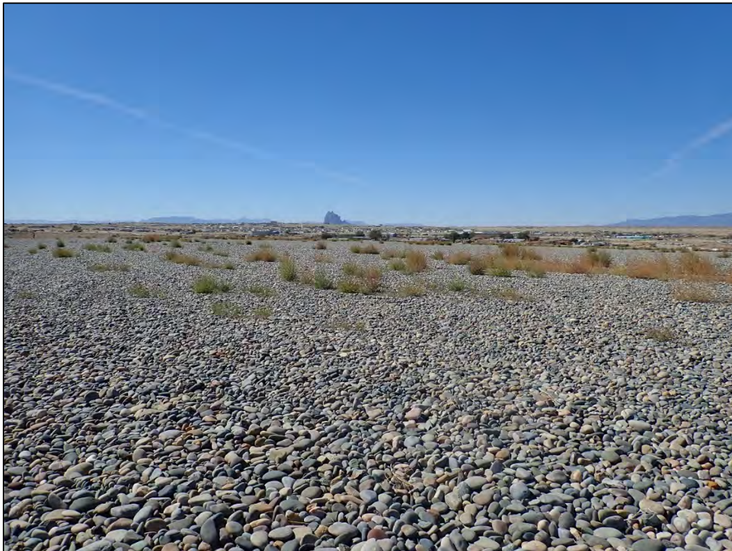
PL-6. Disposal Cell Top Slope with Growing Vegetation
