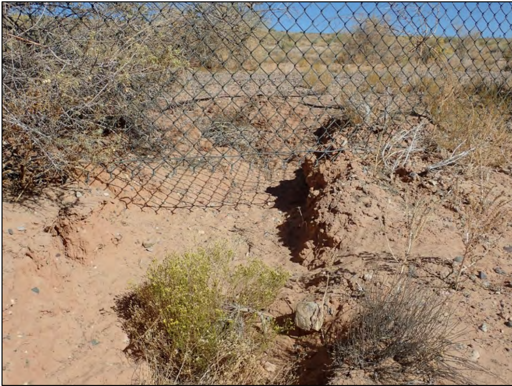
PL-3. Erosion Under Fence
