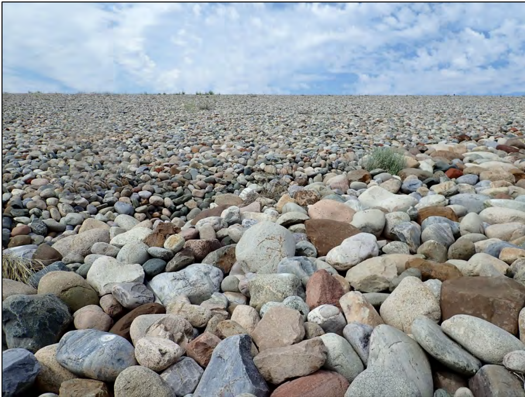
PL-8. Linear Depression in Cell Toe Slope
