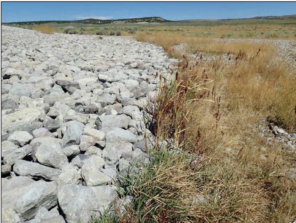
PL-10. Cattails Adjacent to Disposal Cell Toe Slope and Apron
