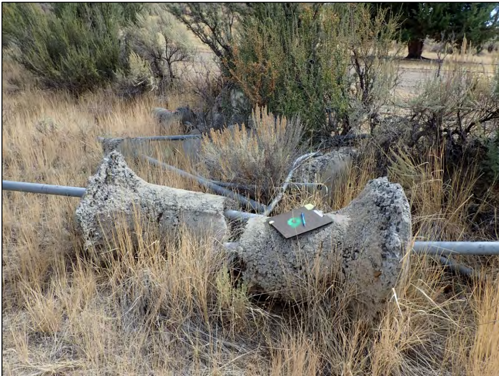
PL-11. Old Fence Posts with Concrete Bases
