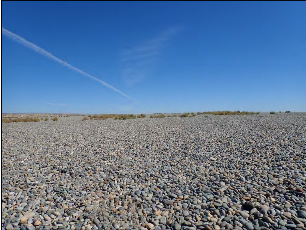
PL-5. Disposal Cell Top Slope
