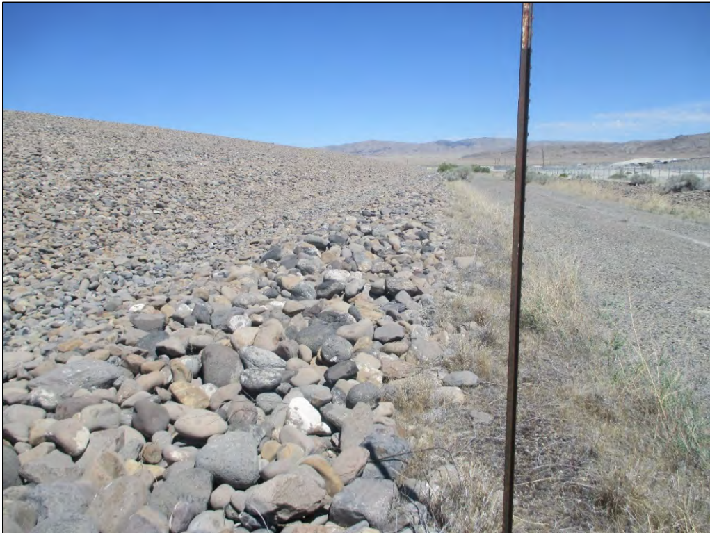
PL-4. Disposal Cell, South Side Toe Drainage
