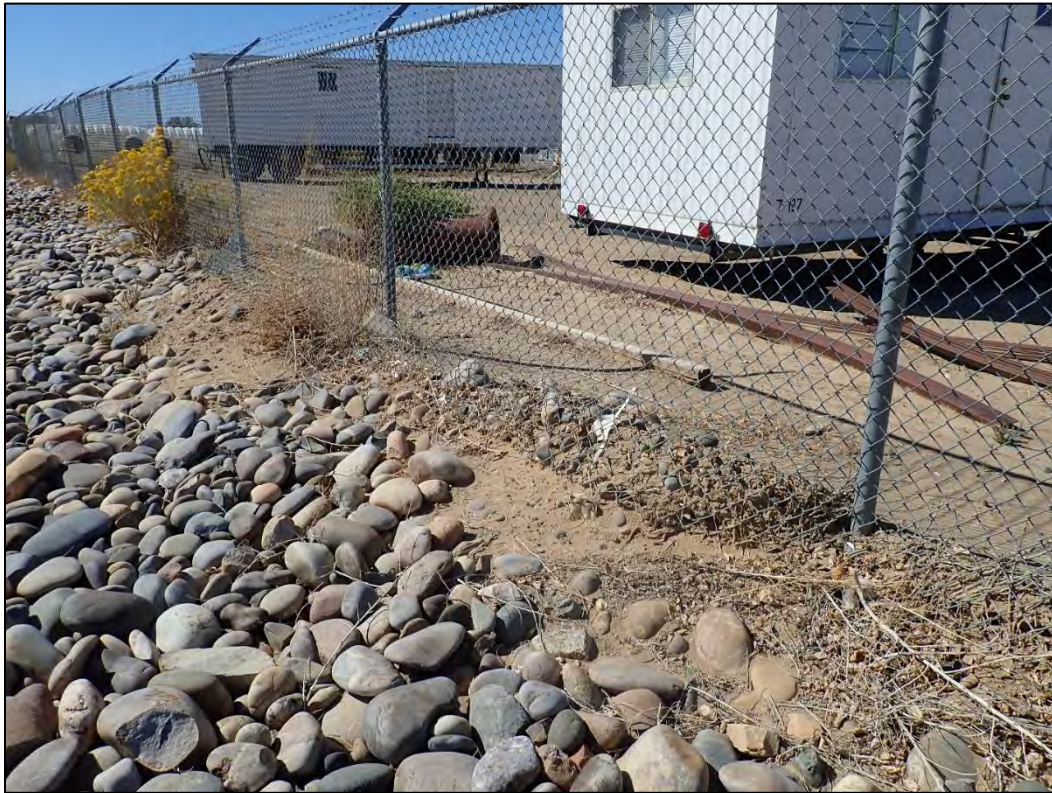
PL-7. Sediment Accumulation Near Southwest Fence Line
