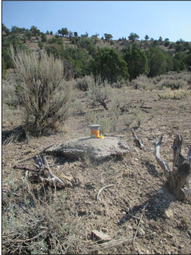
PL-3. Boundary Monument BM-18 with Undercutting
