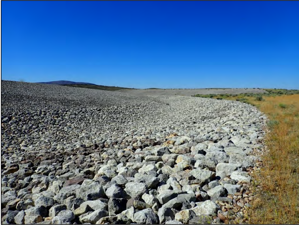
PL-11. Diversion Channel No. 1 and North Side Slope of Disposal Cell
