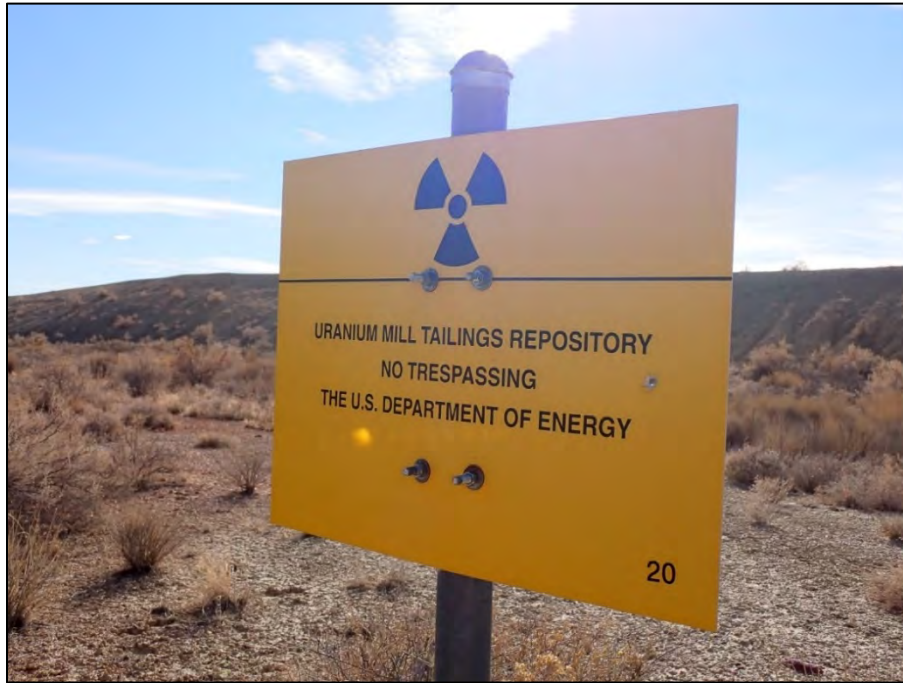
PL-5. Perimeter Sign P20 with Bullet Damage
