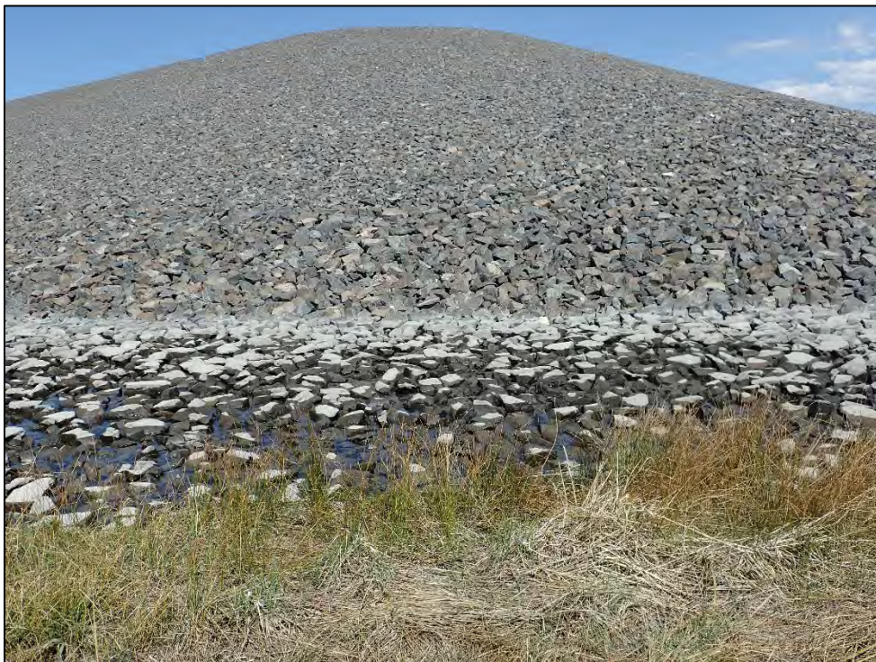
PL-6. Water in Cell Apron, Southeast Corner
