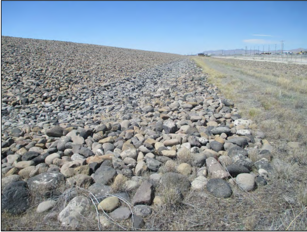
PL-5. Disposal Cell, East Side Toe Drainage
