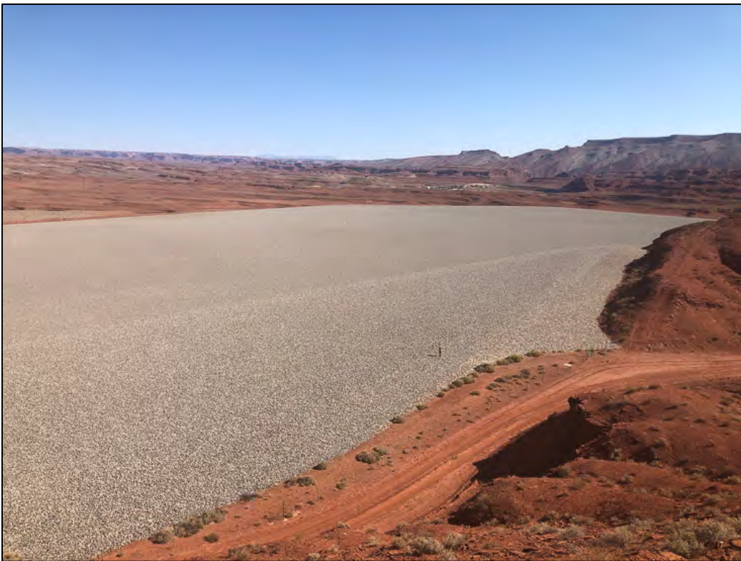
PL-8. Top of Cell – Looking Northeast
