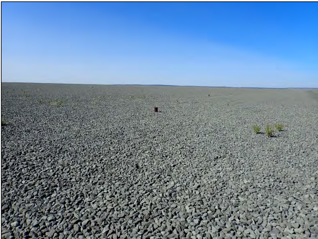
PL-8. Settlement Plate 4 and Top Slope of the Disposal Cell
