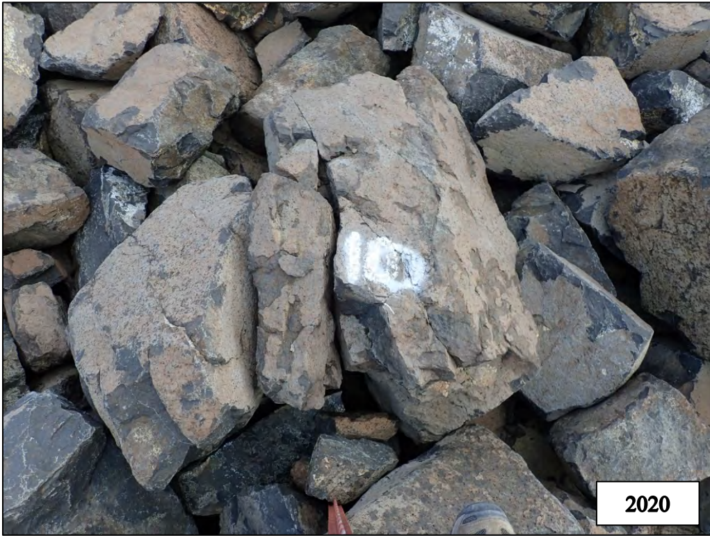
PL-9a. Riprap Monitoring Location Number 10 in Energy Dissipation Area–2020
