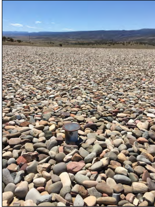
PL-4. Settlement Plate on Disposal Cell
