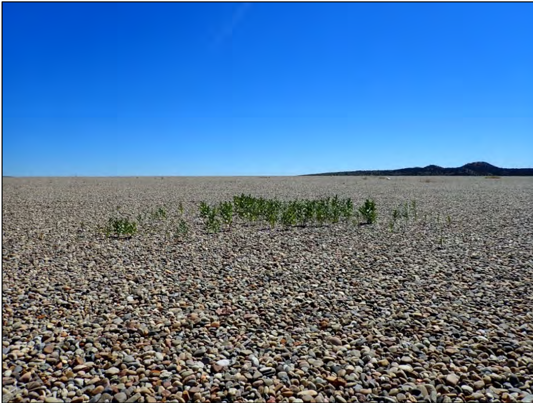
PL-9. Vegetation on Top Slope of Disposal Cell
