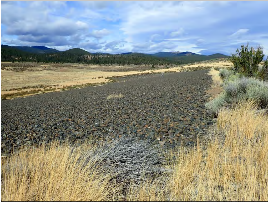
PL-7. Contact Boundary West Side Slope and South Top Corner with Encroaching Vegetation
