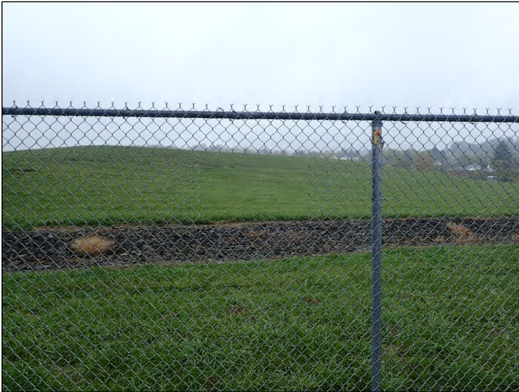
PL-3. Disposal Cell with Missing Perimeter Sign P1
