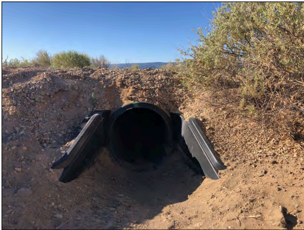
PL-8. Cleaned-Out Culvert
