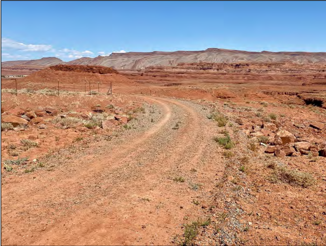
PL-13. Road Repair Area
