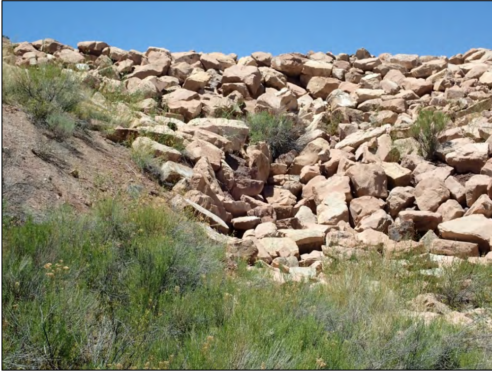
PL-9. Spillway Above Interceptor Channel
