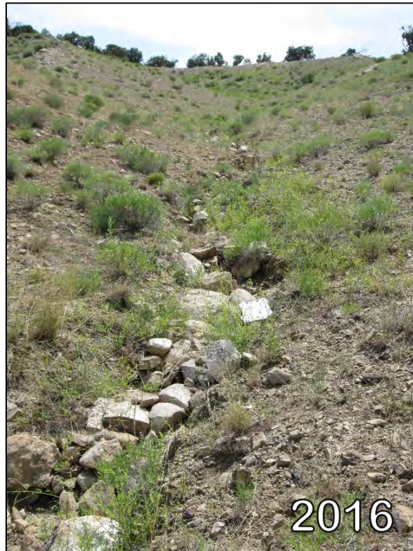
PL-7b. Minor Gully Erosion at Interceptor Trench in 2016
