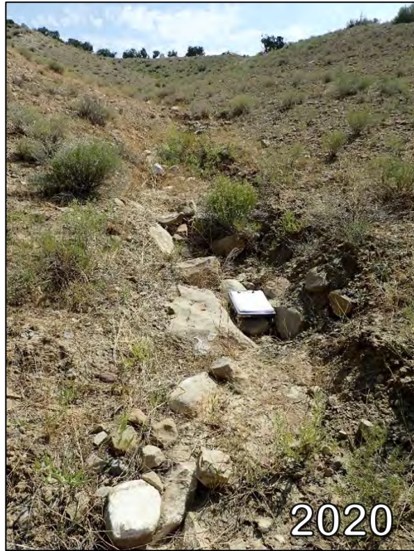
PL-7a. Minor Gully Erosion at Interceptor Trench in 2020
