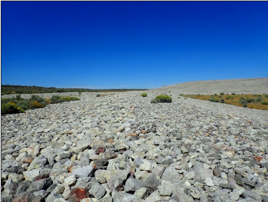
PL-12. Diversion Channel No. 1
