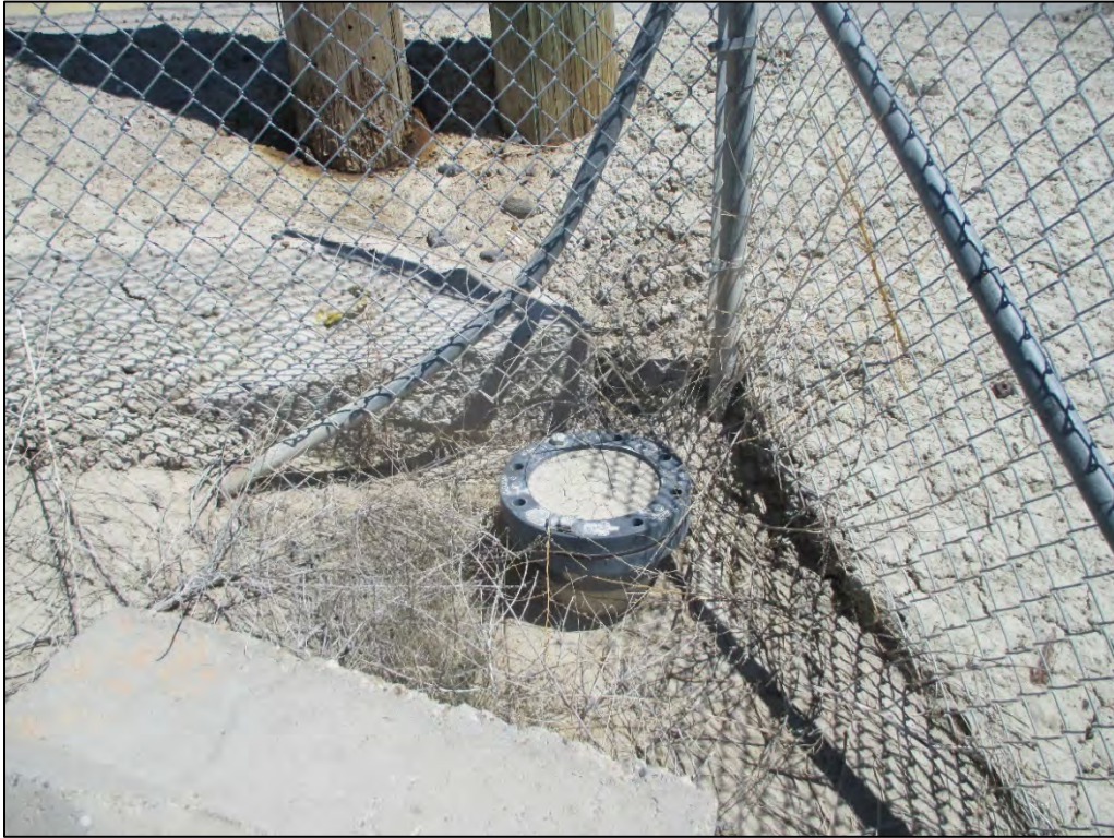
PL-3. Protective Casing on Boundary Monument BM-3
