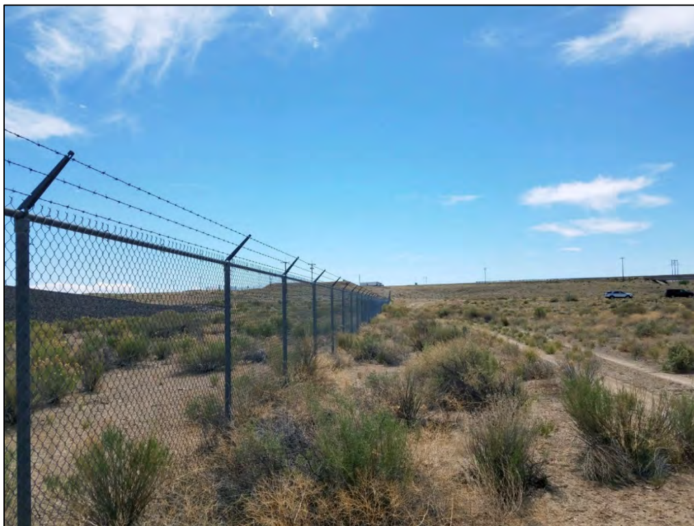
PL-2. Chainlink Security Fence
