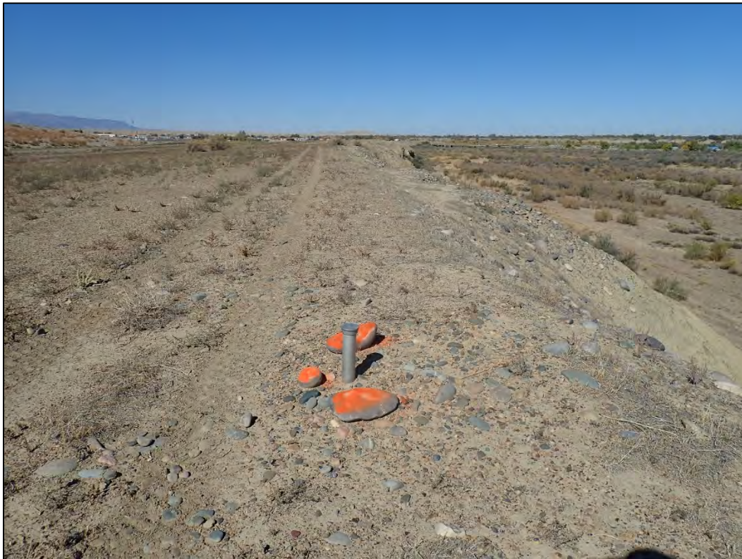
PL-4. Erosion Control Marker E-2
