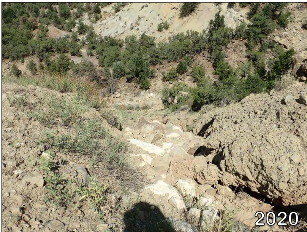
PL-8a. Major Gully Erosion in Interceptor Trench Outfall in 2020
