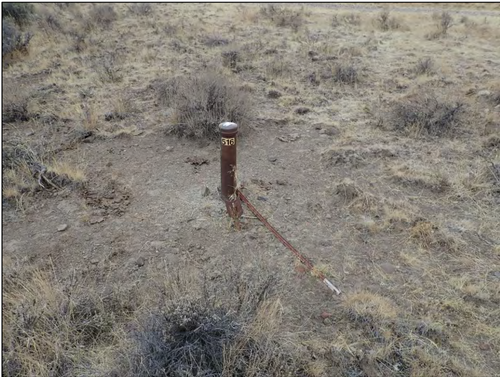
PL-6. Broken T-Post near Monitoring Well 0516
