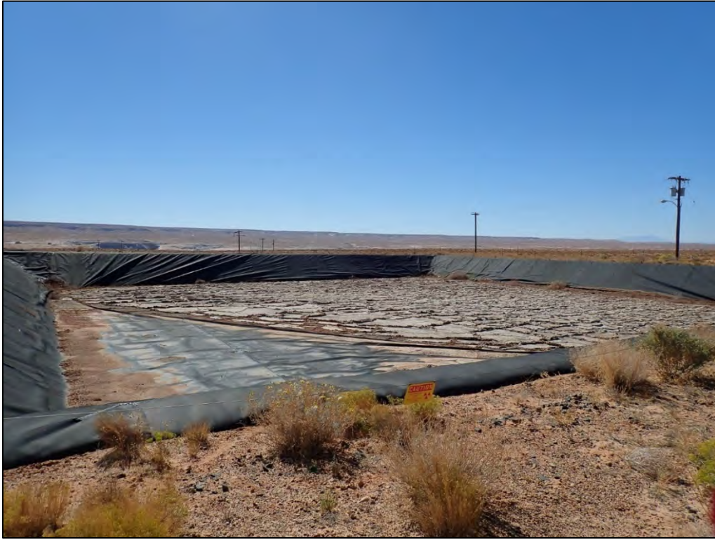
PL-9. Inactive, Lined Evaporation Pond
