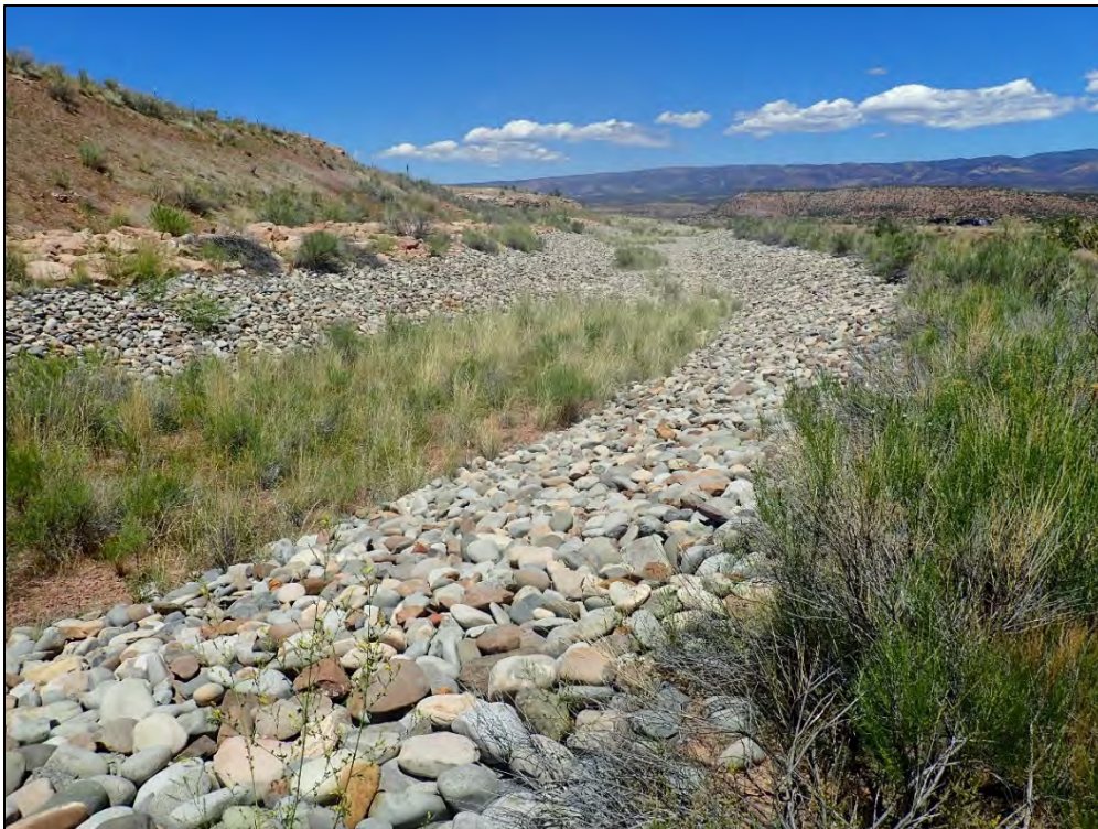
PL-8. Sediment Accumulation and Vegetation in Interceptor Channel
