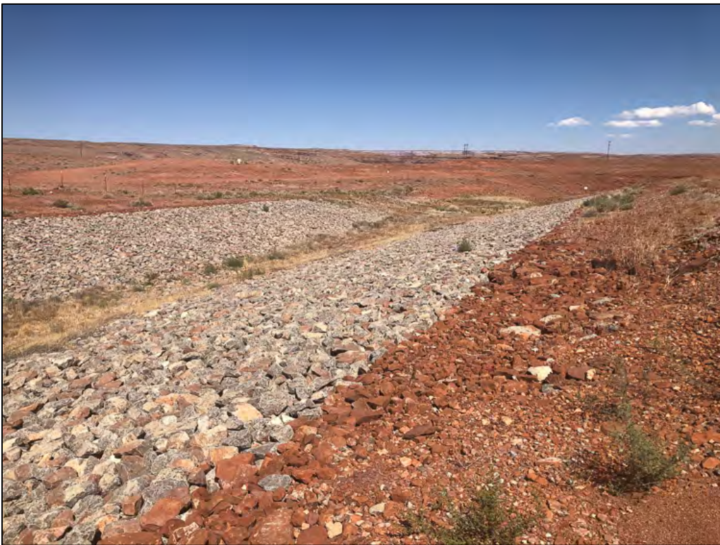
PL-10. West Diversion Channel
