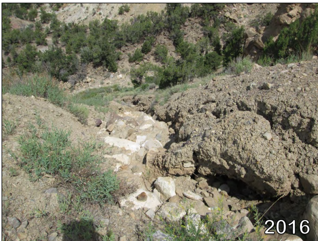
PL-8b. Major Gully Erosion in Interceptor Trench Outfall in 2016
