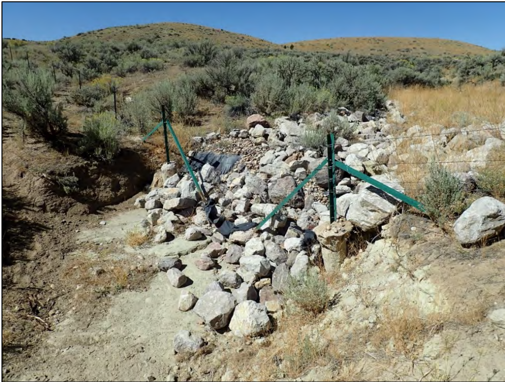
PL-13. Perimeter Fence near Outlet to Diversion Channel No.1
