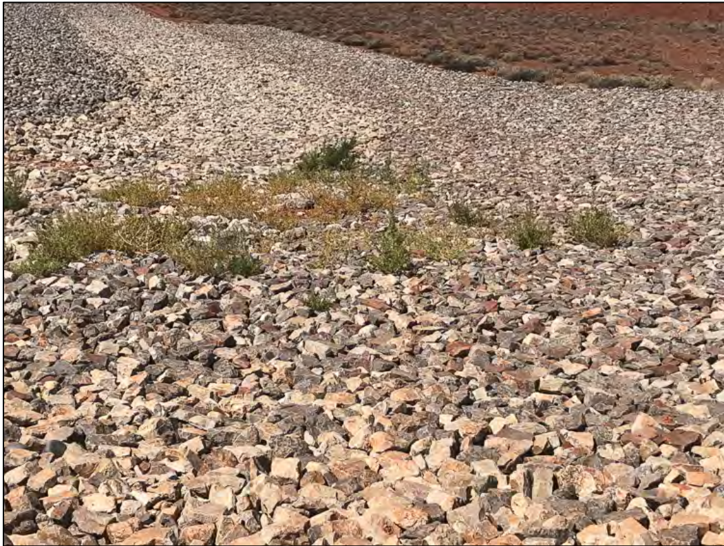
PL-11. Northeast Toe Drain
