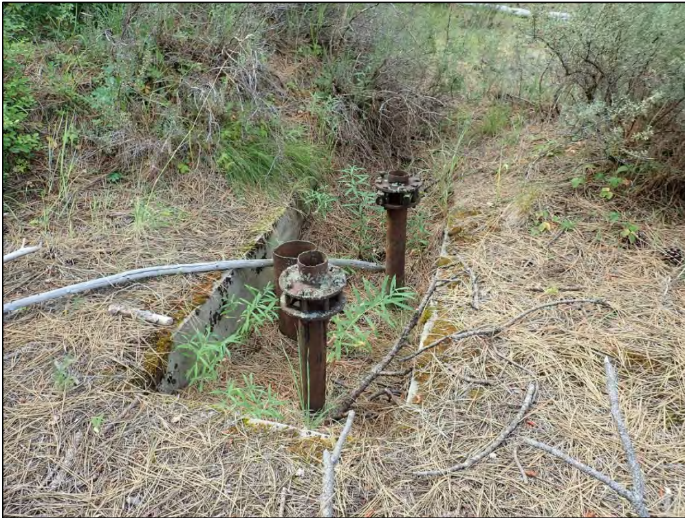
PL-6. Concrete Structure and Water Piping Remains
