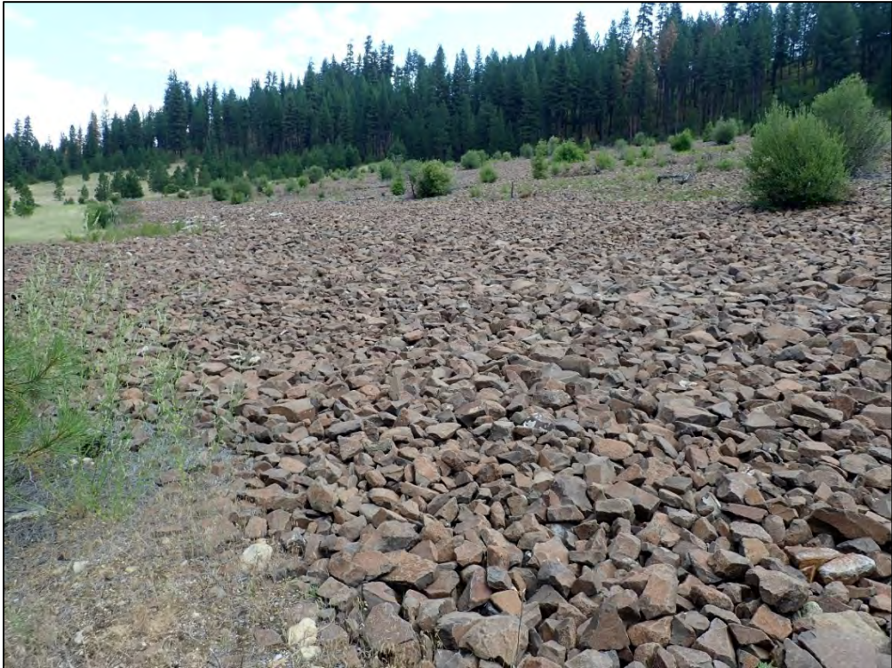
PL-5. Vegetation on Disposal Cell Cover
