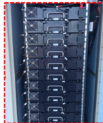
Battery Rack in Enclosure
