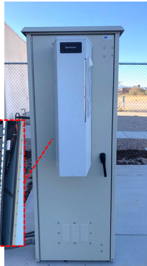
Outdoor Battery Enclosure
