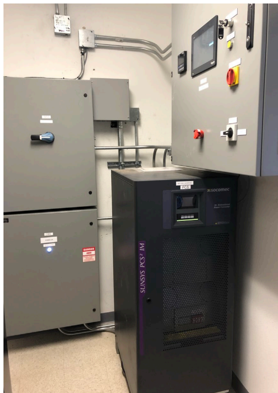
Battery Inverter and Controller
