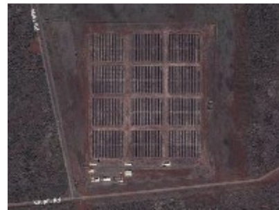
1.2 MW PV Plant
