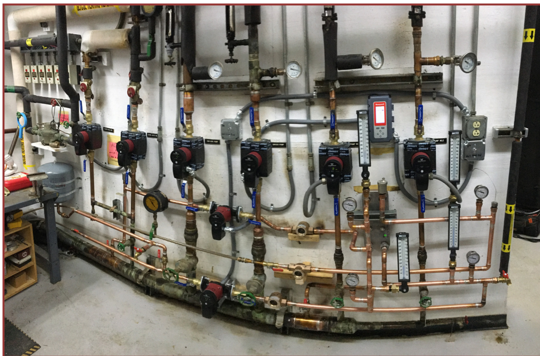
Figure 3: New Grundfos pumps and new glycol heating loop in Northway, Apr 2018. Photo courtesy of TCC / David Pelunis-Messier. materials and the roof was replaced before the photovoltaic system installation.
