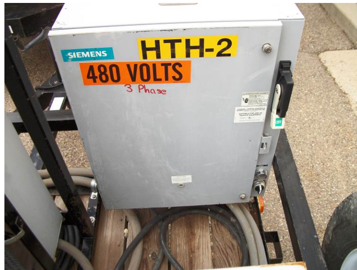
Figure 4. Typical Disconnect Switch
