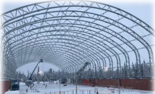
Construction on a new munitions storage facility on Eielson Air Force Base. In order to build on the spot, construction workers had to melt the permafrost underneath. (Sara Karlovitch)
