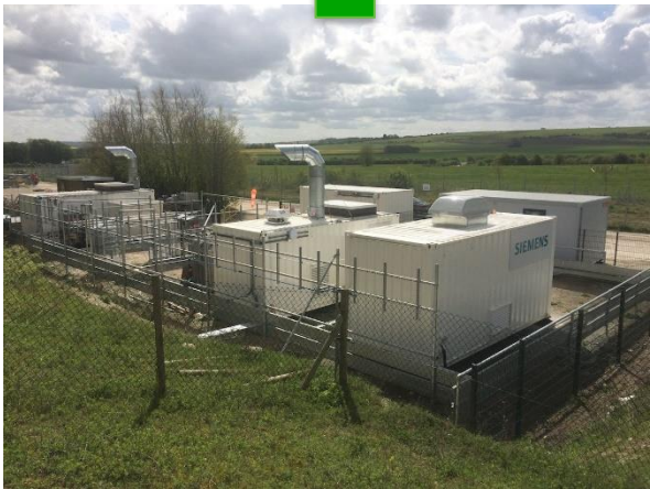
Siemens Green Ammonia Demonstrator at the Rutherford Appleton Laboratory (UK) 10 metric tons per year
