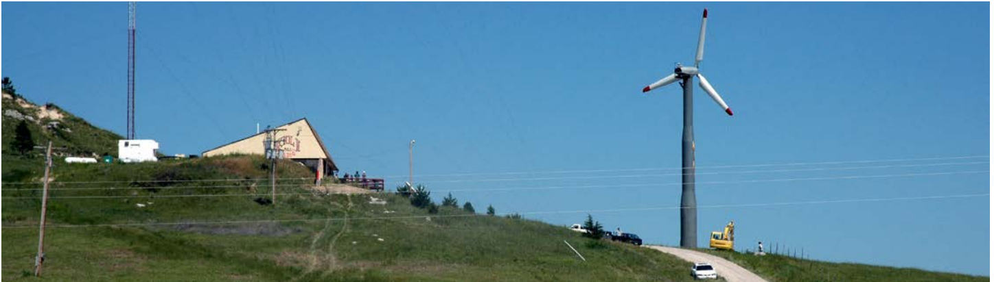
The Lakota Nation installed a 65-kW Nordtank turbine that annually supplies 120 MWh of power to KILI, the Pine Ridge Reservation radio station known as the voice of the Lakota Nation in South Dakota. Photo by Bob Gough, NREL 16258
