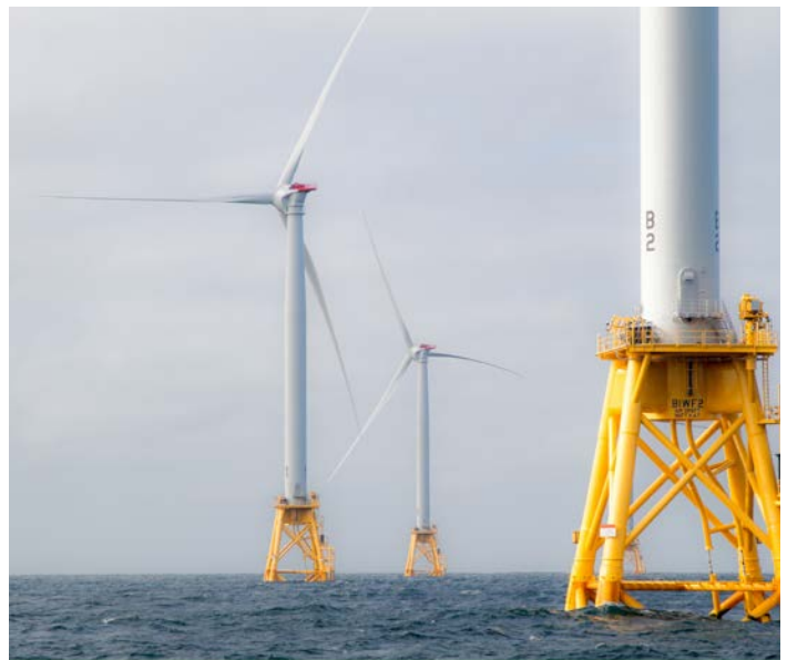
The Block Island Wind Farm, the first U.S. offshore wind farm, represents the launch of an industry that has the potential to contribute significantly to a reliable, stable, and affordable energy mix. Photo by Dennis Schroeder, NREL 41193
