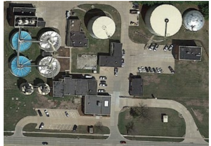
Water treatment facility
