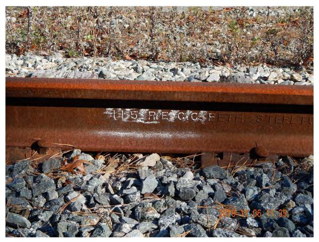
Figure 2-424. 115-lb. Rail at Industrial Spur at Second Potential Rail Transload Location (2019)
