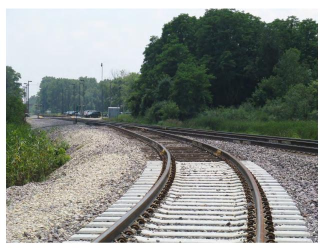
Figure 2-148. Junction of Zion On-site Rail Spur with Union Pacific Railroad Showing Concrete Rail Ties (2013)
