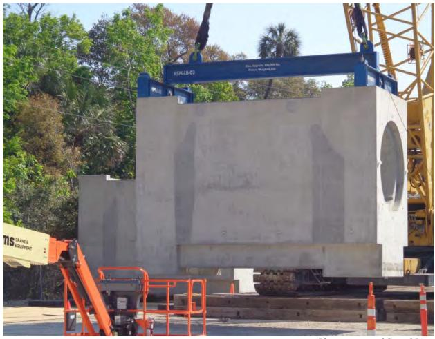
Figure 2-188. Horizontal Storage Module Being Unloaded from Railcar (2015)
