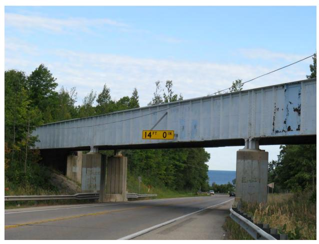
Figure 2-76. Low Overhead Clearance Abandoned Railroad Bridge on U.S. 31 (2013)
