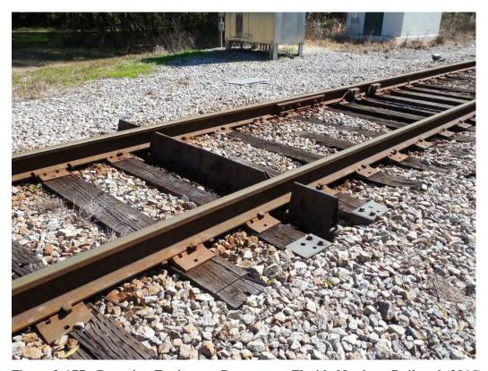
Figure 2-177. Dragging Equipment Detector on Florida Northern Railroad (2015)
