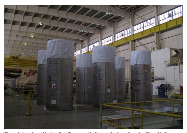
Figure 2-141. Spent Nuclear Fuel Transportable Storage Canisters Staged at Zion (2013)
