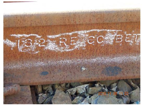
Figure 2-413. 132-lb. Rail at First Potential Rail Transload Location (2019)
