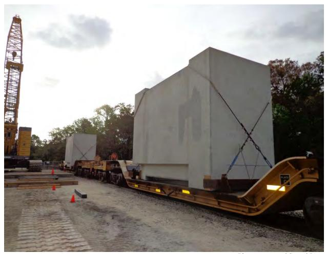
Figure 2-186. Two Horizontal Storage Modules Loaded on Railcars (2015)
