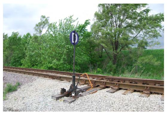
Figure 2-347. Derailer at Entrance to Cargill Industrial Spur (2017)
