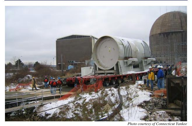
Figure 2-43. Connecticut Yankee Reactor Pressure Vessel Being Loaded onto Barge
