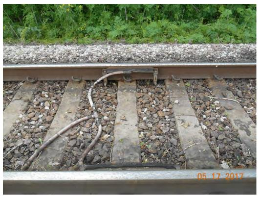
Figure 2-350. Close-up of Greaser Activators on Cargill Industrial Spur (2017)
