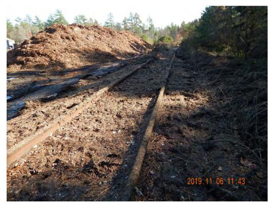
Figure 2-422. Industrial Spur at Second Potential Rail Transload Location Covered with Compost (2019)
