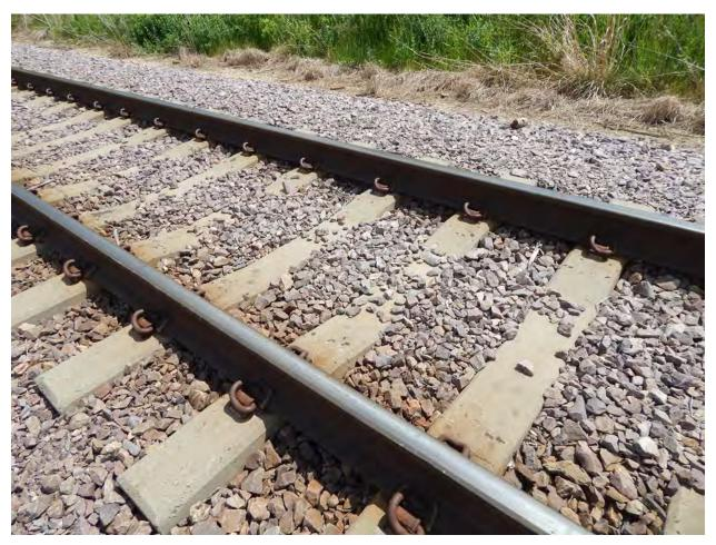
Figure 2-342. Rail, Concrete Ties, and Pandrol Clips on Cargill Industrial Spur (2017)
