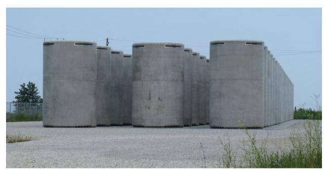
Figure 2-140. Vertical Concrete Storage Casks Staged at Zion (2013)
