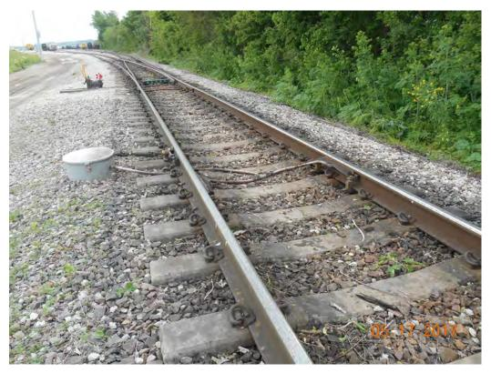
Figure 2-349. Derailer and Greaser on Cargill Industrial Spur (2017)
