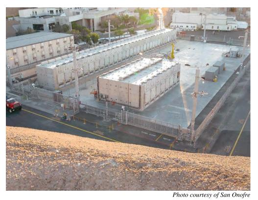
Figure 2-275. Original San Onofre Independent Spent Fuel Storage Installation (2009)
