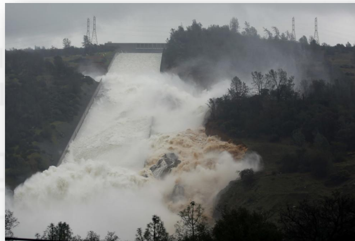
Oroville Spillway Failure, 2017
