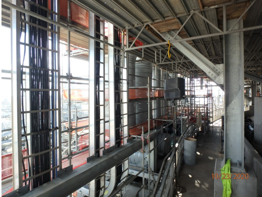
LNG Tank B waterfall piping insulation in progress
