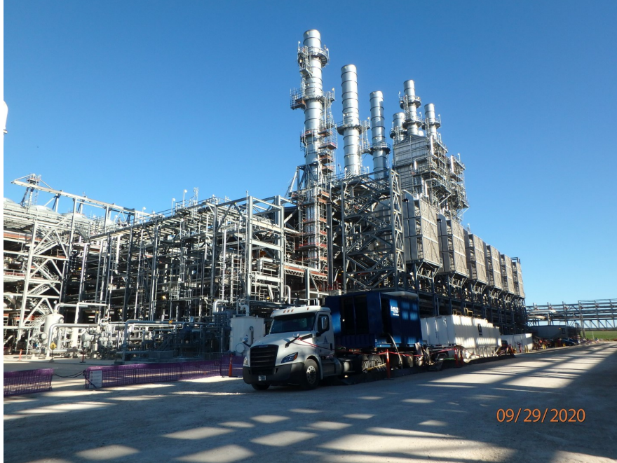
Aqua milling of inlet air chilling system in progress
