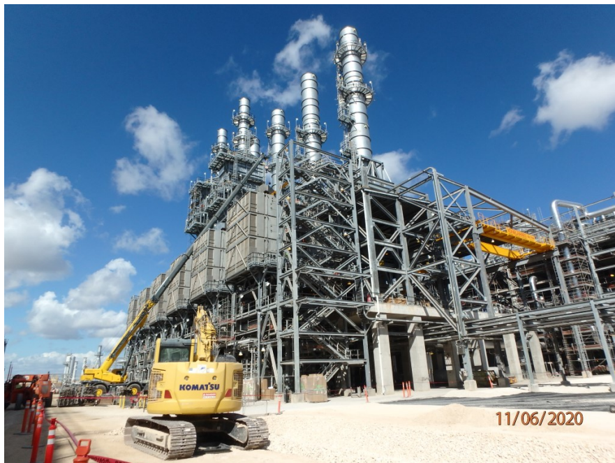
Train 3 - final grading progress
