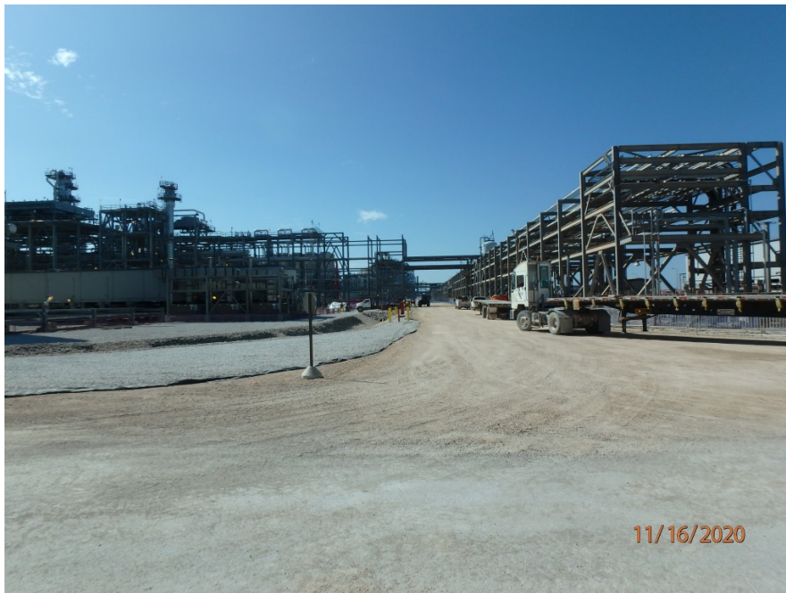
Train 3 - perimeter north road grading prepare for asphalt
