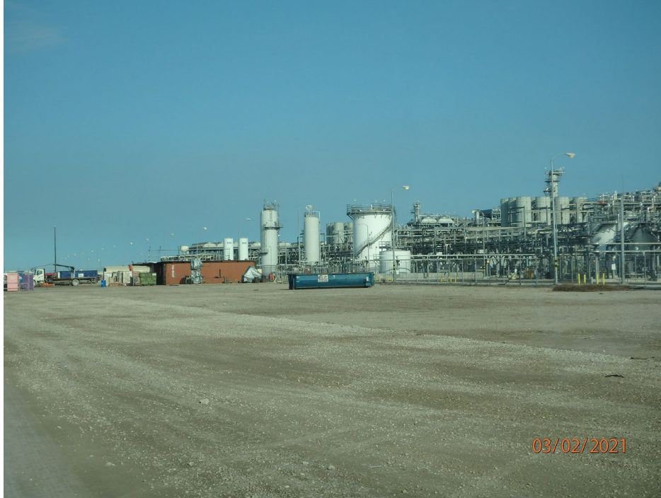
Demobilize 200 ft strip area in progress
