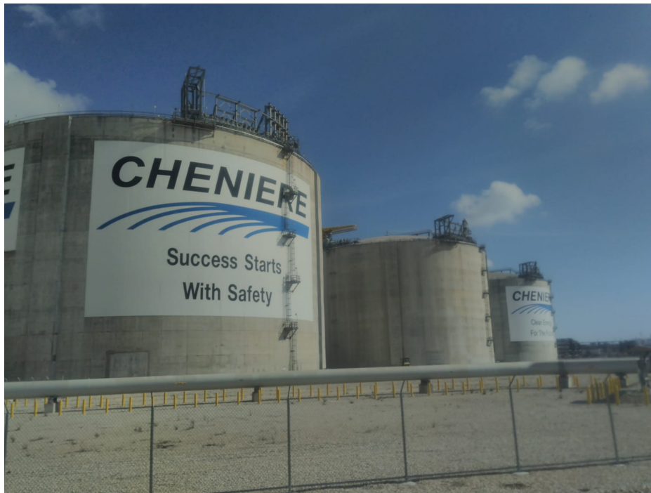
Permanent fence installation at LNG Tank area
