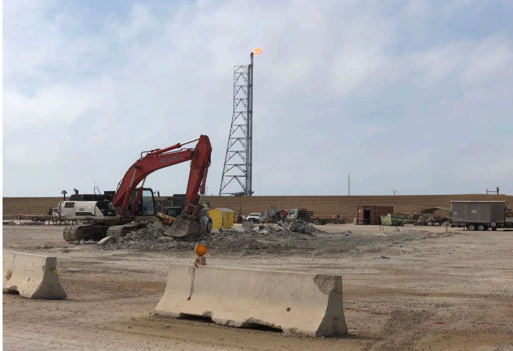
Demobilized and remove concrete slab at South Mechanic shop
