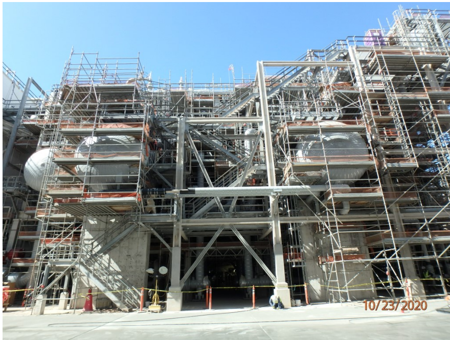
Propane refrigeration area progress overview
