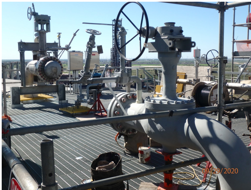
LNG Tank B - fifth pump tie-in piping installation complete
