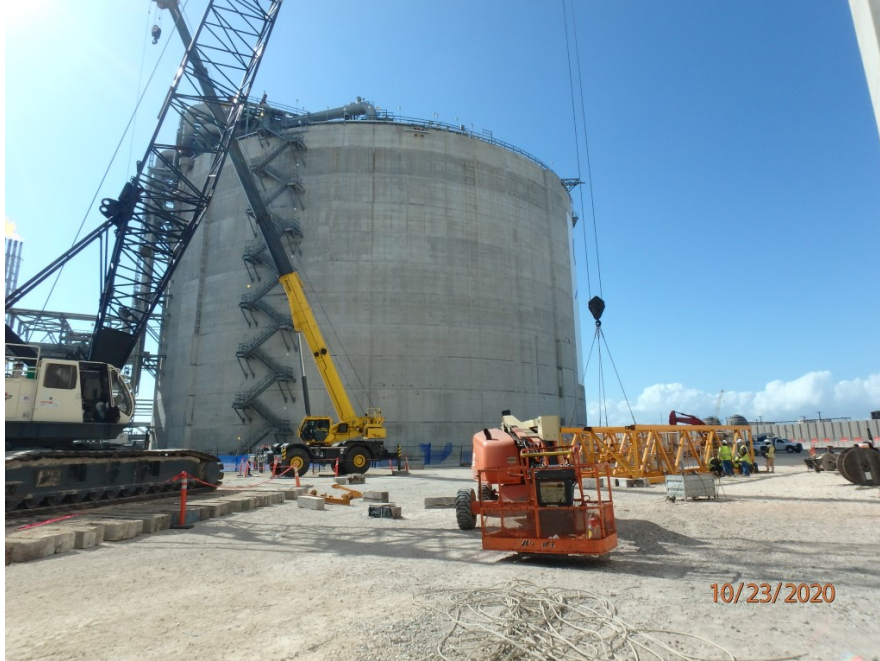
Removal of tower crane at LNG Tank B
