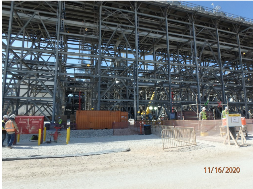
Train 3 - entrance into train 3 after introduction of refrigerants
