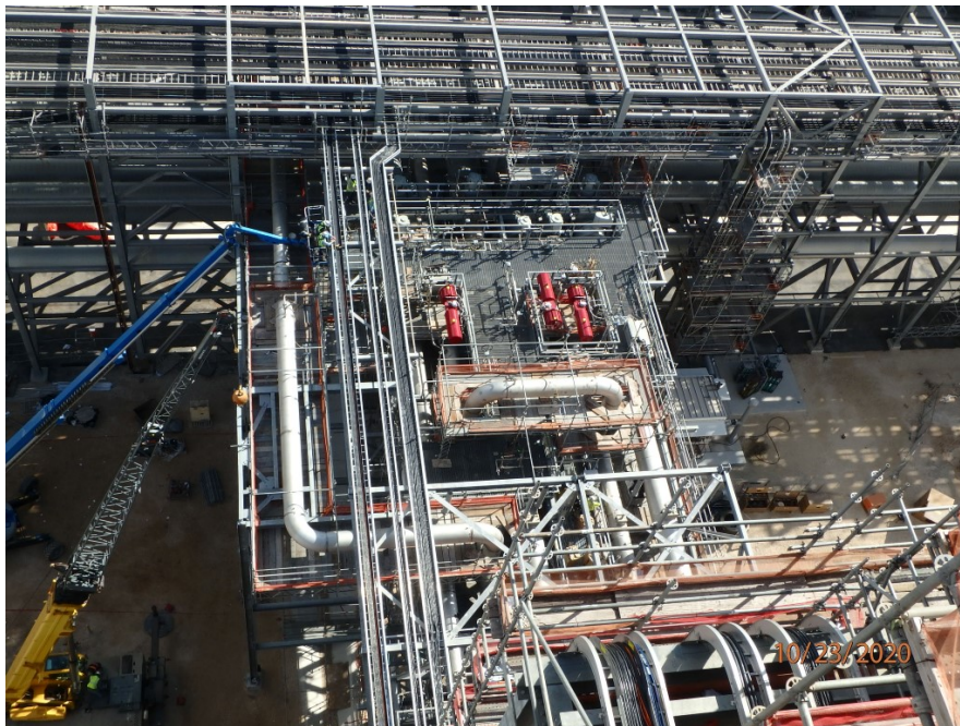
OSBL finger rack platform and jump over scope complete
