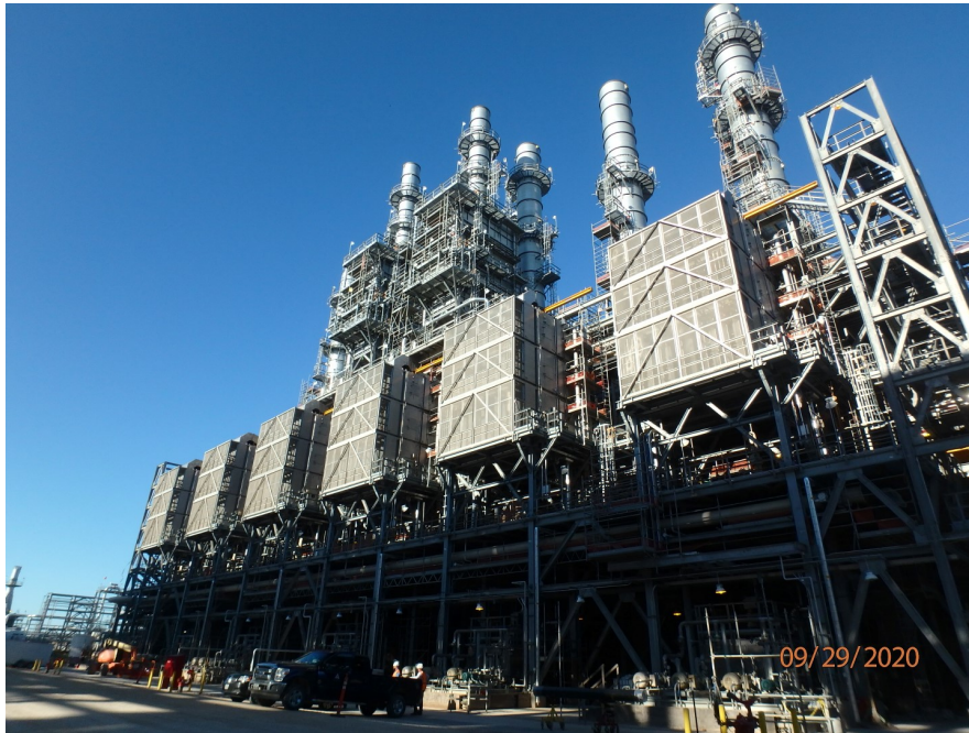
Refrigeration compressor area progress overview
