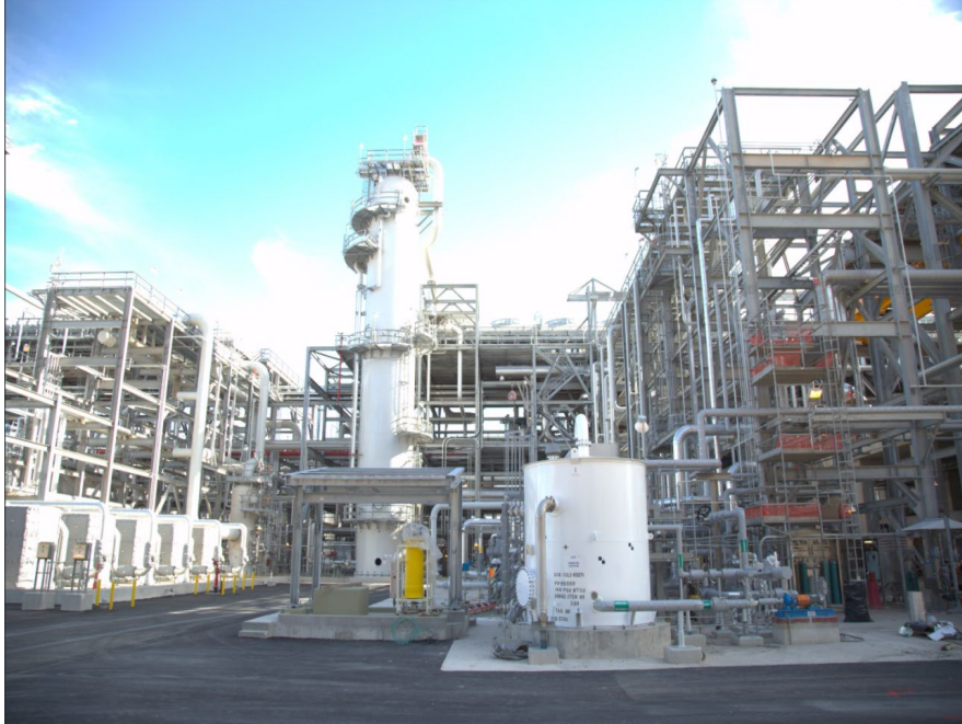
Train 3 - RO sump caustic skid foundation and shelter complete
