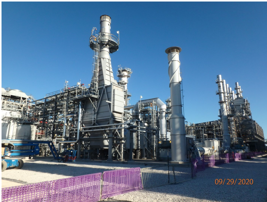
Thermal oxidizer area progress overview
