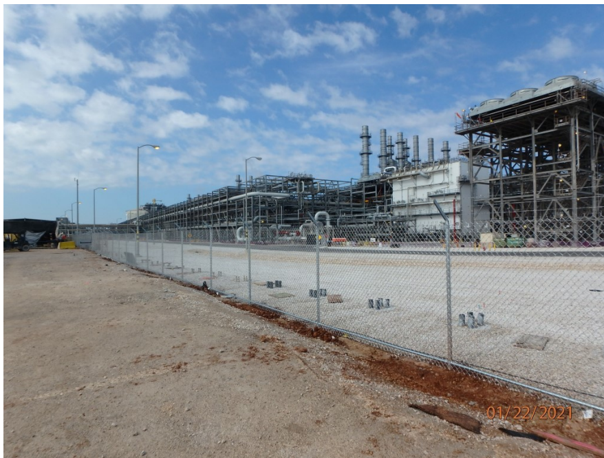
Permanent fence installation in progress
