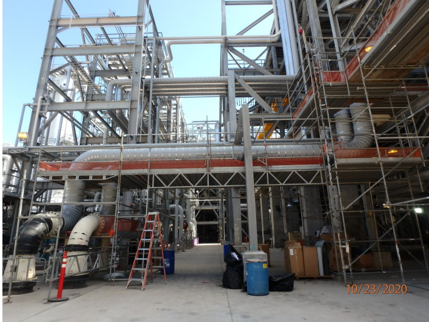
Inlet air chilling system piping insulation in progress
