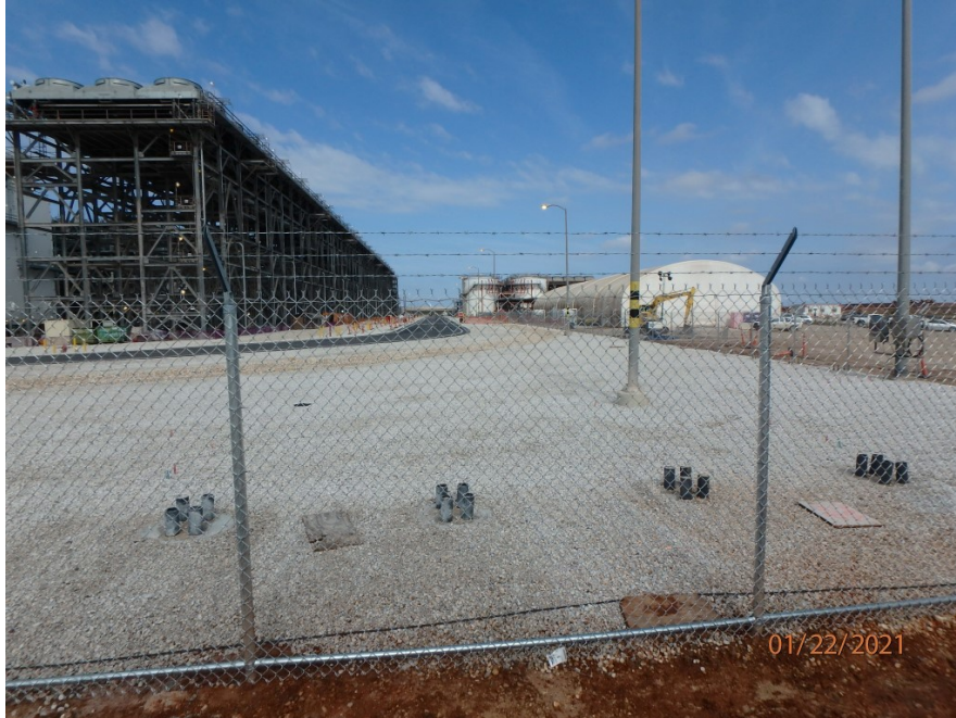
Permanent fence installation south of Train 3
