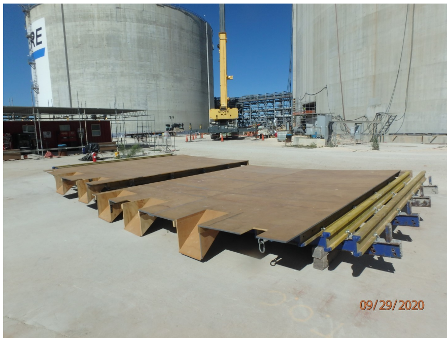
LNG Tank B - formwork for wall closure
