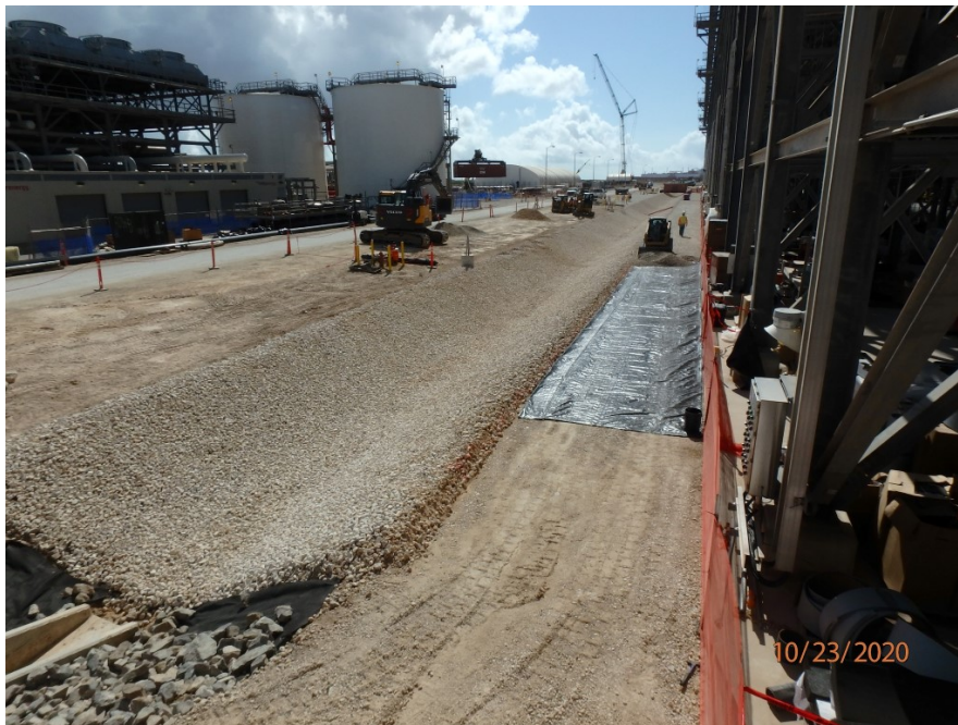
Final grade work in progress
