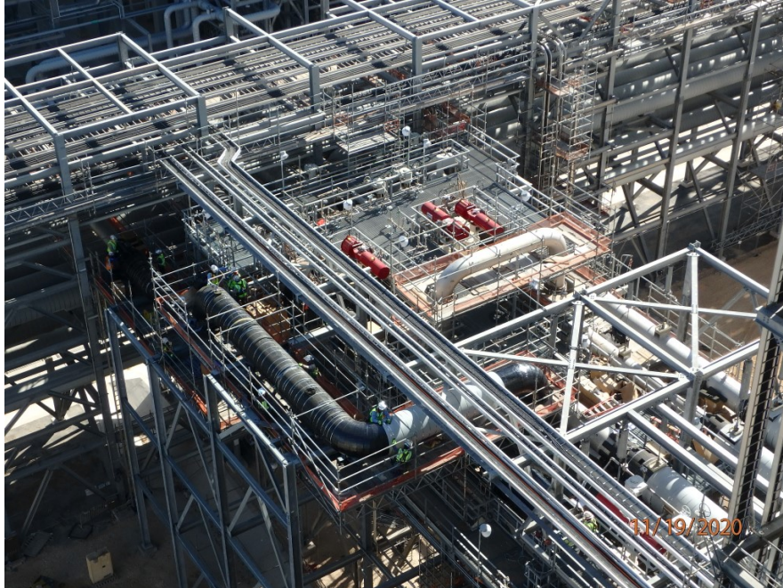
OSBL pipe rack - piping insulation in progress
