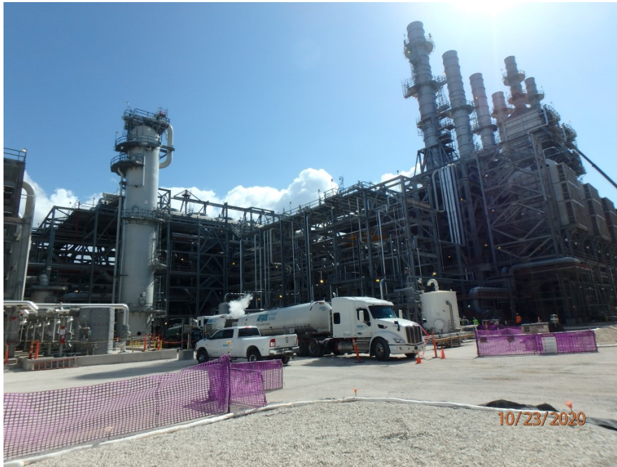
High pressure leak checks feed gas circuit in progress
