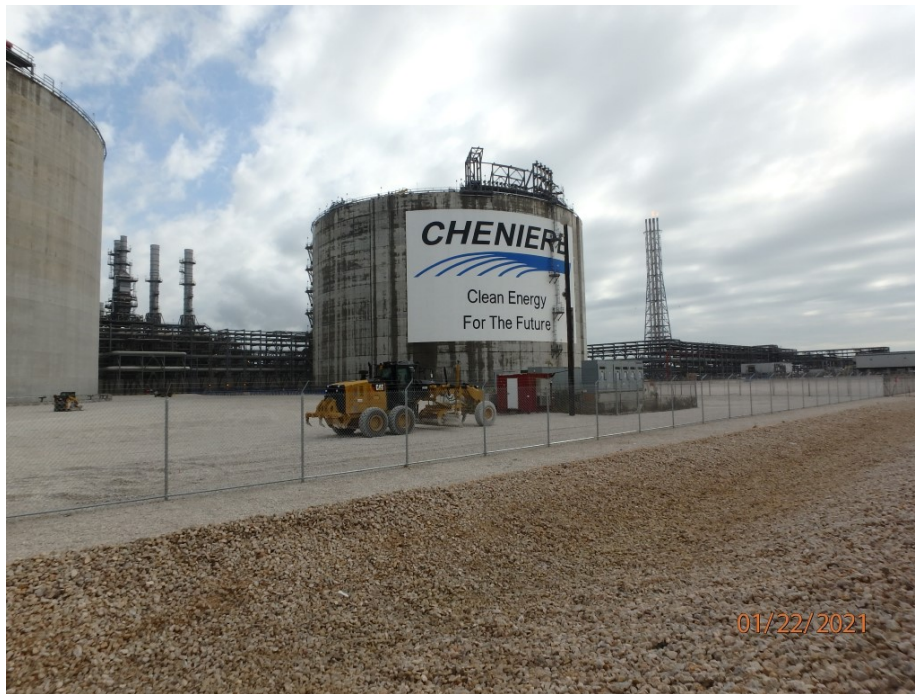
Removing temporary facility from LNG Tank B area
