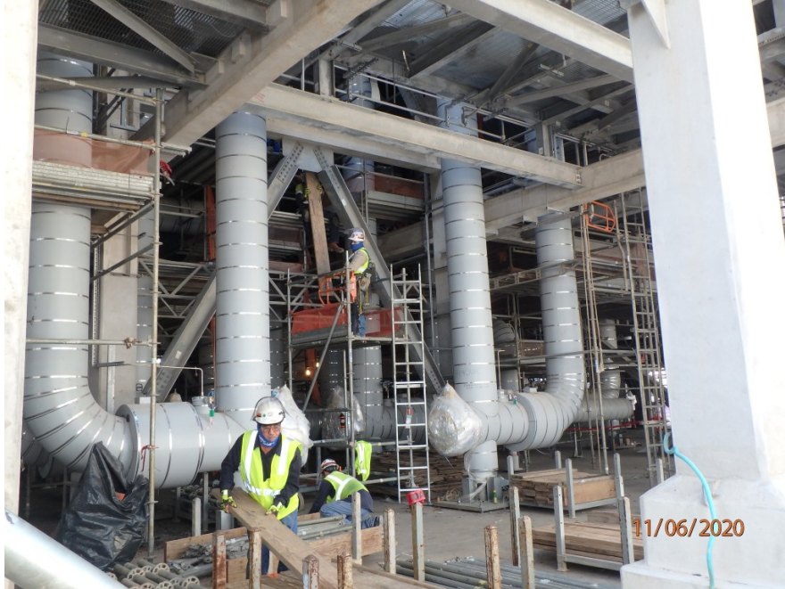
Train 3 - scaffold dismantled
