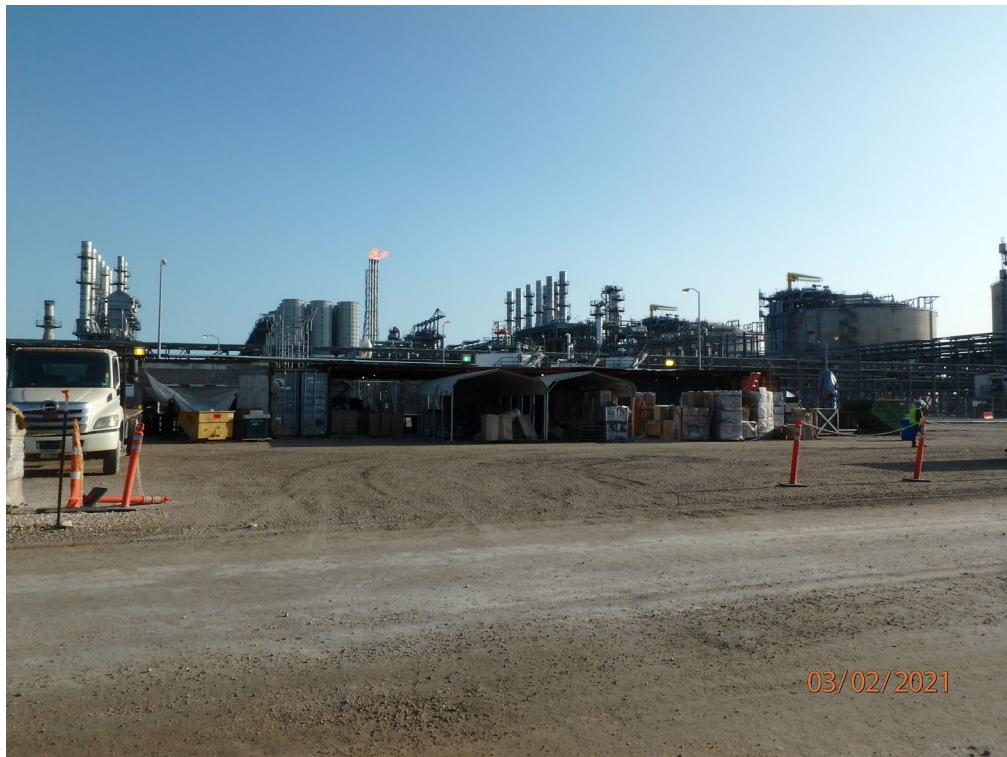
Demobilize insulation fabrication area in progress
