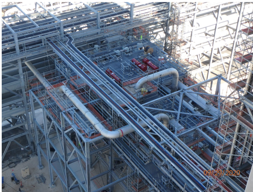
OSBL finger rack - jumbover and rundown piping installation complete
