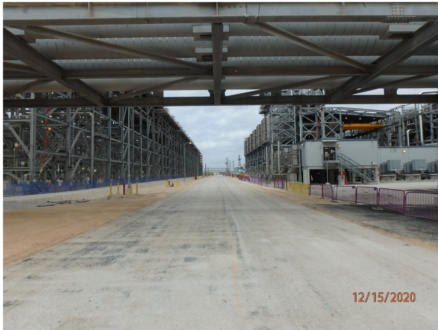
Final grading on Crockett road west of Train 3
