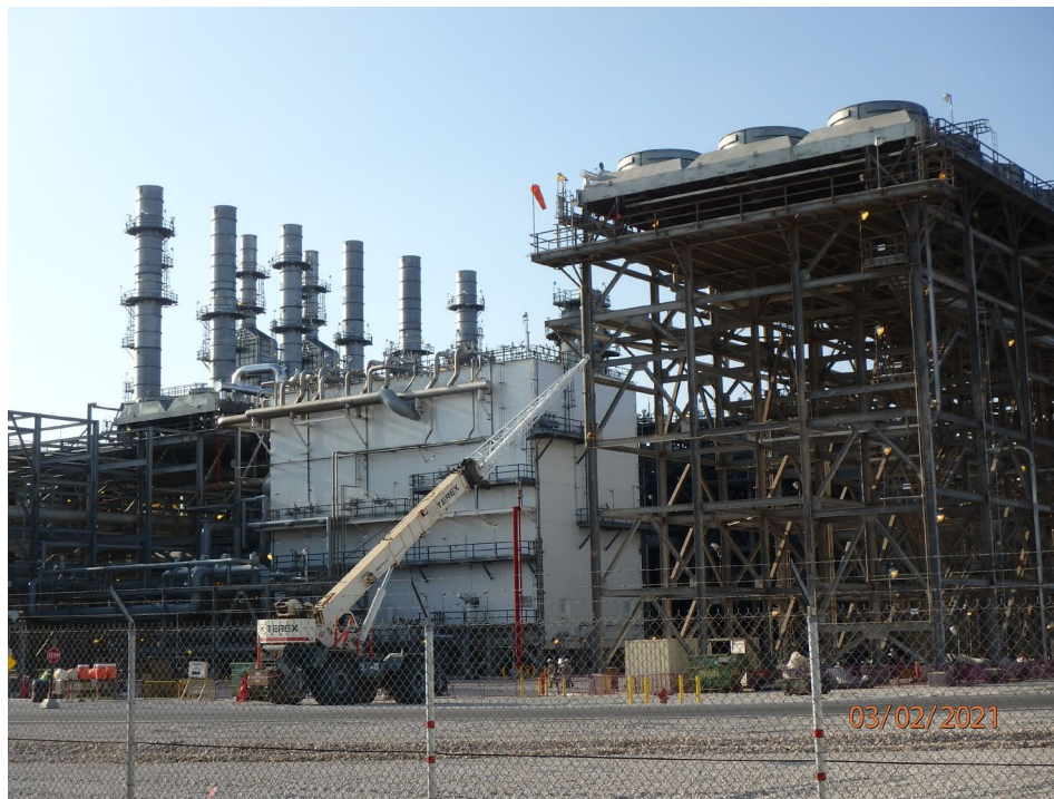
Removal of temporary facility in Train 3
