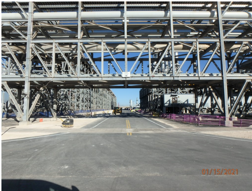
Road asphalt paving and striping west of Train 3
