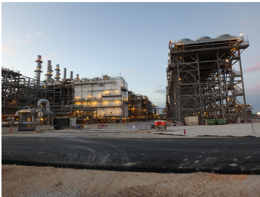
Asphalt paving on Fanin road south of Train 3
