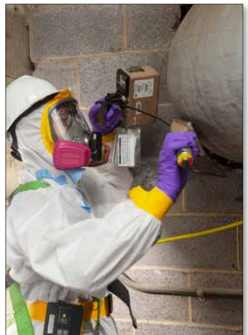
A worker conducts deactivation activities at Y-12's Alpha-2 Building in January 2021.
