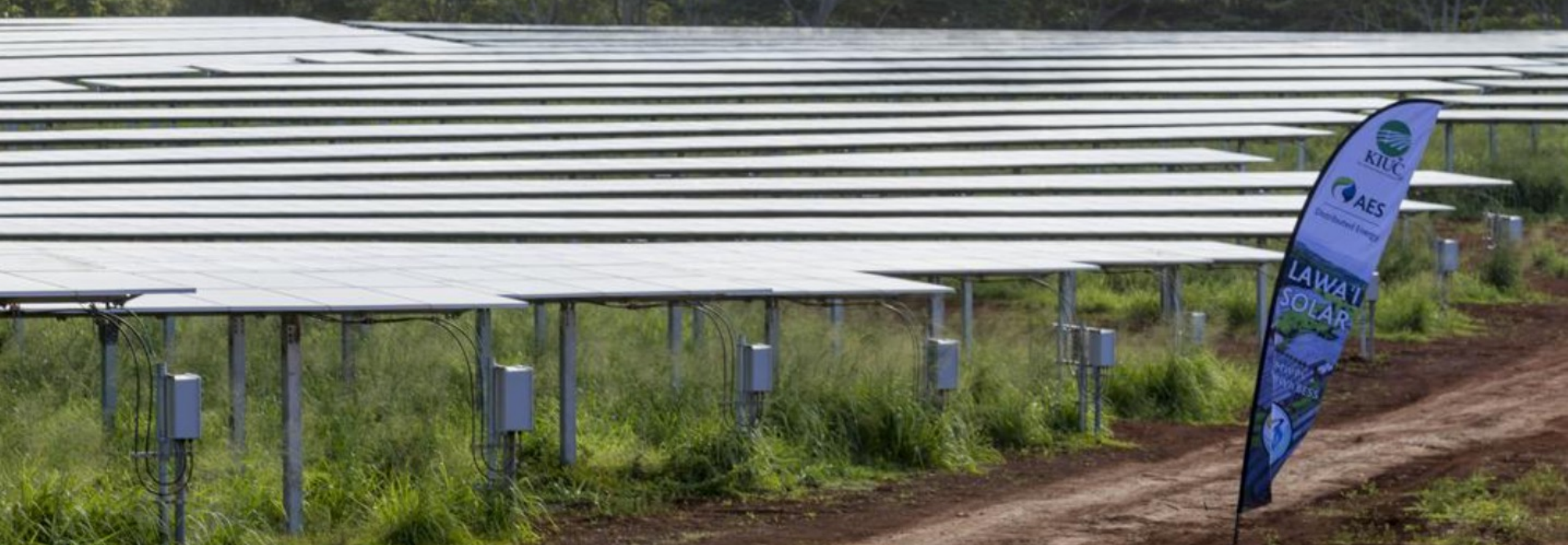
U.S. Navy Naval Facilities Engineering Command's 19.3-megawatt solar project and 70-megawatt-hours battery energy storage system shares power with the Kauai Island Utility Cooperative
