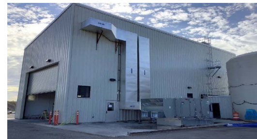
The New DARHT Accelerated Weather Enclosure completed in June 2020
