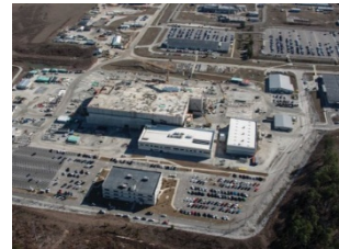
Plans are underway to repurpose the MOX project at the Savannah River Site
