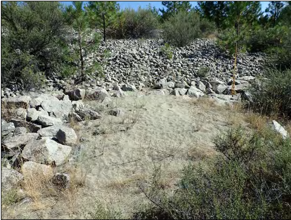
PL-9. Sand Deposit at Toe of Containment Dam Outslope
