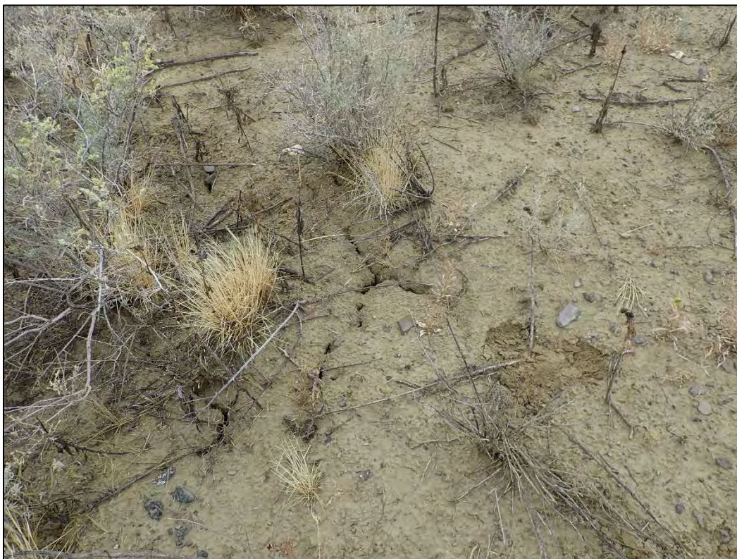
PL-9. Desiccation Crack on Disposal Cell Top Slope
