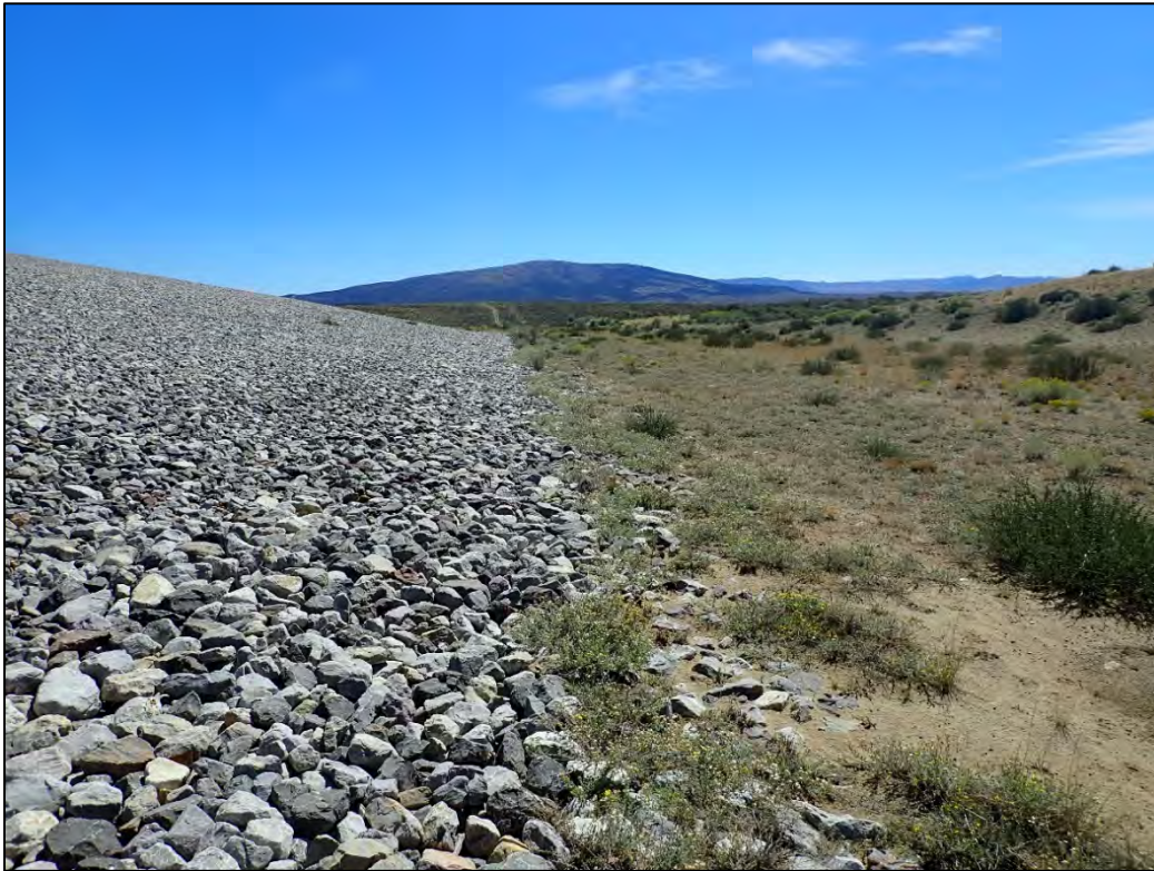
PL-13. Windblown Sediment Accumulating at Toe of Disposal Cell West Side Slope
