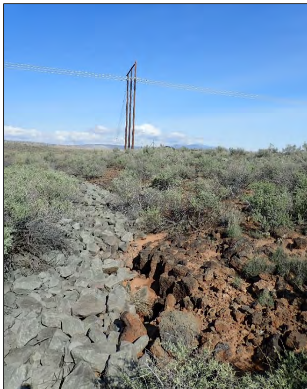
PL-18. Settlement in Fill Covering Basalt at the Interface of the East Dump Cover
