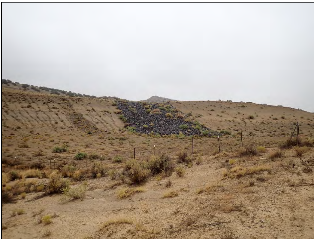
PL-18. Armored Side Slope Near South Channel
