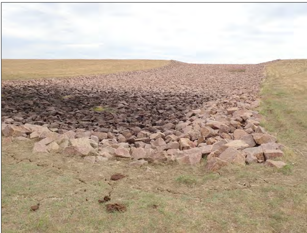
PL-11. South Swale Discharge Point Riprap
