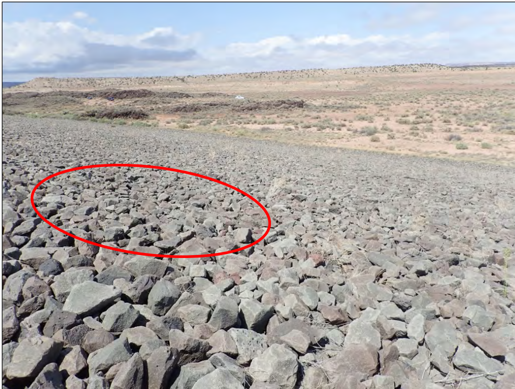
PL-11. Potential Settlement on the North Side Slope of the Main Tailings Disposal Cell
