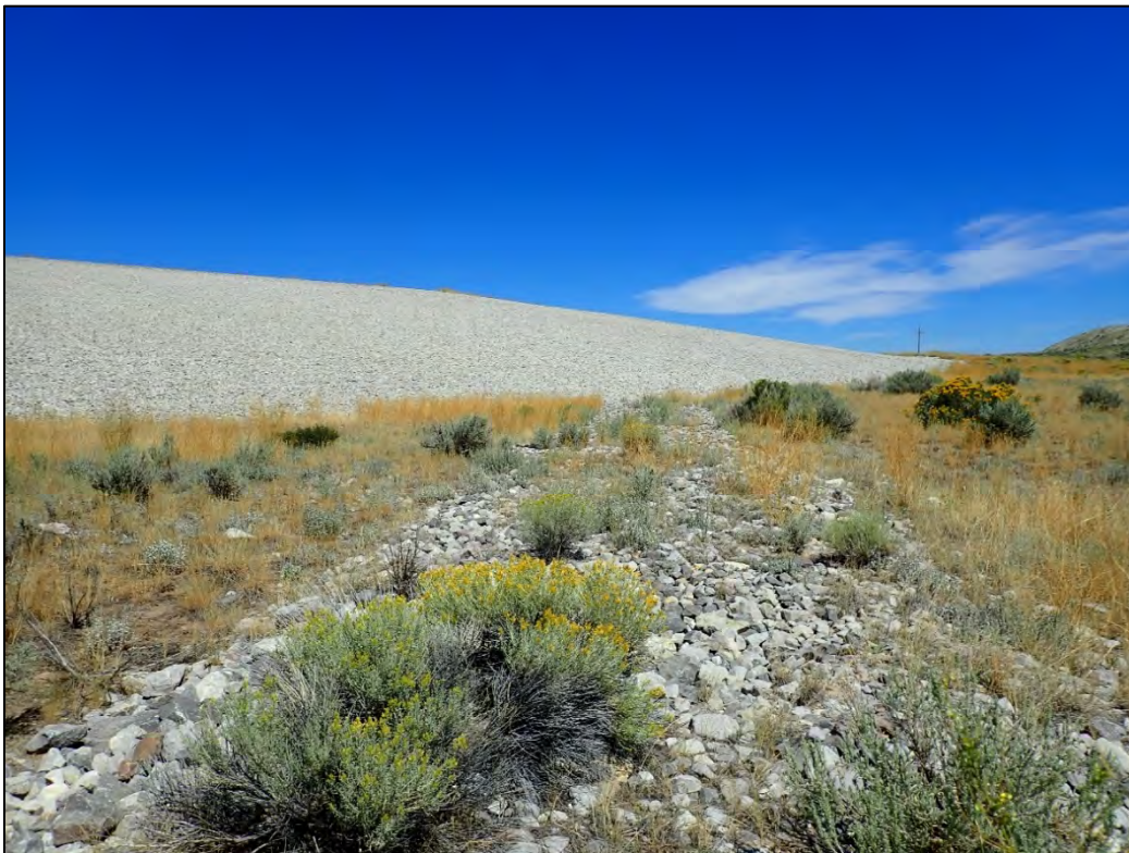
PL-14. Apron Toe Drain North of Ancillary Cell and Disposal Cell South Side Slope in Background
