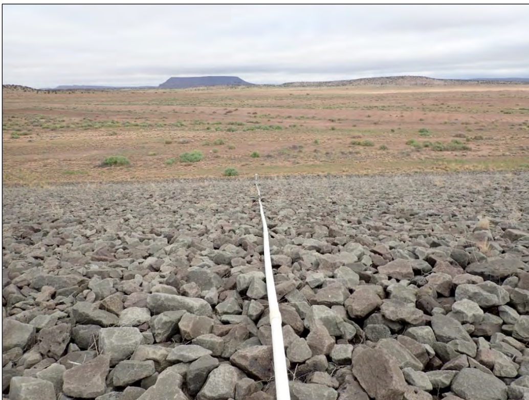
PL-10. Siphon on North Side Slope of the Main Tailings Disposal Cell
