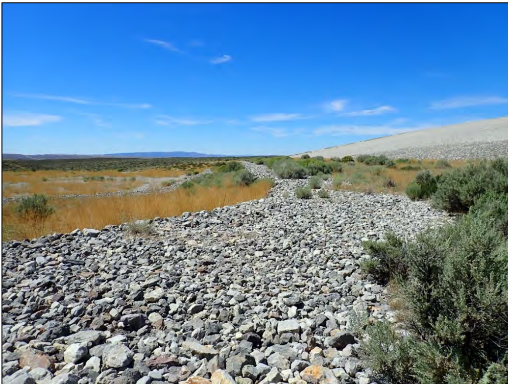
PL-20. Rock Berm North of Ancillary Cell
