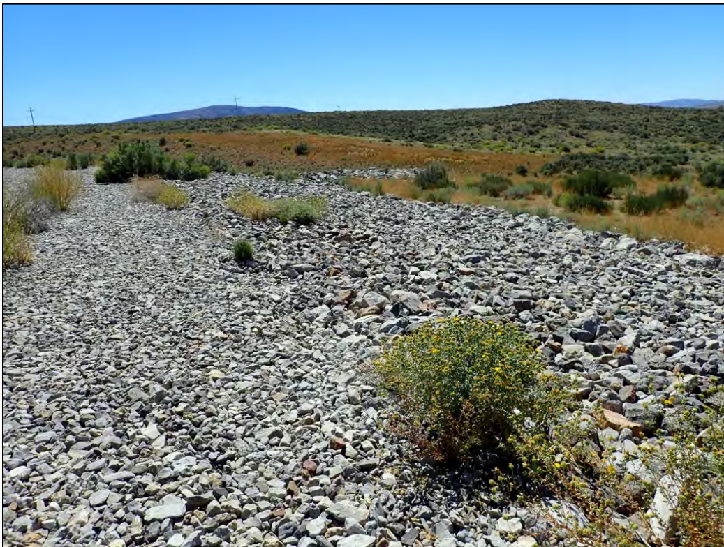
PL-16. Ancillary Cell West Side Slope with Small Depression on Cell Top Slope in Foreground
