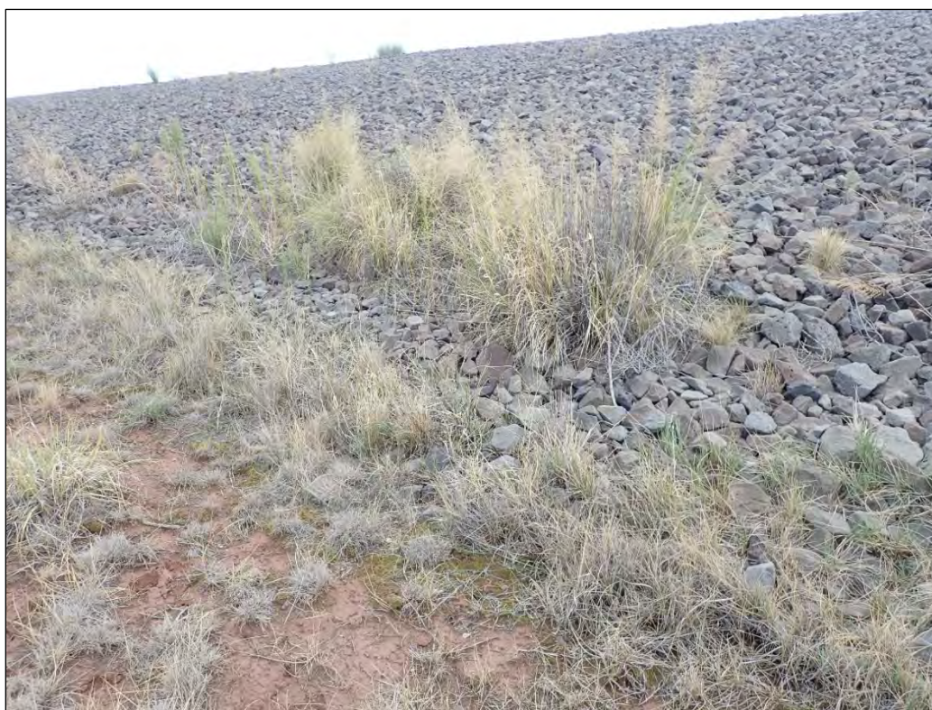
PL-14. Wet Area Near North Toe Slope of the Carbonate Tailings Disposal Cell
