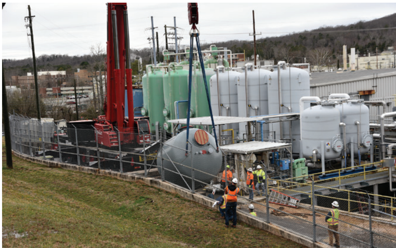
Zeolite tank installation
