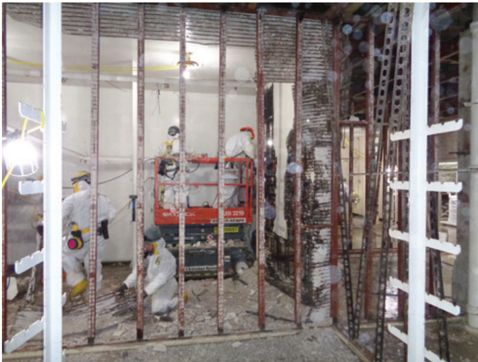
Asbestos removal in the Biology Complex
