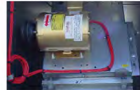
Exclusive AAON® slide out blower assembly provides easy access and service loop.
