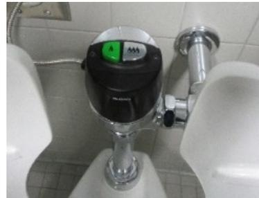
Figure 15. Dual flush system
