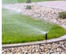
Figure 47. Spray-type sprinkler
