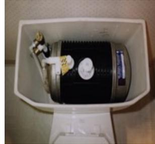
Figure 6. Pressure-assisted tank toilet
