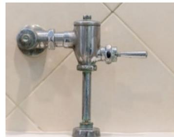
Figure 8. Piston flush valve
