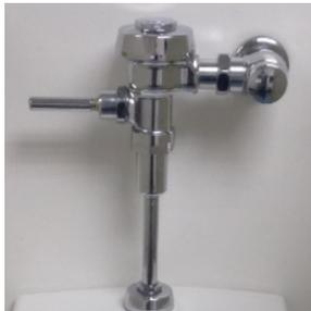
Figure 14. Manual flush valve
