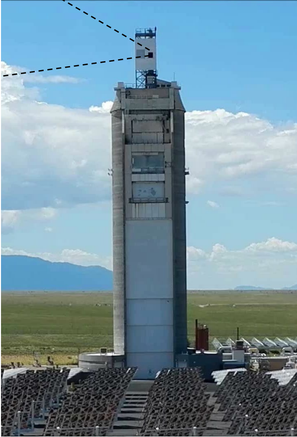
National Solar Thermal Test Facility Sandia National Laboratories
