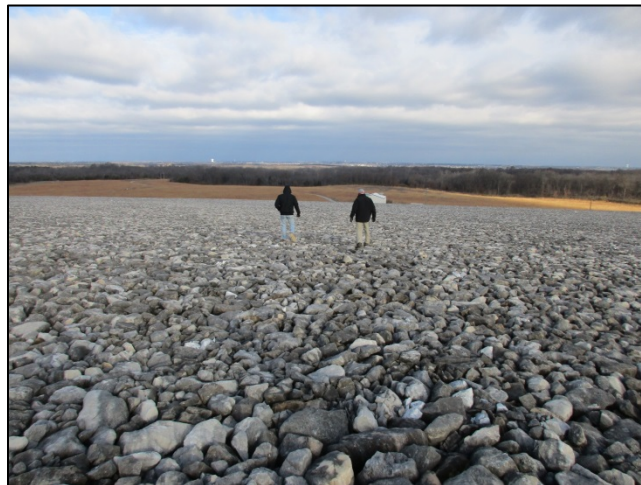
Photo 3: Disposal Cell Inspection
