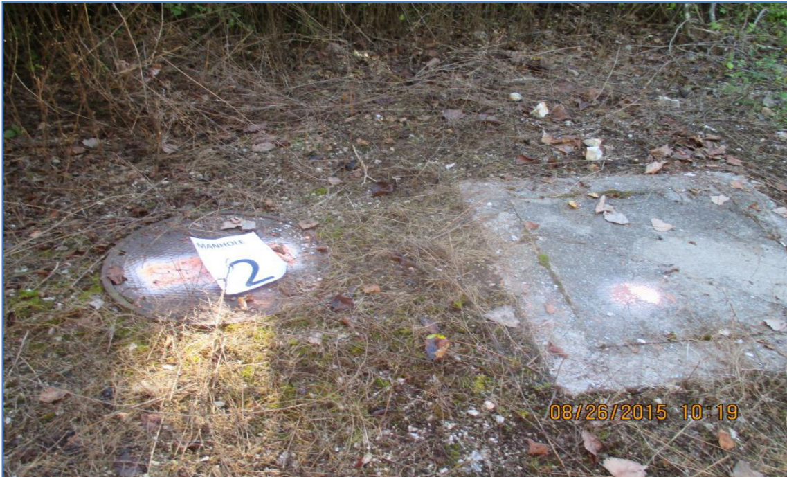
Manhole 2: Near Old Railroad Line
