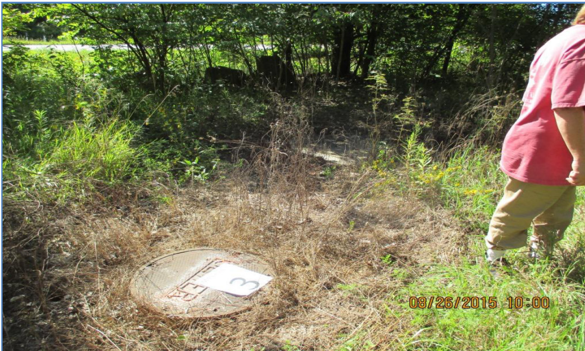
Manhole 3: Near Highway 94
