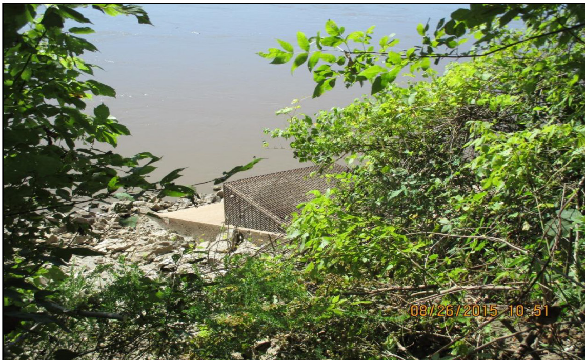
Discharge Outfall Structure at Missouri River
