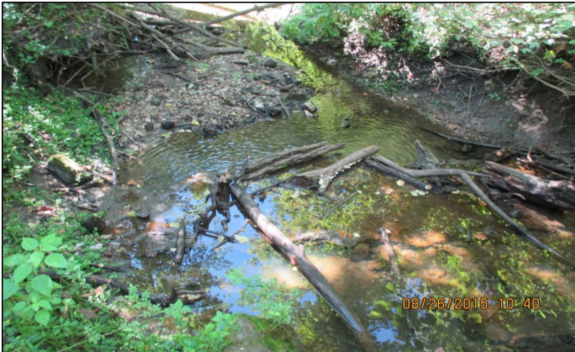
Pipeline crossing under small creek
