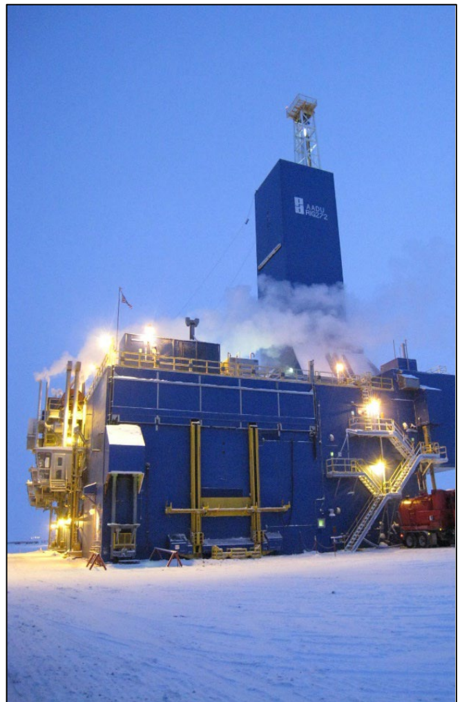
Figure 2: The Parker 272 rig on location at the 7-11-12 site, Prudhoe Bay Unit, December 2018. The well was operated by BP Exploration, (Alaska), Inc. with NETL’s contractor Petrotechnical Resources-Alaska.
