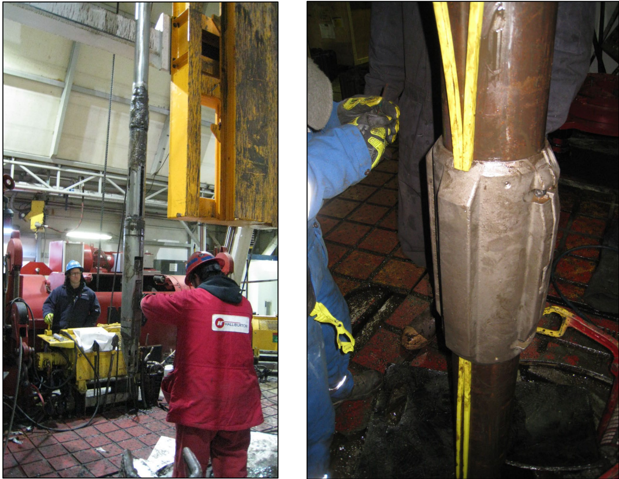
Figure 3: Operations at the Hydrate-01 well included side-wall pressure coring (left) and deployment of twin distributed acoustic sensing/distributed temperature sensing fiber-optic cables as strapped to the well casing during completion (right).
