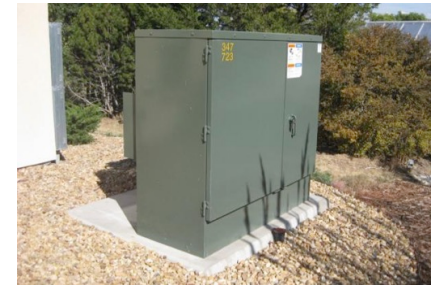
Three-Phase Pad-mount transformer
