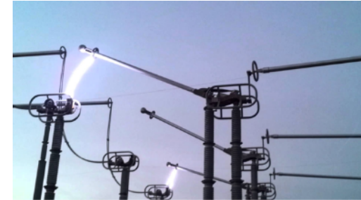
Opening HV Air-break disconnect under load (Not supposed to happen, but still cool!)
