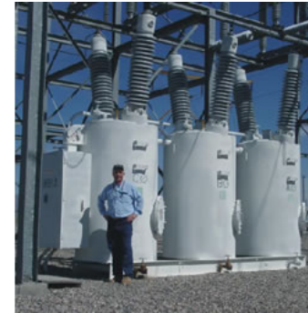
High Voltage Circuit Breakers
