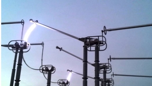
Overhead High-Voltage Disconnect Switches
