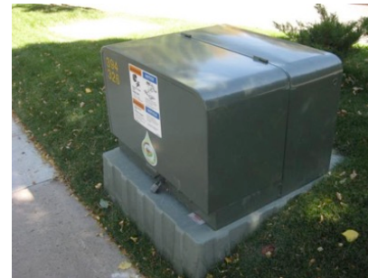
Single-Phase Pad-mount transformer
