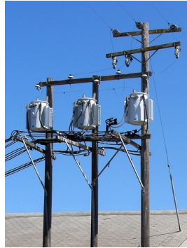
Three-Phase Overhead Transformers
