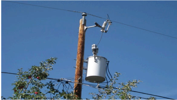
Single-Phase Overhead Transformer
