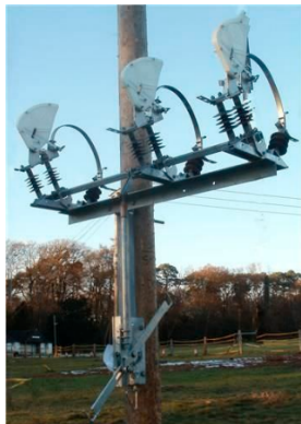
Overhead High-Voltage Disconnect Switches
