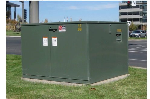
Pad-mount switch cabinet (PMH)
