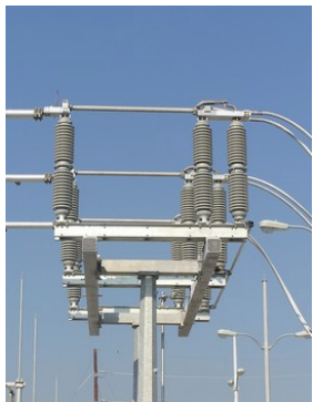
Overhead High-Voltage Disconnect Switches
