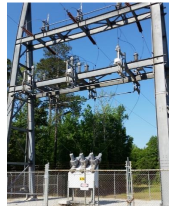
High Voltage Circuit Breakers
