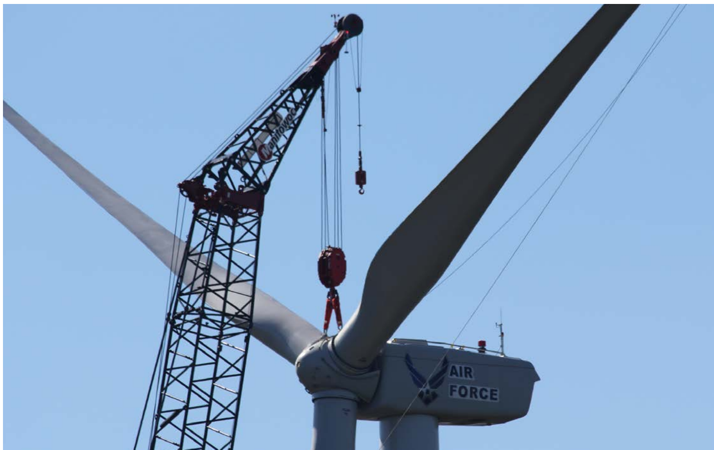
Distributed wind technology, like this turbine stationed at the U.S. Department of Defense's Joint Base Cape Cod in Bourne, Massachusetts, can be adopted by entities such as federal agencies. A new training developed by PNNL, NREL, and FEMP will provide the knowledge needed to make decisions about distributed wind technology investments. Photo by Steve Mellin, Joint Base Cape Cod
