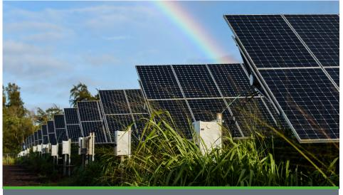
The AES Lawai Solar Project in Hawaii consists of a 28-megawatt solar photovoltaic system with a 100-megawatt-hour battery energy storage system. Photo courtesy of Dennis Schroeder / National Renewable Energy Laboratory.
