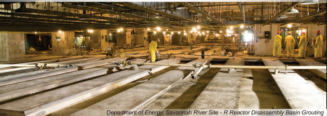
Department of Energy, Savannah River Site - R Reactor Disassembly Basin Grouting
