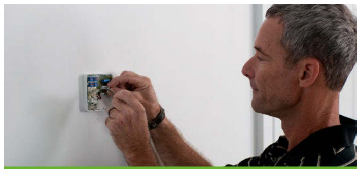
Smart ventilation controls enable more reliable design, installation, and operation to achieve desired indoor air quality. Photo from FSEC
