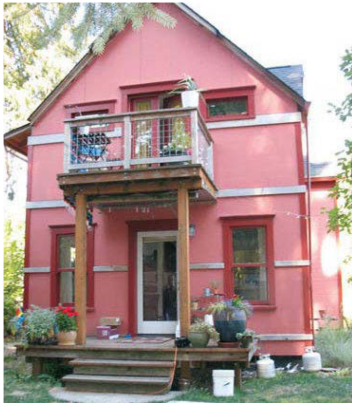
This test home in Olympia, WA, was used to help demonstrate low-cost smart ventilation controls.
