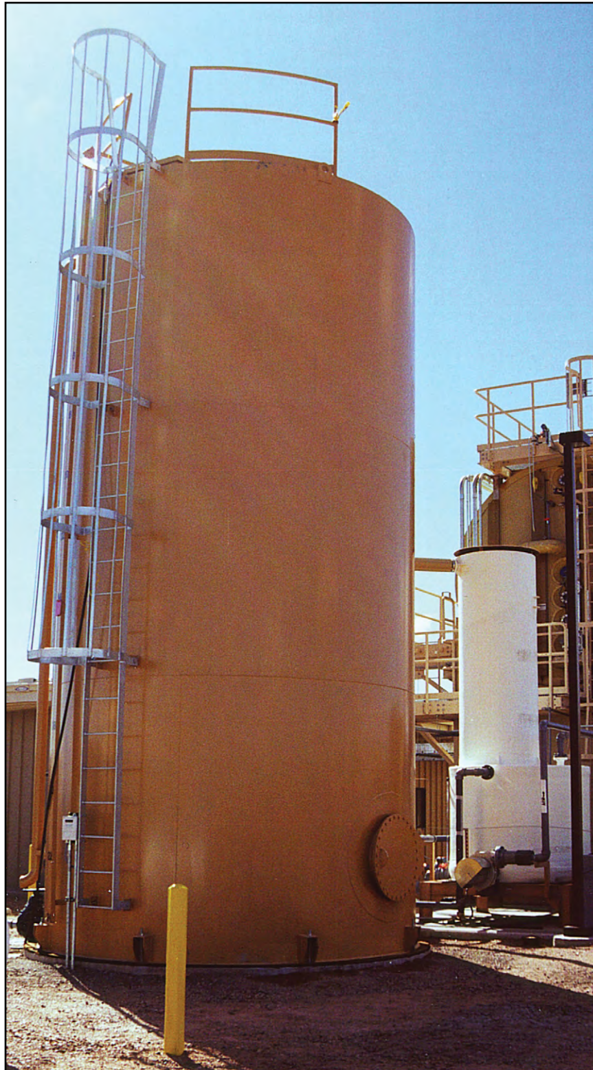
Distillation Unit at the Tuba City, Arizona, Site.
