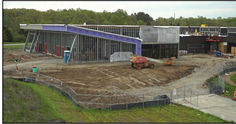
At the Weldon Spring Site in Missouri, U.S. Army Corps of Engineers contractors have completed exterior wall structures and began siding installation on the new interpretive center (spring 2020).
