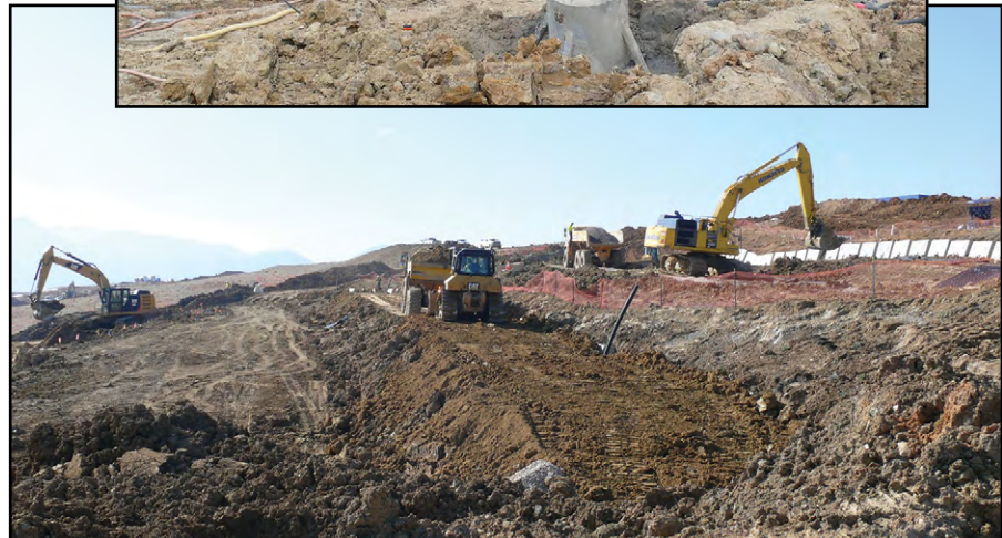
Left: At the Original Landfill stabilization project at the Rocky Flats Site in Colorado, an equipment operator grades soil on top of a drainage ditch below anchor row three on the landfill's east side. A replacement stand pipe, shown in the foreground, was installed to be able to access seep 10 (spring 2020). Top right: LM subcontractors drill into bedrock through the center of a concrete block placed on the landfill's west side, preparing to install a stabilization anchor (spring 2020). Bottom right: Equipment operators on the landfill's east side place gravel in an interceptor ditch below anchor row three and place backfill soil over completed anchor row four (spring 2020).
