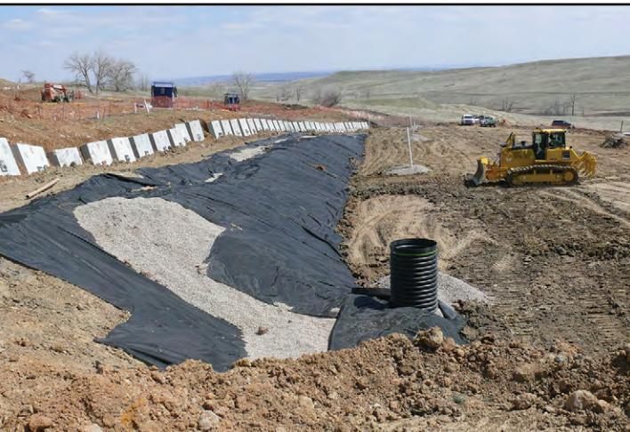
Left: At the Original Landfill stabilization project at the Rocky Flats Site in Colorado, an equipment operator grades soil on top of a drainage ditch below anchor row three on the landfill's east side. A replacement stand pipe, shown in the foreground, was installed to be able to access seep 10 (spring 2020). Top right: LM subcontractors drill into bedrock through the center of a concrete block placed on the landfill's west side, preparing to install a stabilization anchor (spring 2020). Bottom right: Equipment operators on the landfill's east side place gravel in an interceptor ditch below anchor row three and place backfill soil over completed anchor row four (spring 2020).
