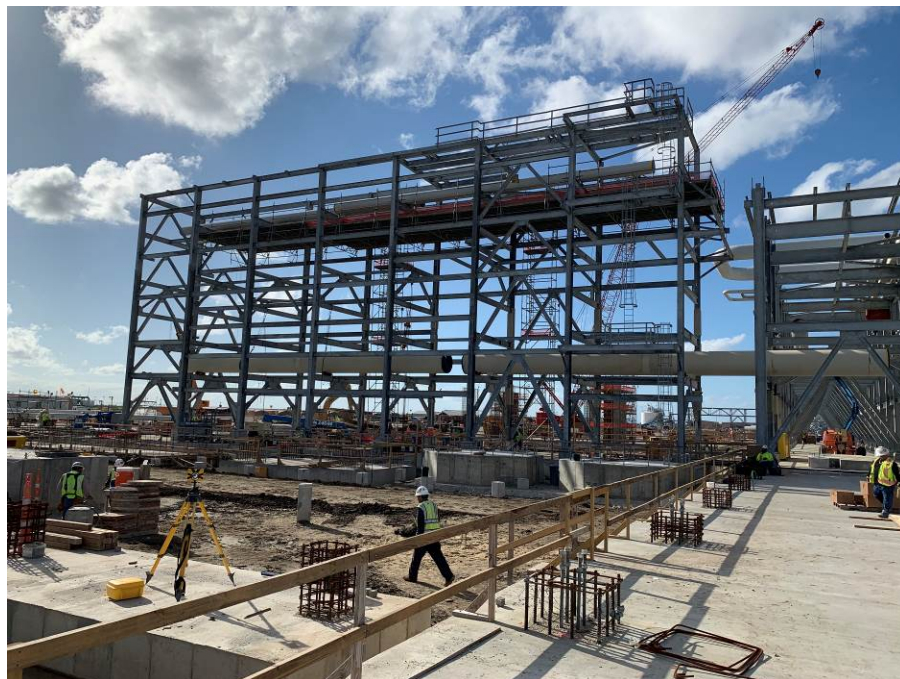
Steel and Pipe Progress at Mercury Dehydration Rack
