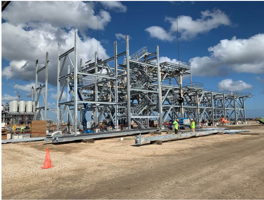
Structural Steel progress at Propane Condenser Rack
