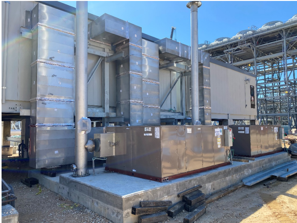
HVAC Ducting at Compressor Substation Area
