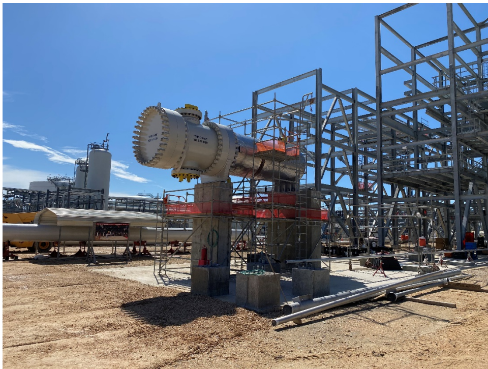
Feed Gas Heater
