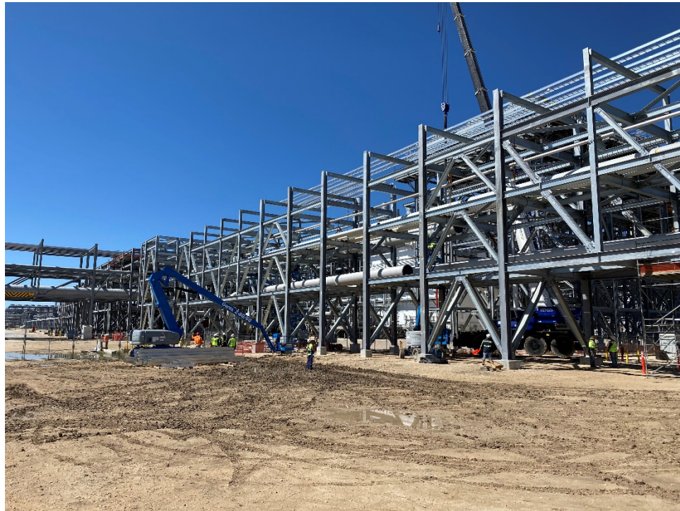
Steel and Pipe Progress at Piperack
