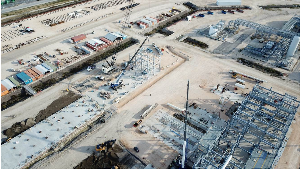
Structural Steel Progress at South End of Train 6
