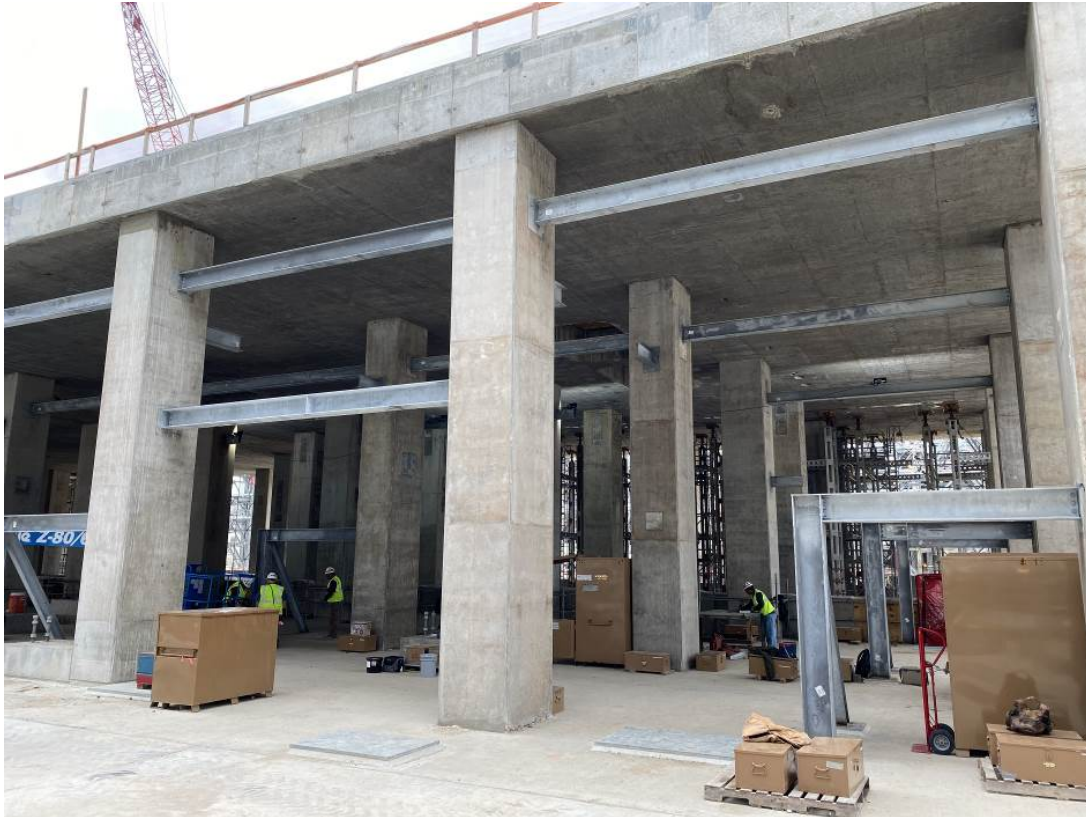
"Under the Tabletop" structural steel in the Compressor Area
