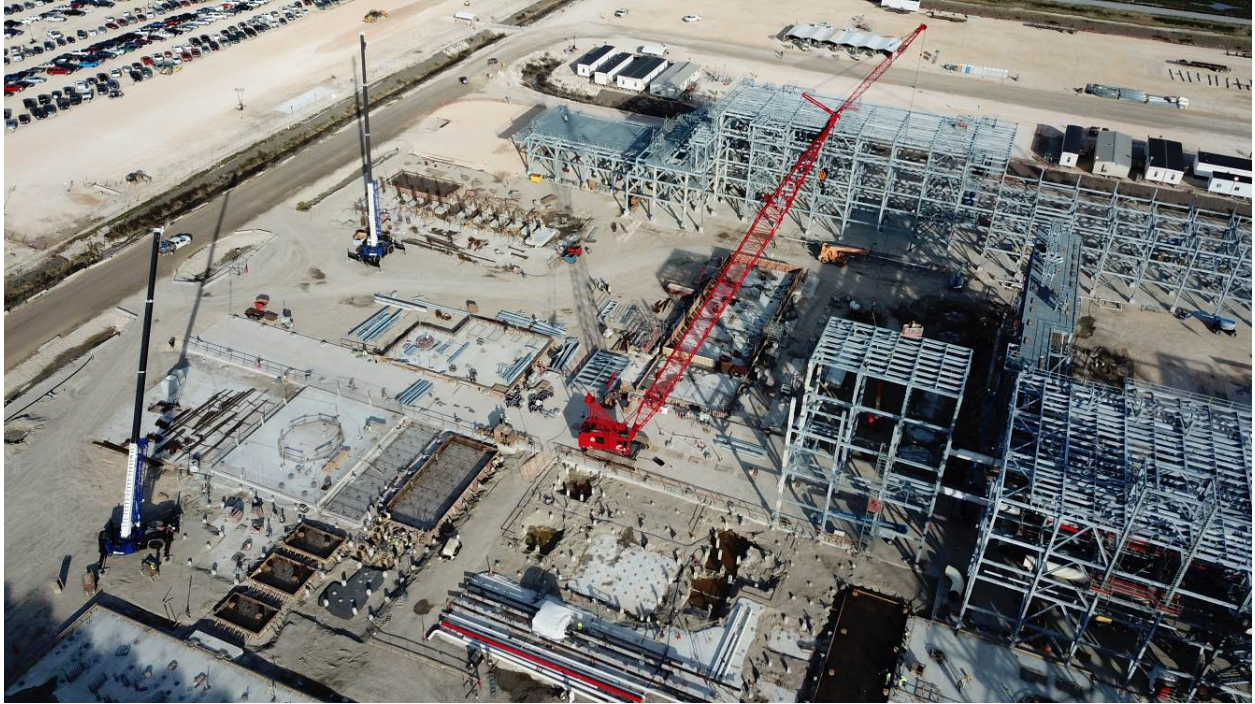
Progress at North End of Train 6
