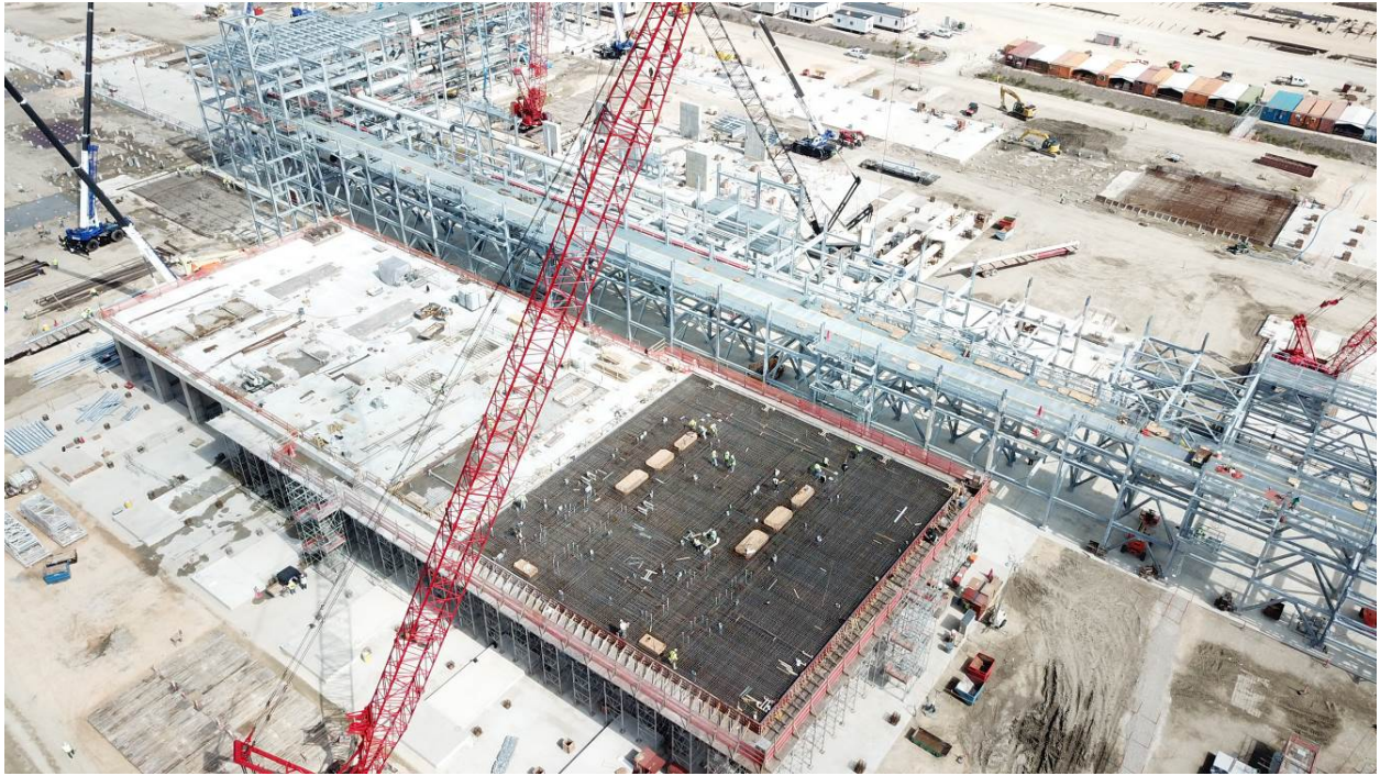
Train 6 Progress facing East
