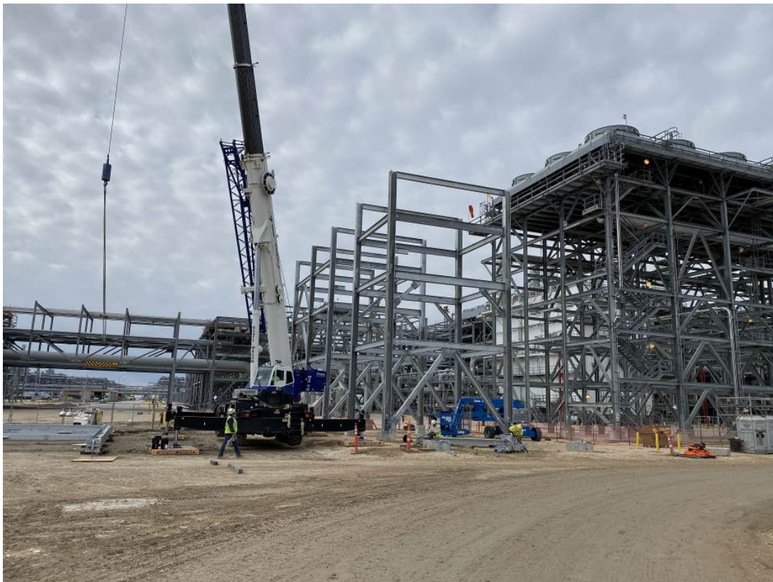
Structural Steel in the E-W Piperack Area
