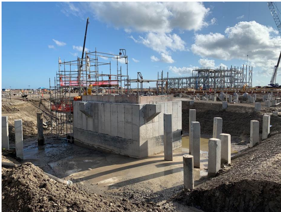
Amine Sump Progress at Amine Regeneration Area
