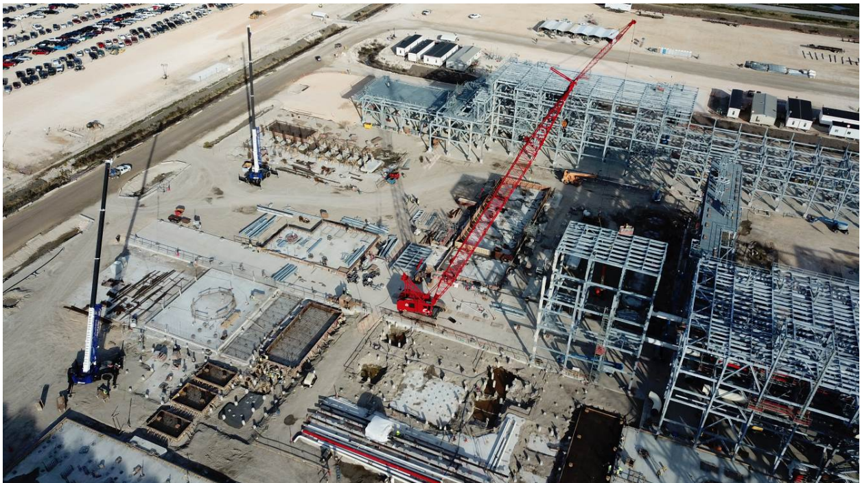
Progress at North End of Train 6
