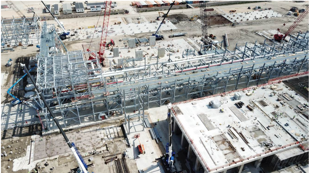
Upper and Lower Structural Steel Progress at Cryo Rack Area 446D01
