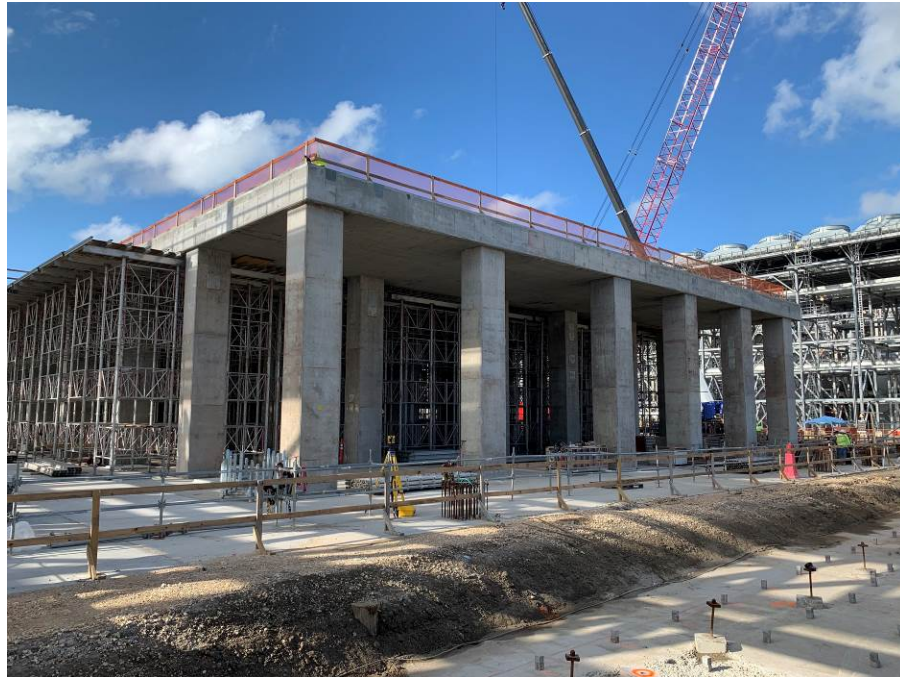
Propane Tabletop at Compressor Area
