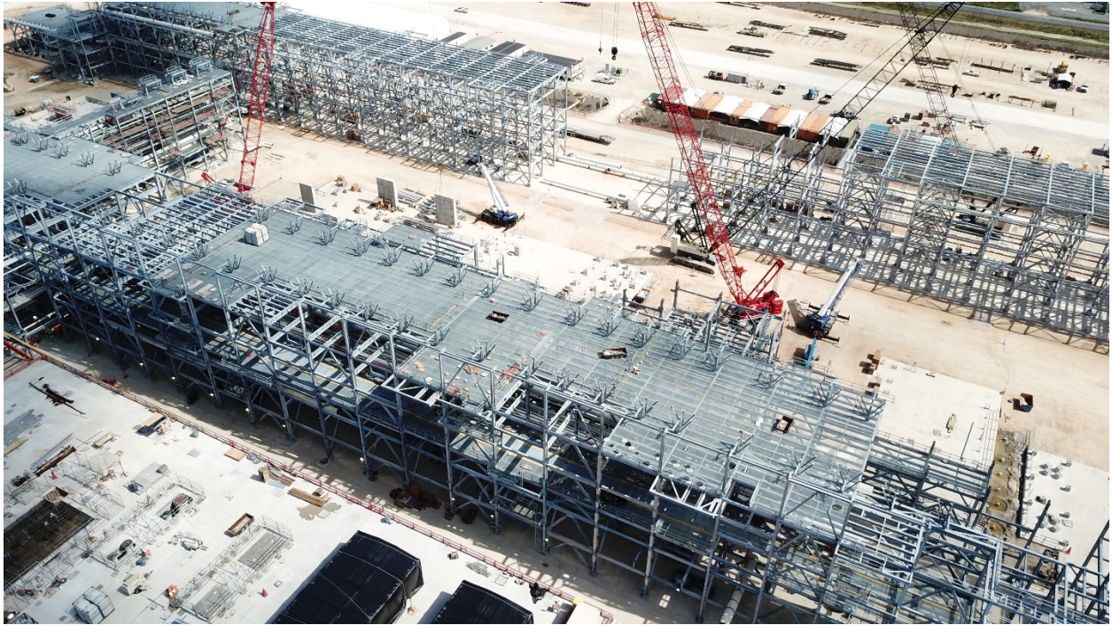
Steel Progress through Train 6
