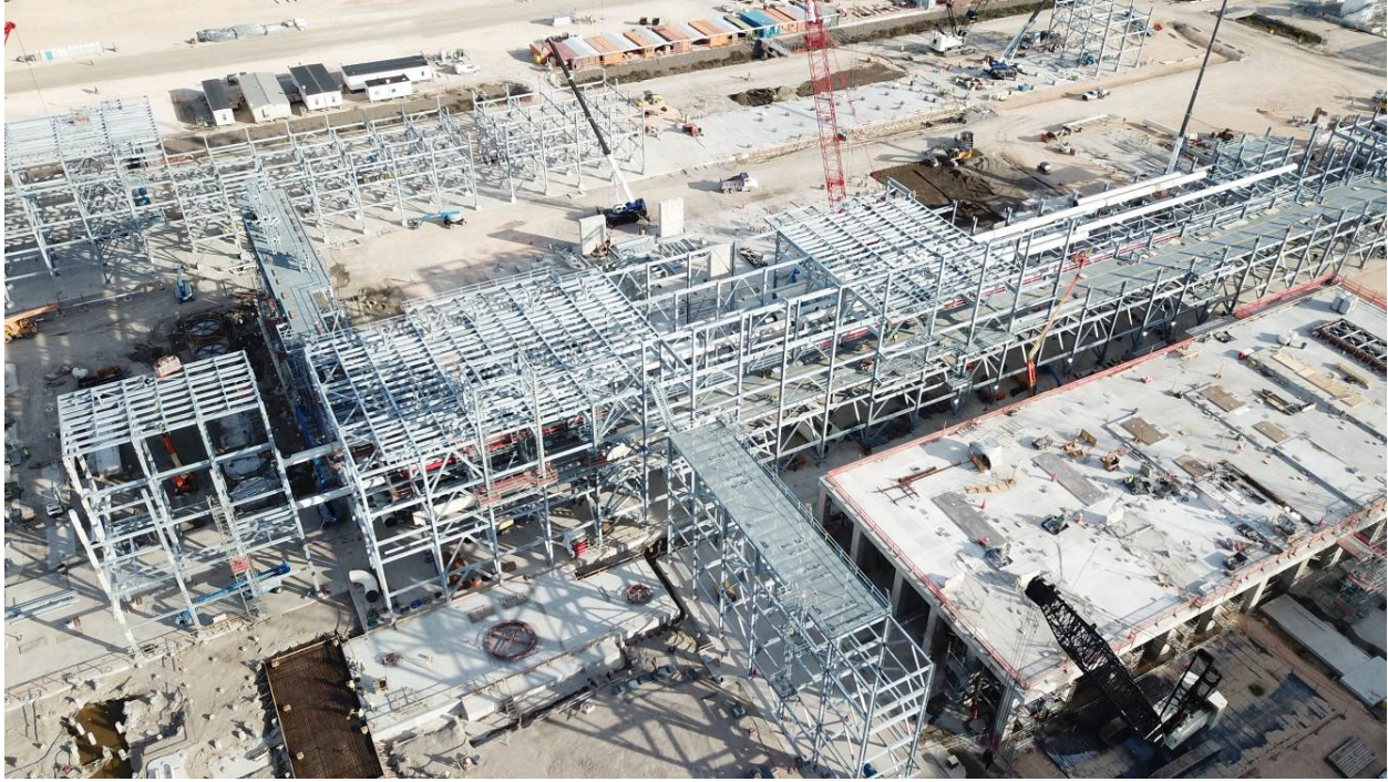
Train 6 Progress facing East
