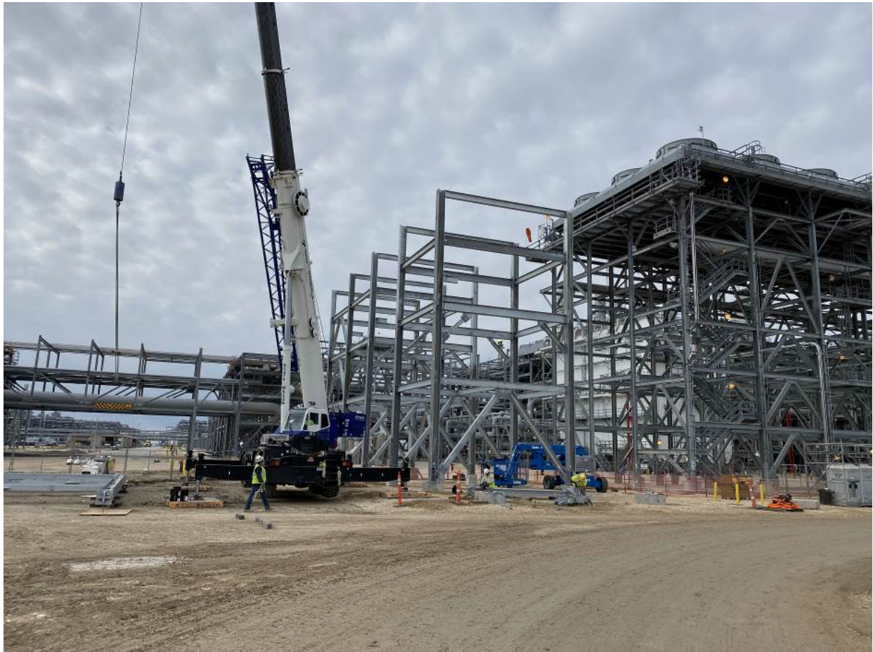
Structural Steel in the E-W Piperack Area
