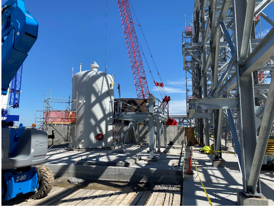
Carbon Treater and Amine Surge Tank
