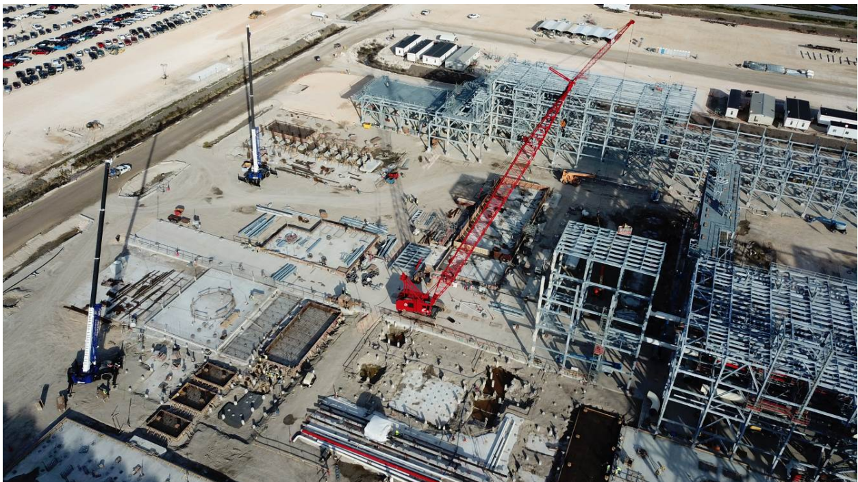
Progress at North End of Train 6
