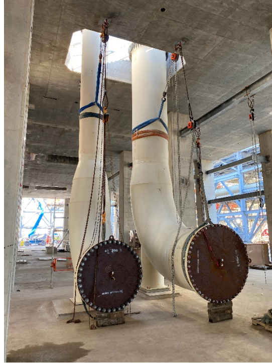
First Hockey-stick pipe in Compressor Area
