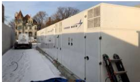
Battery Energy Storage
