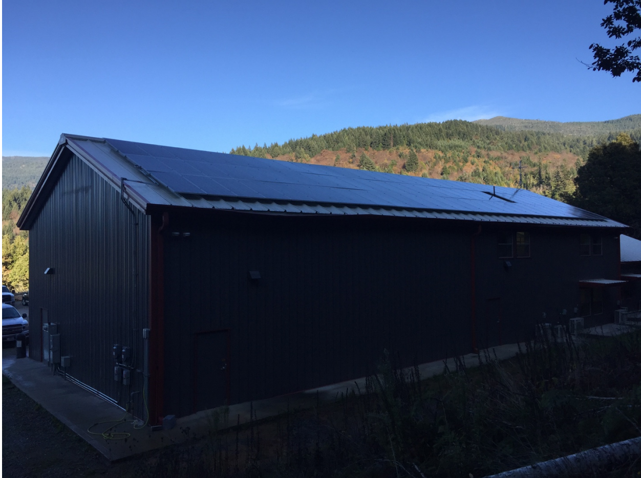
Figure 6: Rooftop PV system on Tulley Creek Transportation Building
