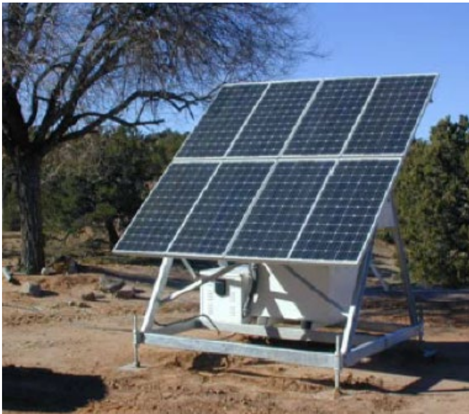
Figure 11: Example of a standardized, palletized PV system. Source: Navajo Tribal Utility Authority
