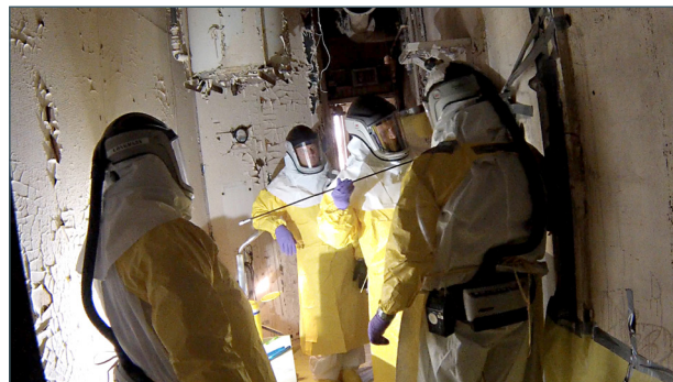
SITE: OAK RIDGE NATIONAL LABORATORY ACTIVITY: BUILDINGS 3028 AND 3029
