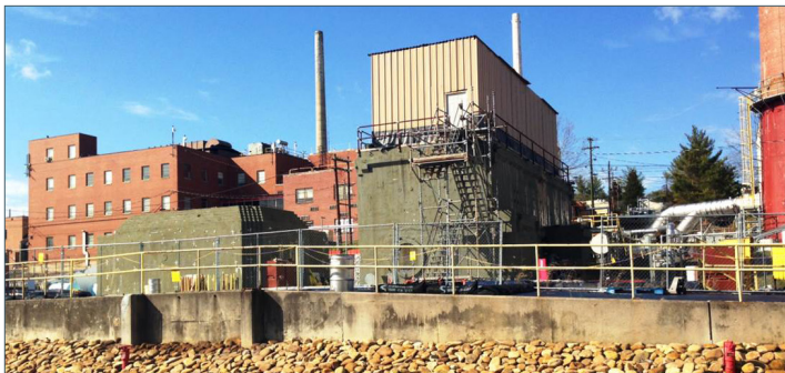
SITE: OAK RIDGE NATIONAL LABORATORY ACTIVITY: BUILDING 3026
