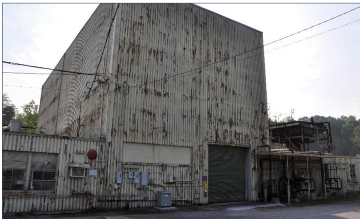
SITE: OAK RIDGE NATIONAL LABORATORY ACTIVITY: BUILDING 7500
