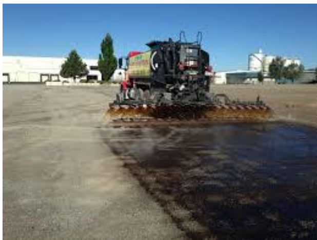
Photo 3. Application of dust palliatives for dust suppression
