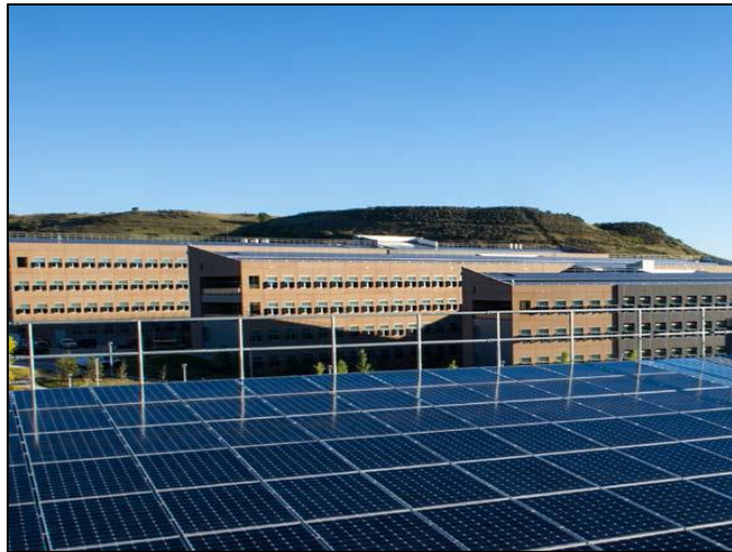
National Renewable Energy Laboratory's Roof Array
