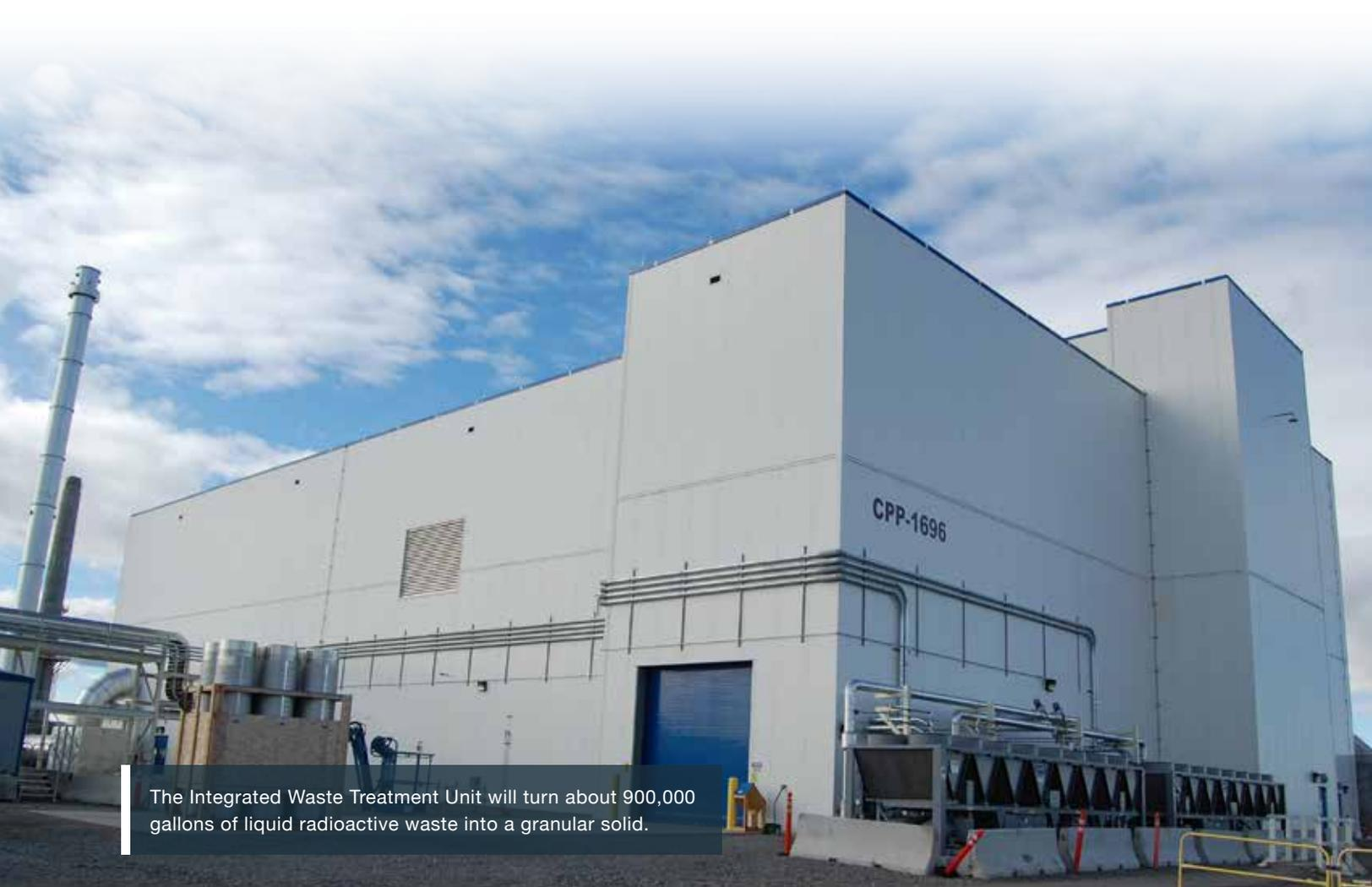
The Integrated Waste Treatment Unit will turn about 900,000 gallons of liquid radioactive waste into a granular solid.
