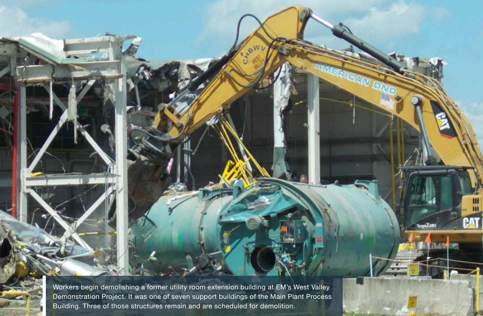
Workers begin demolishing a former utility room extension building at EM's West Valley Demonstration Project. It was one of seven support buildings of the Main Plant Process Building. Three of those structures remain and are scheduled for demolition.
