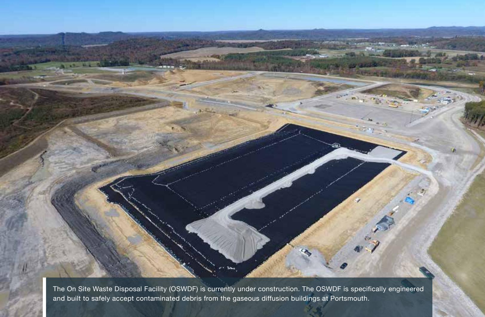
The On Site Waste Disposal Facility (OSWDF) is currently under construction. The OSWDF is specifically engineered and built to safely accept contaminated debris from the gaseous diffusion buildings at Portsmouth.
