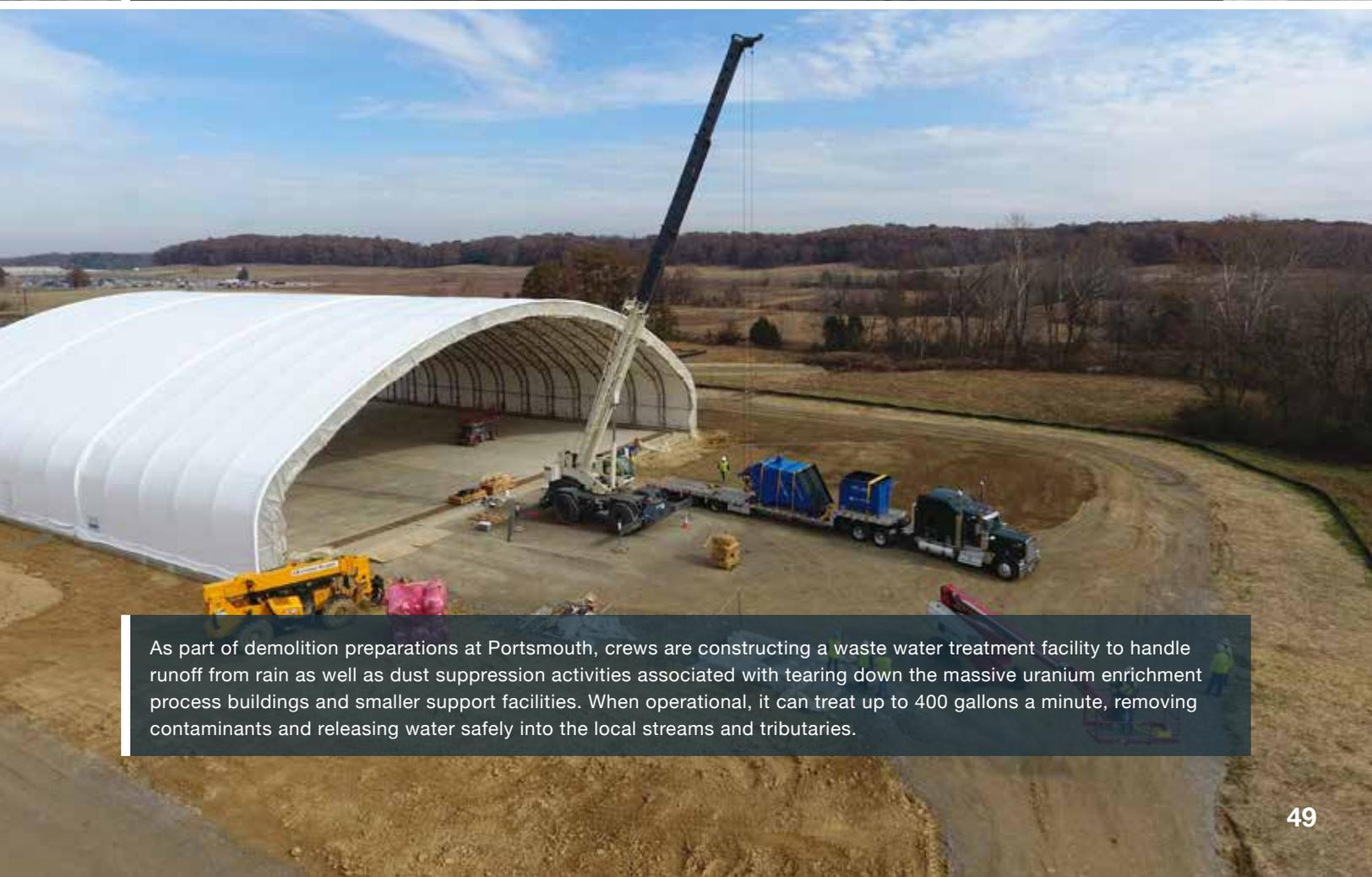
As part of demolition preparations at Portsmouth, crews are constructing a waste water treatment facility to handle runoff from rain as well as dust suppression activities associated with tearing down the massive uranium enrichment process buildings and smaller support facilities. When operational, it can treat up to 400 gallons a minute, removing contaminants and releasing water safely into the local streams and tributaries.
