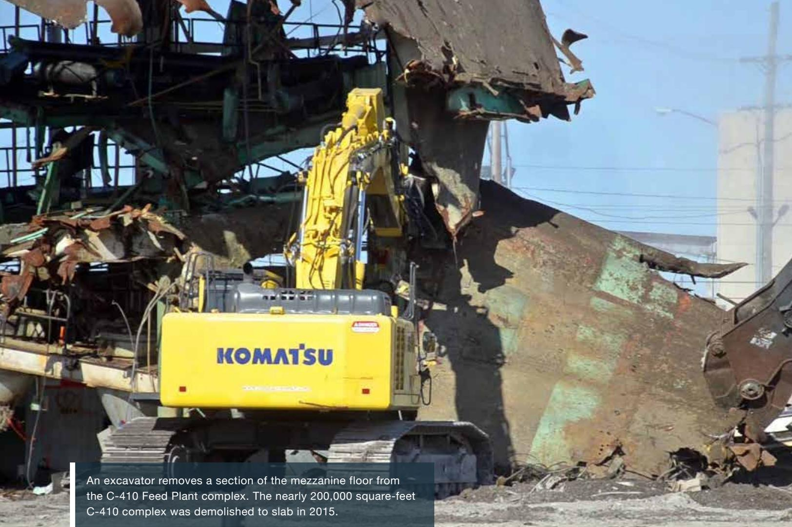
An excavator removes a section of the mezzanine floor from the C-410 Feed Plant complex. The nearly 200,000 square-foot C-410 complex was demolished to slab in 2015.
