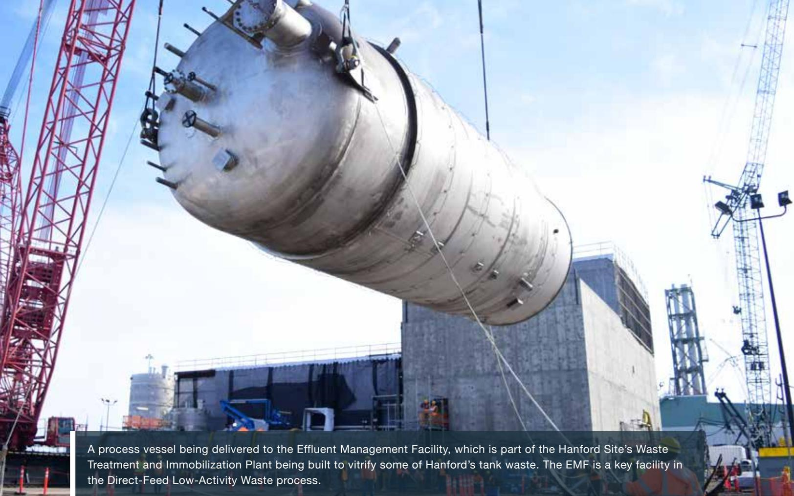
A process vessel being delivered to the Effluent Management Facility, which is part of the Hanford Site's Waste Treatment and Immobilization Plant being built to vitrify some of Hanford's tank waste. The EMF is a key facility in the Direct-Feed Low-Activity Waste process.
