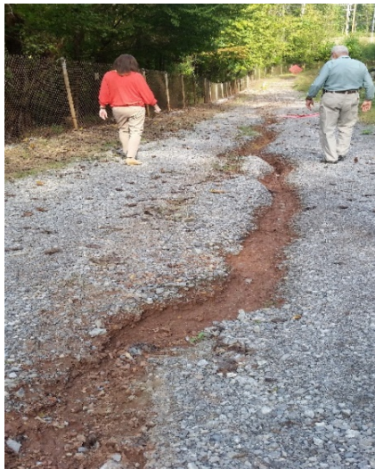
Example of washout conditions (left) on Midway Turnpike as well as improper clearance and excess vegetation (right) on Sam Grubb Road (Picture on left taken by audit team; picture on right obtained from Oak Ridge Office Year 1 Roadway Baseline Inspection report)
