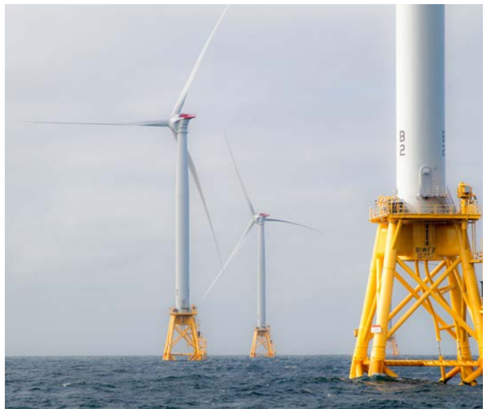
The Block Island Wind Farm, the first U.S. offshore wind farm, represents the launch of an industry that has the potential to contribute significantly to a reliable, stable, and affordable energy mix. Photo by Dennis Schroeder, NREL 41193
