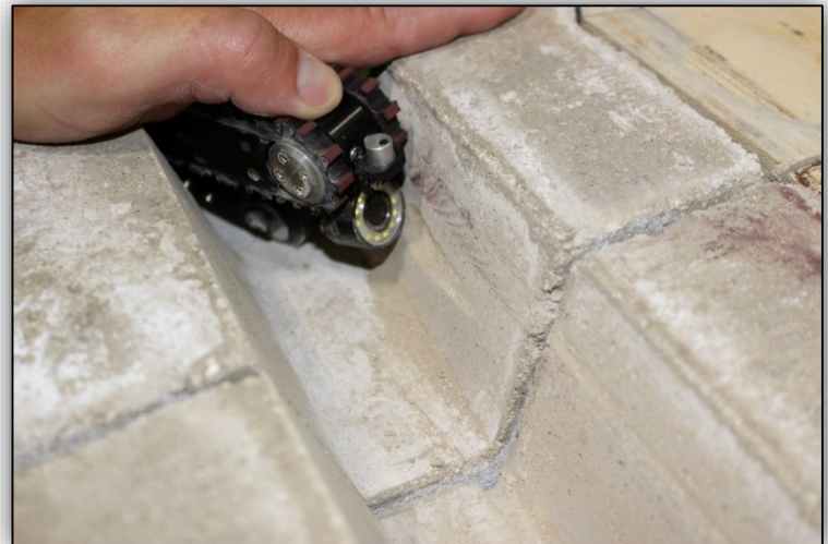
Traversed junctions only after gouging (8/7) Exposed Air Channel
