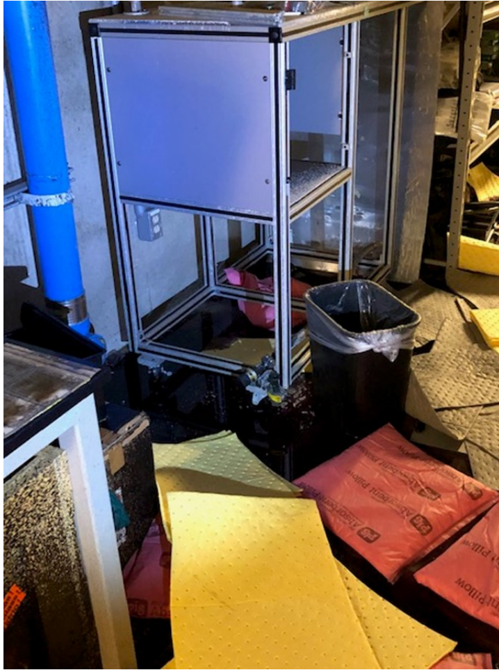
Figure 12. Sulfuric Acid Pooling Around Items on the First Floor
