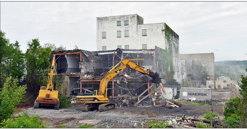
Demolition is underway on K-131, and crews will progress to K-631.
