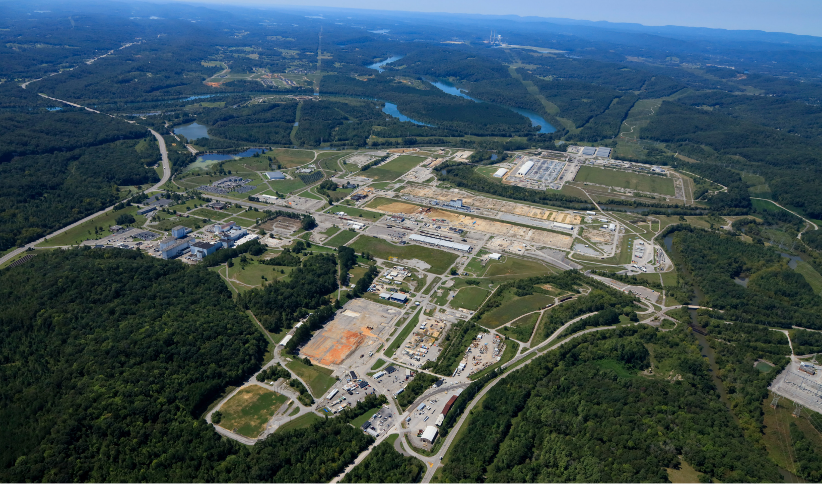
An aerial photo of East Tennessee Technology Park show progress made to remove unneeded facilities from the site and further the goal of turning most of the site into an industrial park.
