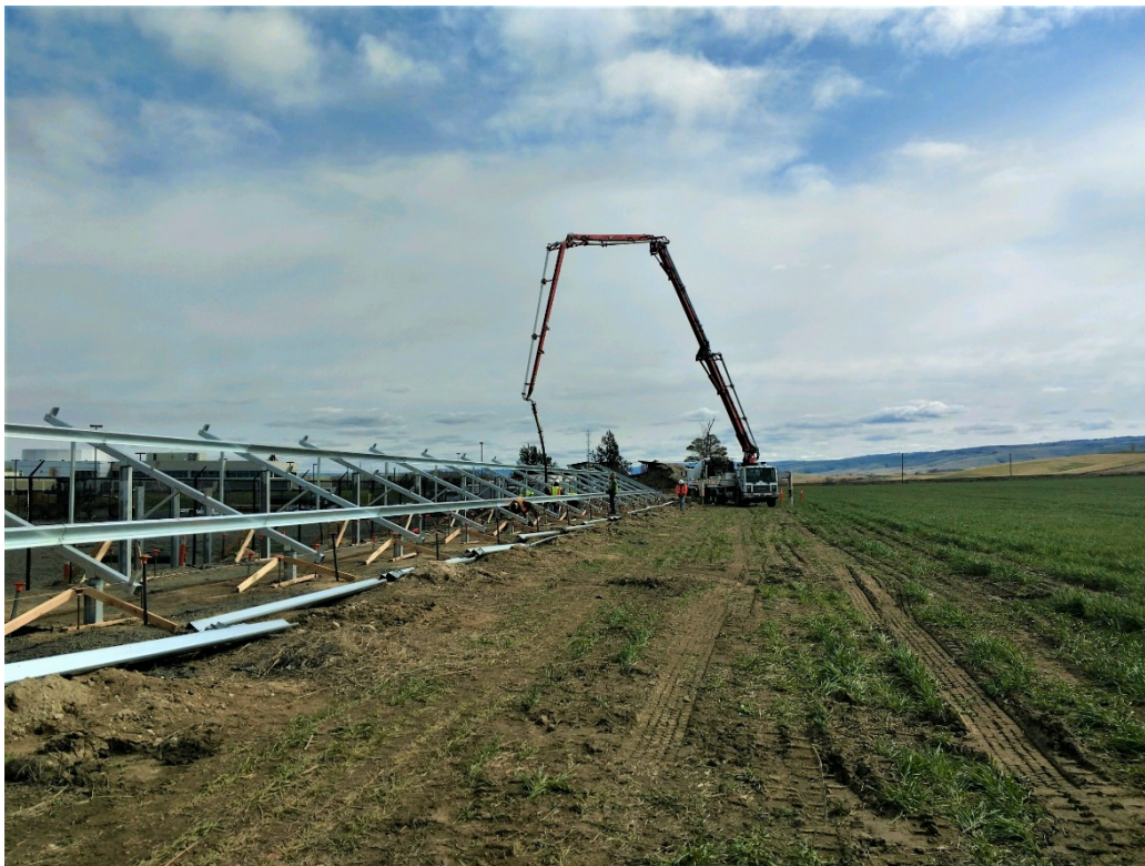
Figure 2-4: Solar PV array footings were secured in place using concrete poured with precision from a concrete pumping truck with articulating boom delivery system.
