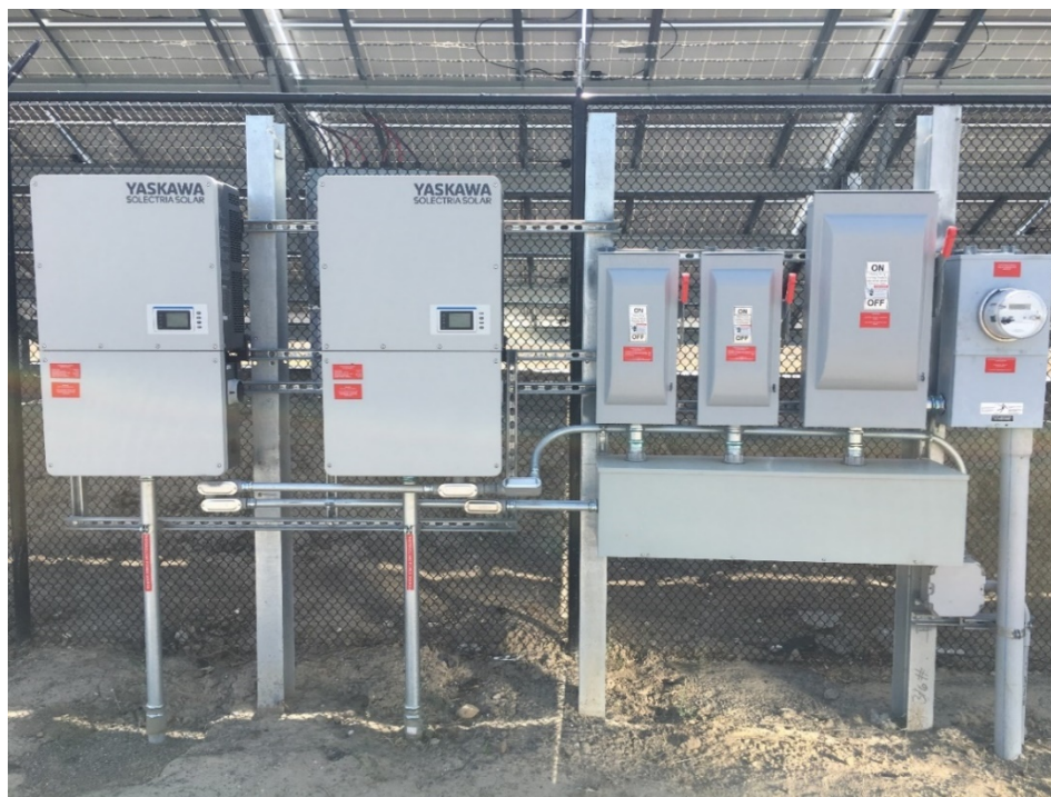
Figure 2-5: Equipment rack for the solar PV array system showing Yaskawa Solectria Solar PVI 50/60TL inverters (left), associated switchgear and meter (right).
