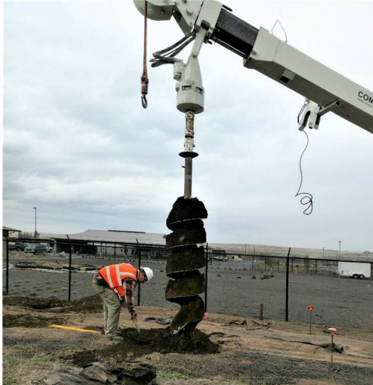
Figure 2-3: Excavation of holes via hydraulic auger. The holes, having a depth of 10 ft, were used to secure solar PV array footings.
