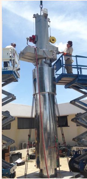
Workers in Jamaica load HEU into the transportation cask for return to the U.S. – Photo courtesy of NNSA.
