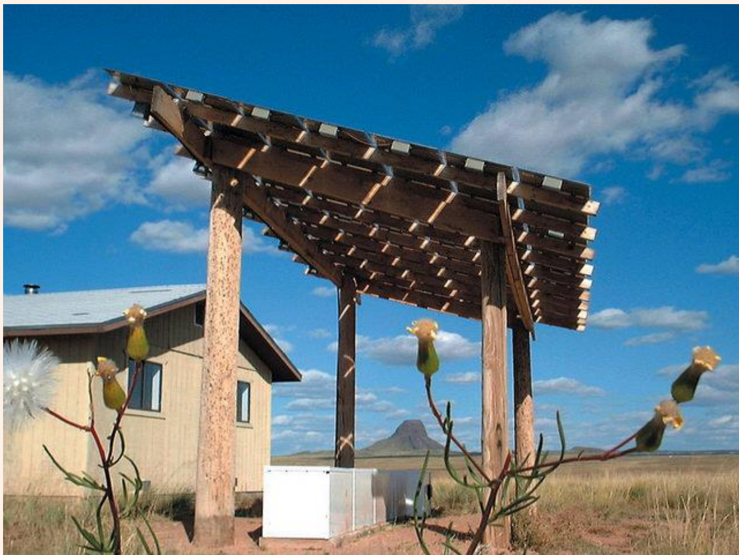
Solar Electric Array: Solar electric array on off-grid Navajo home in Arizona.
