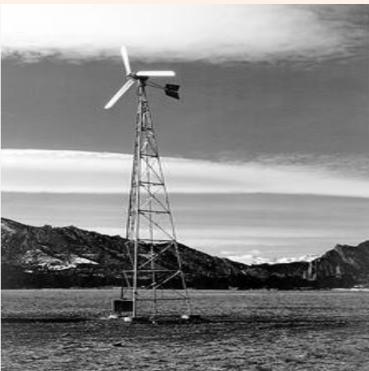
The Dunlite turbine, with 3 blades and a 12 foot rotor diameter, was tested at Rocky Flats. (circa 1977)
