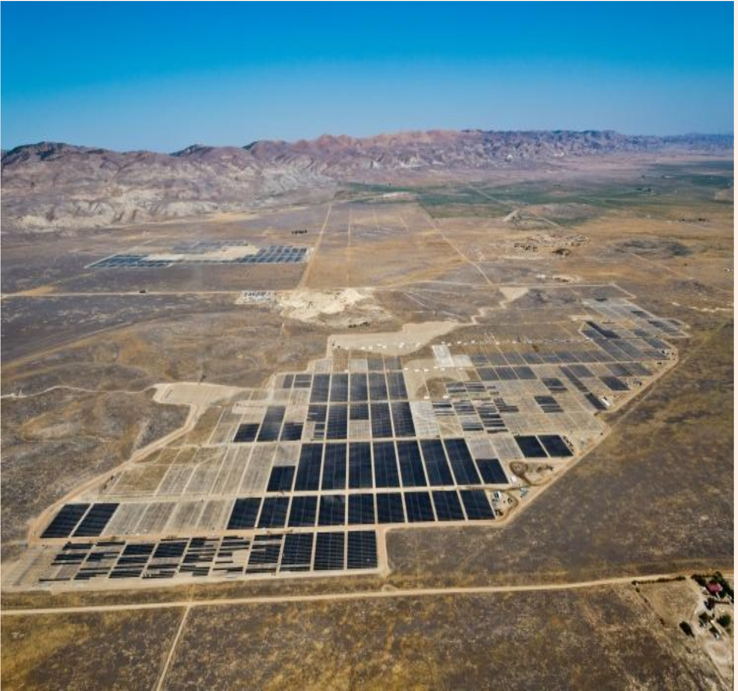
Super Sized Solar Grid – An aerial view of the California Valley Solar Ranch, that has a capacity of 250 megawatts -- enough energy to power the equivalent of every home in San Luis Obispo County. | Photo courtesy of SunPower.
