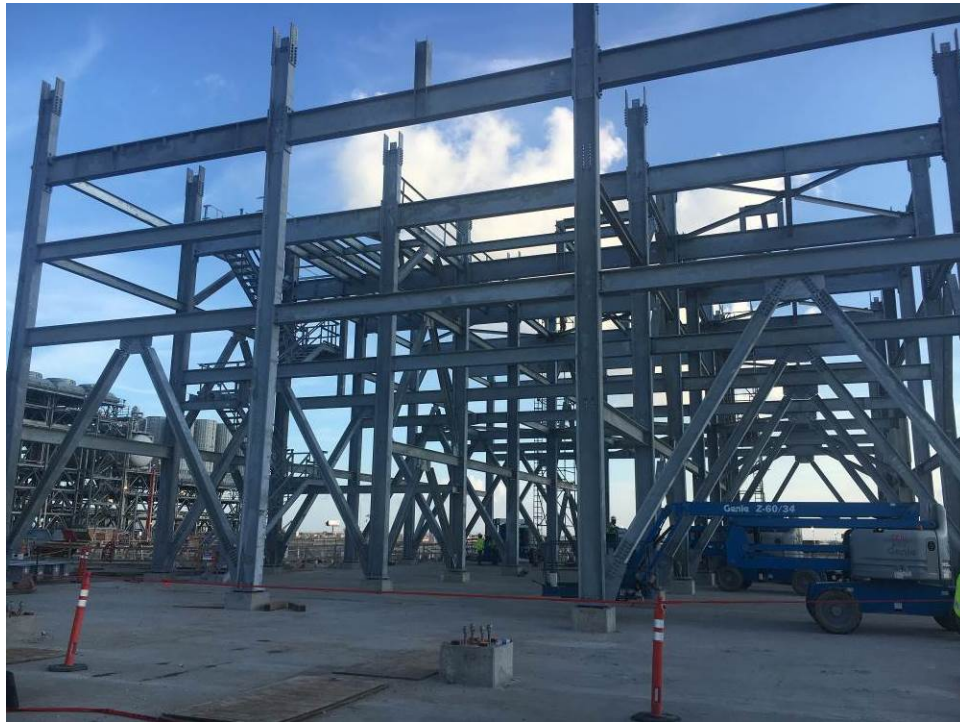
Steel Erection underway at Cryo Area
