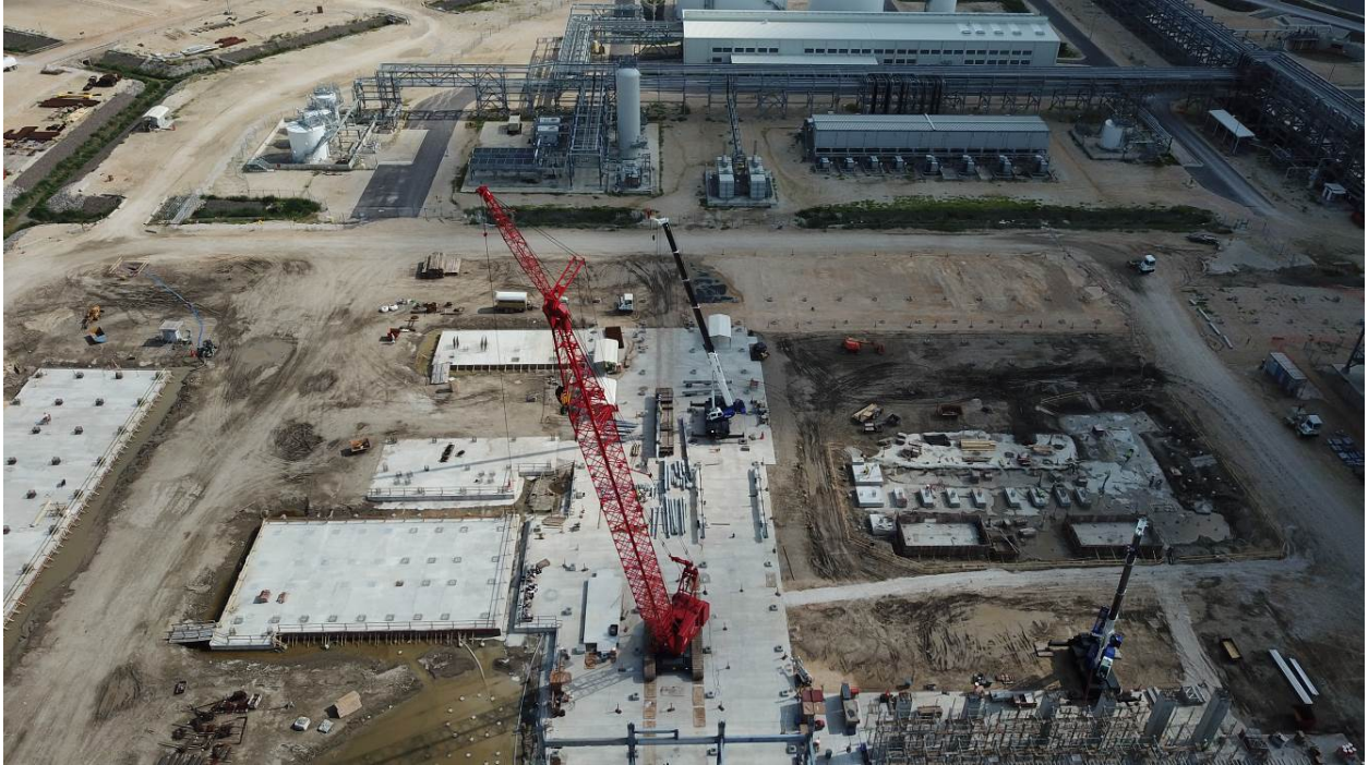
Concrete Foundations progress at South Side of Train 6
