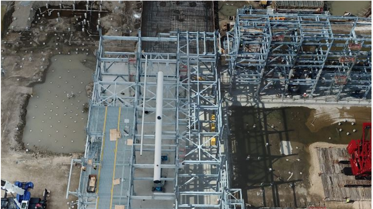
1 st Aboveground Pipe in Cryo Rack Area
