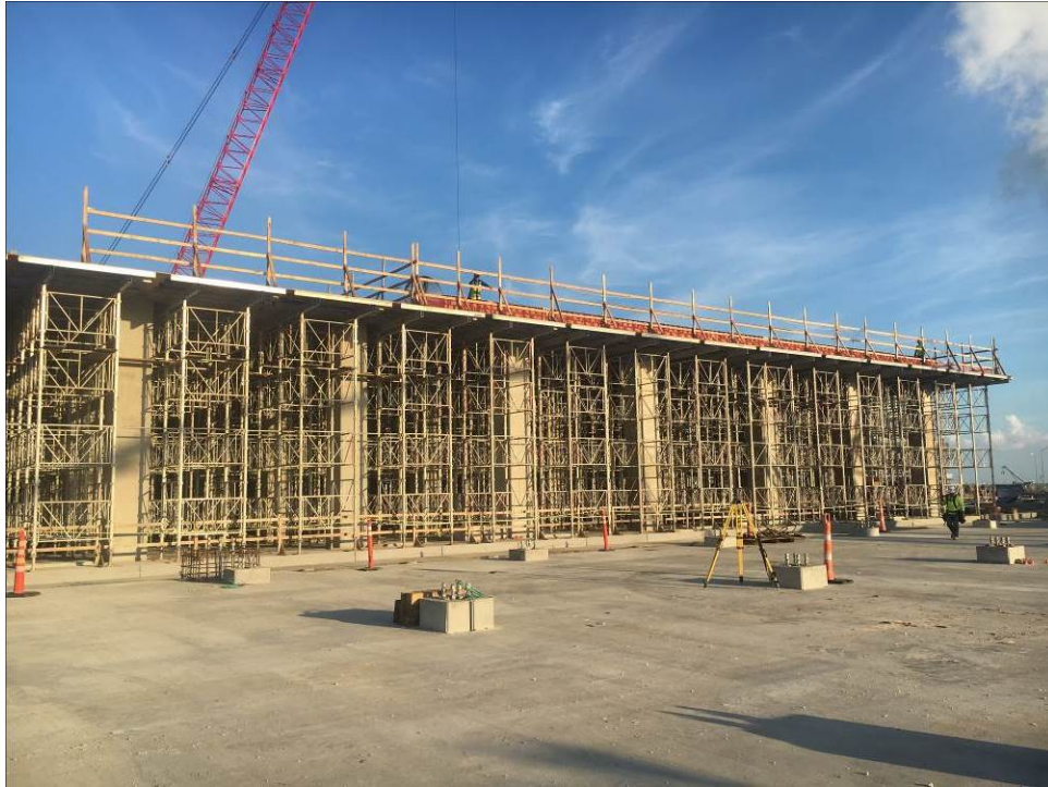
Compressor Area progress
