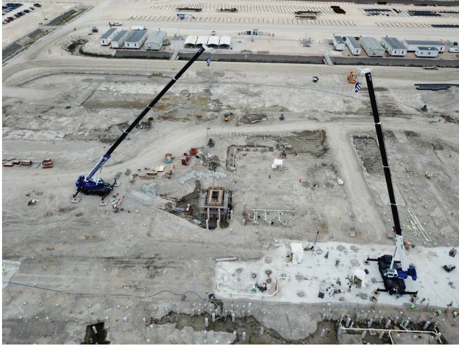
Hot Oil and Amine Underground Pipe and Sumps Progress
