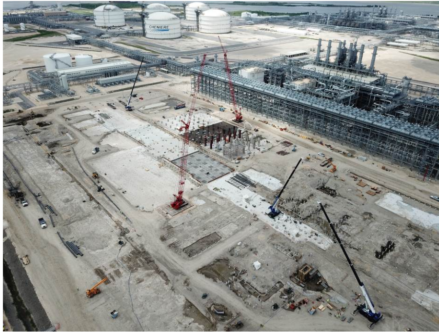
Train 6 – Aerial View
