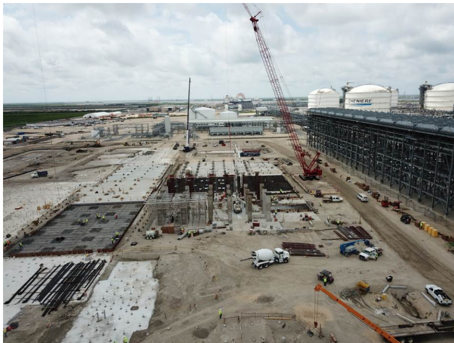
Concrete works in Compressor Area and Cryo Area
