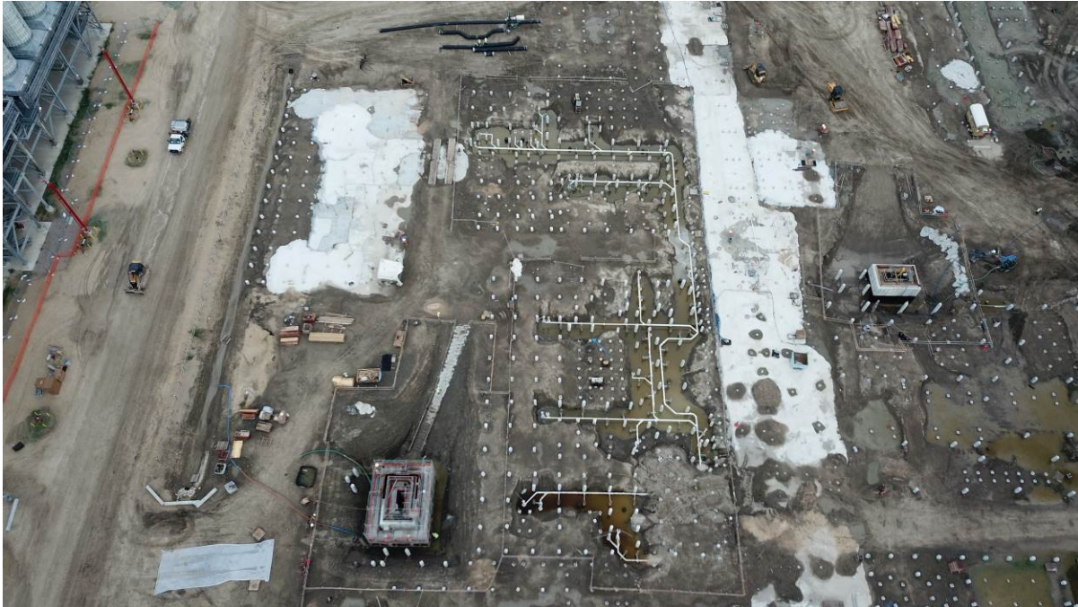
Hot Oil and Amine Underground Pipe and Sumps Progress
