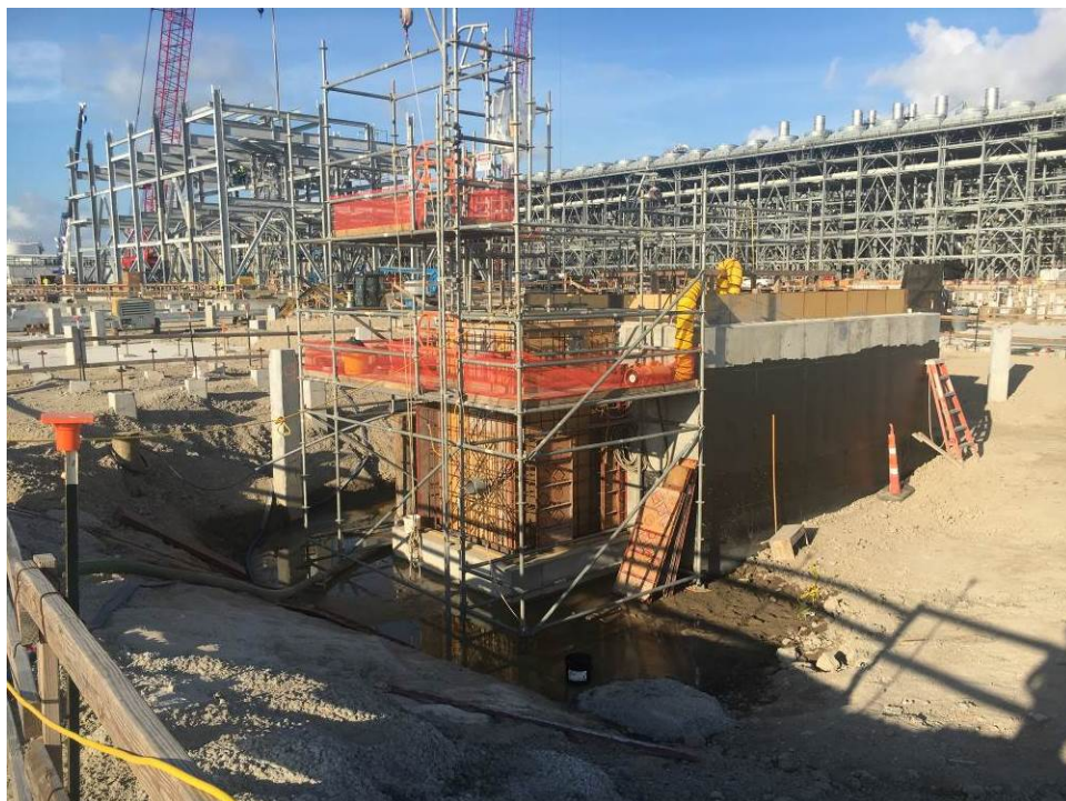
Valve Box progress at Hot Oil Sump
