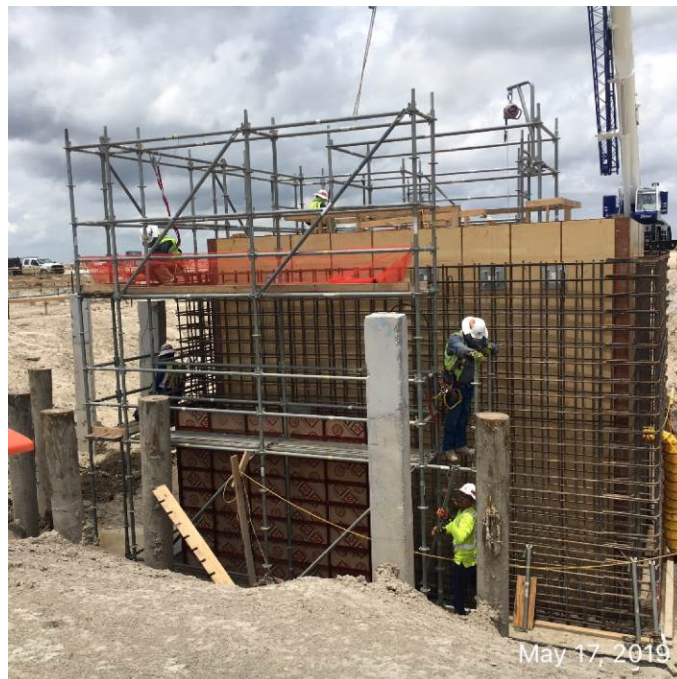
Wall Construction at Hot Oil Sump
