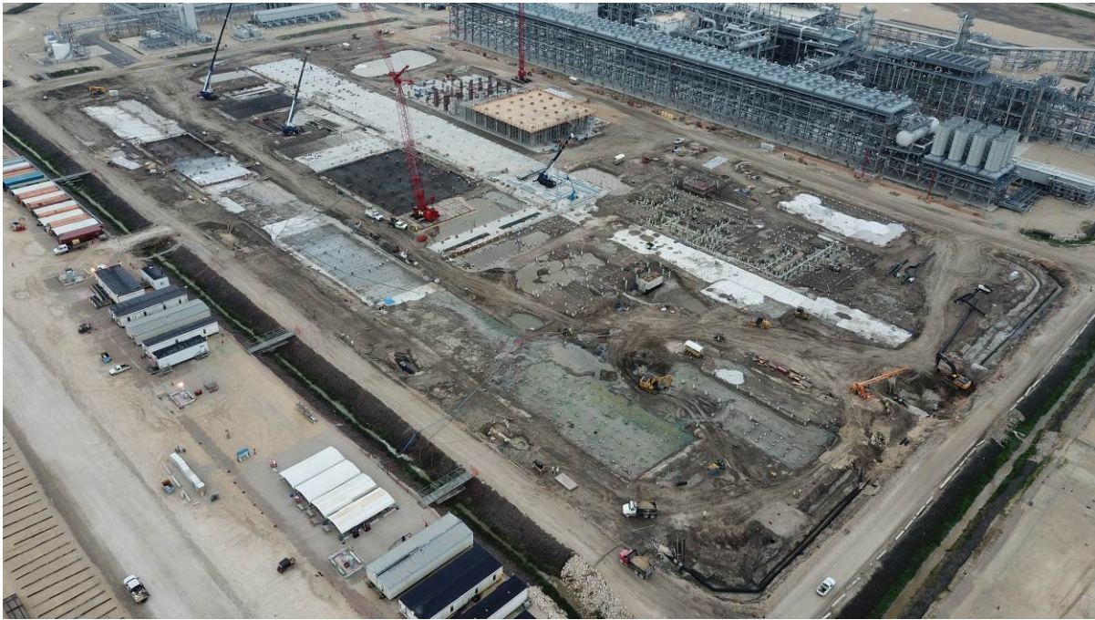
Train 6 – Aerial View
