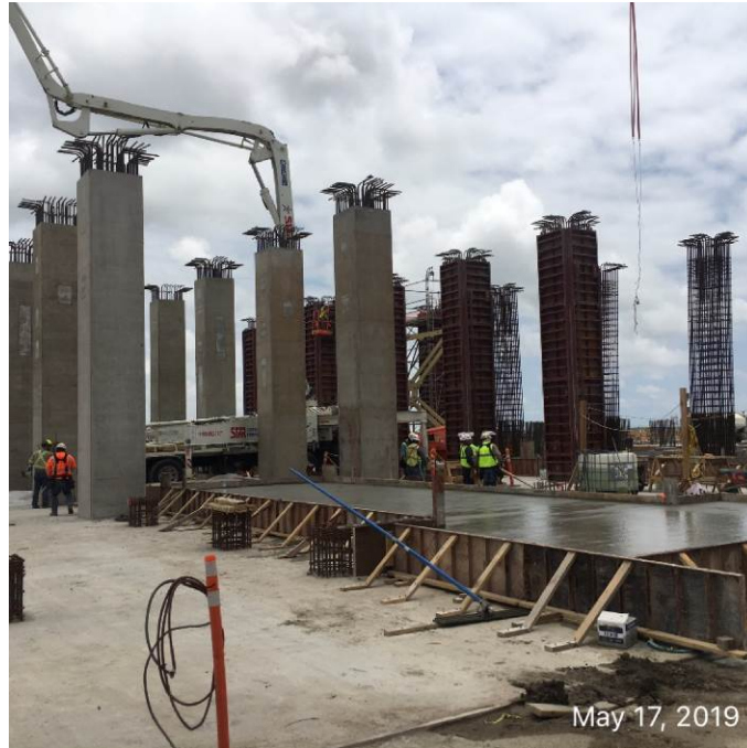
Concrete Columns and Equipment Pads at Propane Section of Compressor Area
