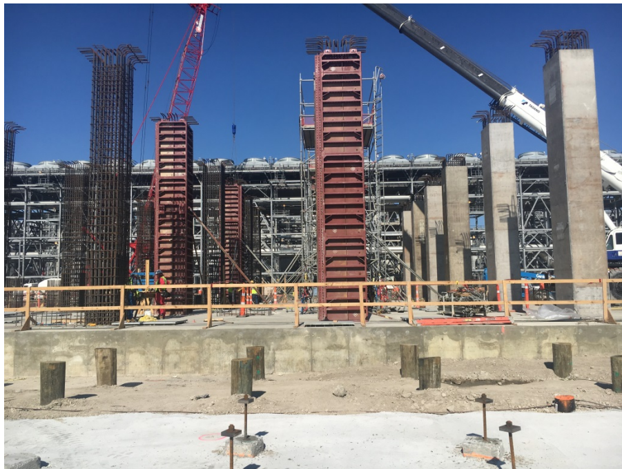
Concrete Columns in Propane Section of Compressor Area
