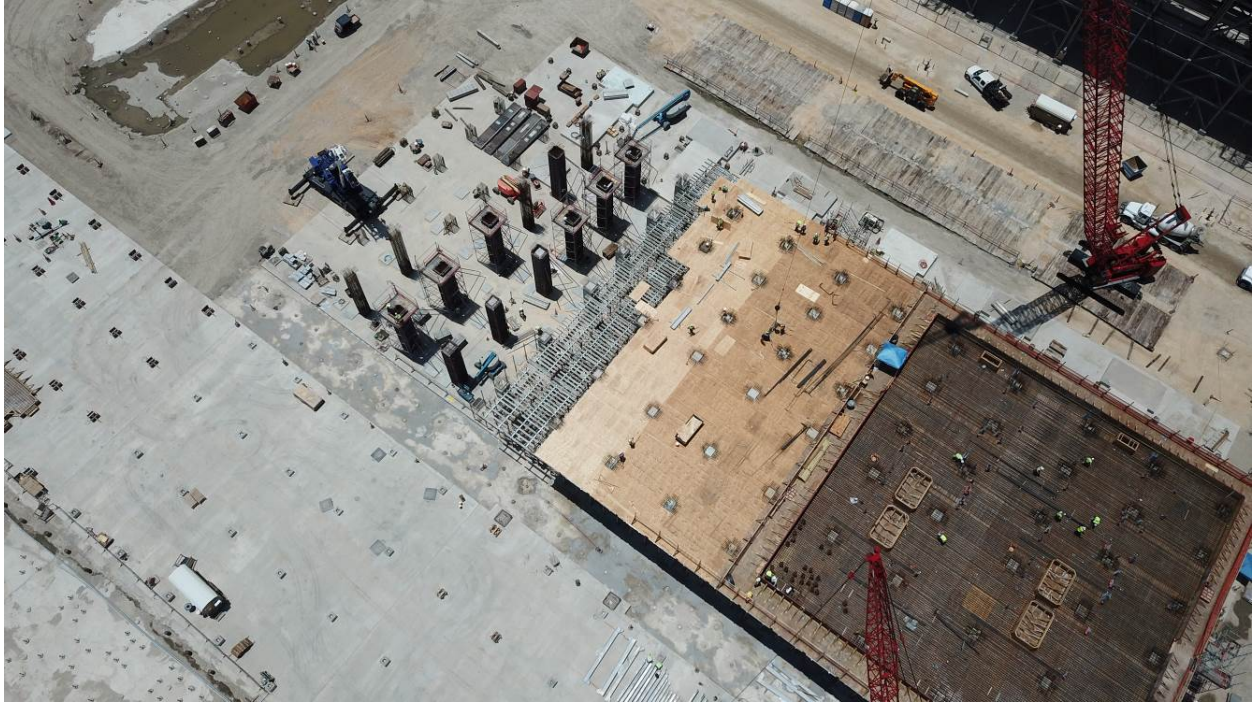
Aerial View of Compressor Area progress
