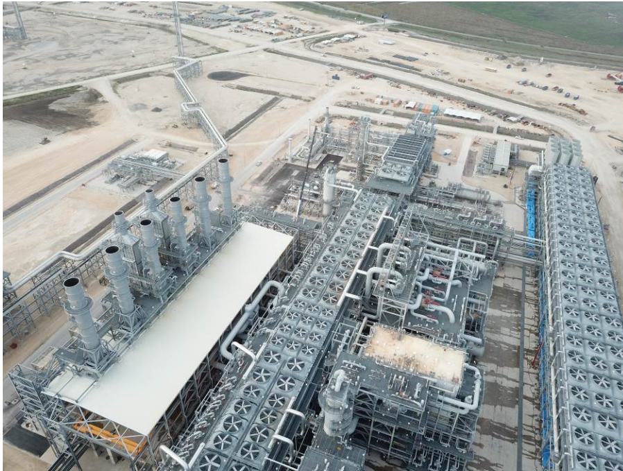
Train 5 – Aerial View
