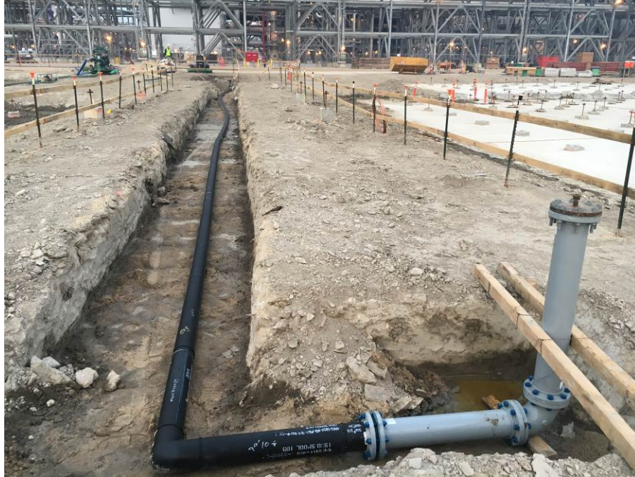
Train 6 – Installed UG Firewater Pipe
