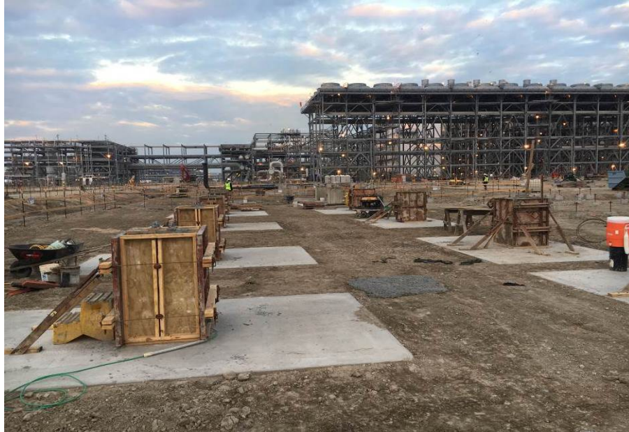
Train 6 – R10 Pipe Rack Pile Caps and Pedestals Complete
