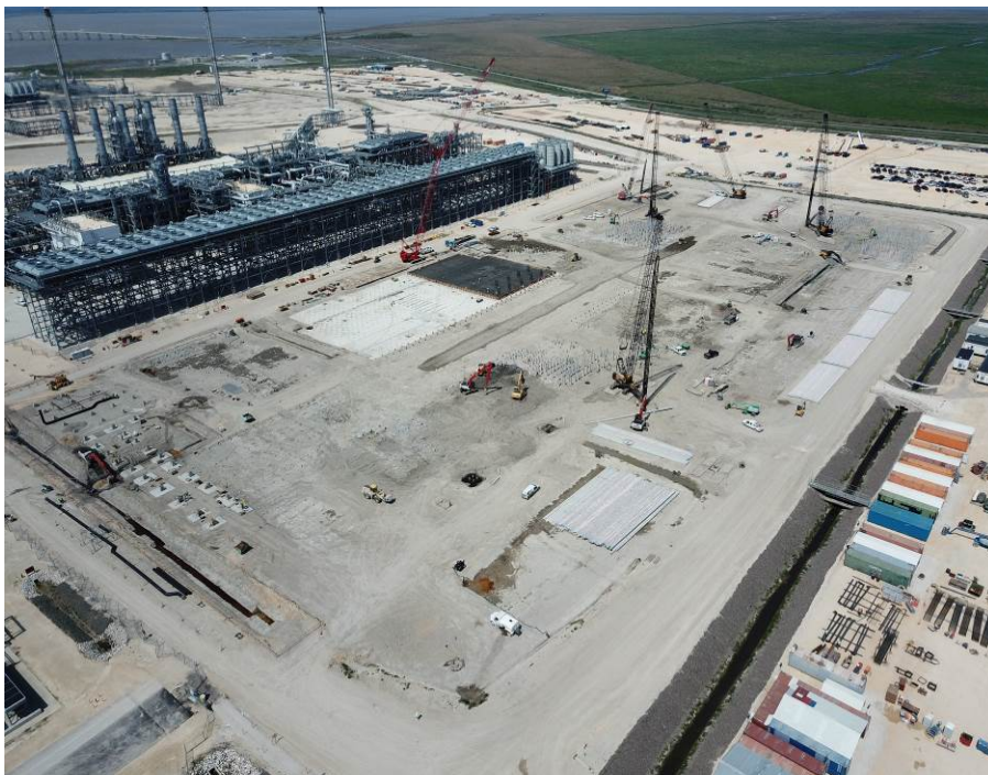
Train 6 – Aerial View
