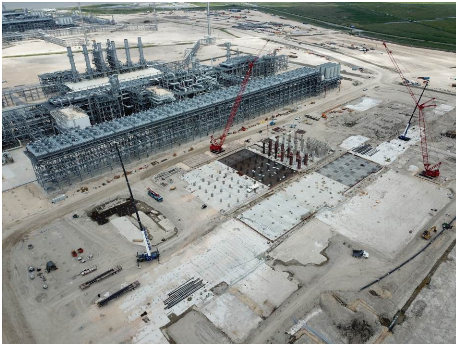
Aerial View of Concrete Progress
