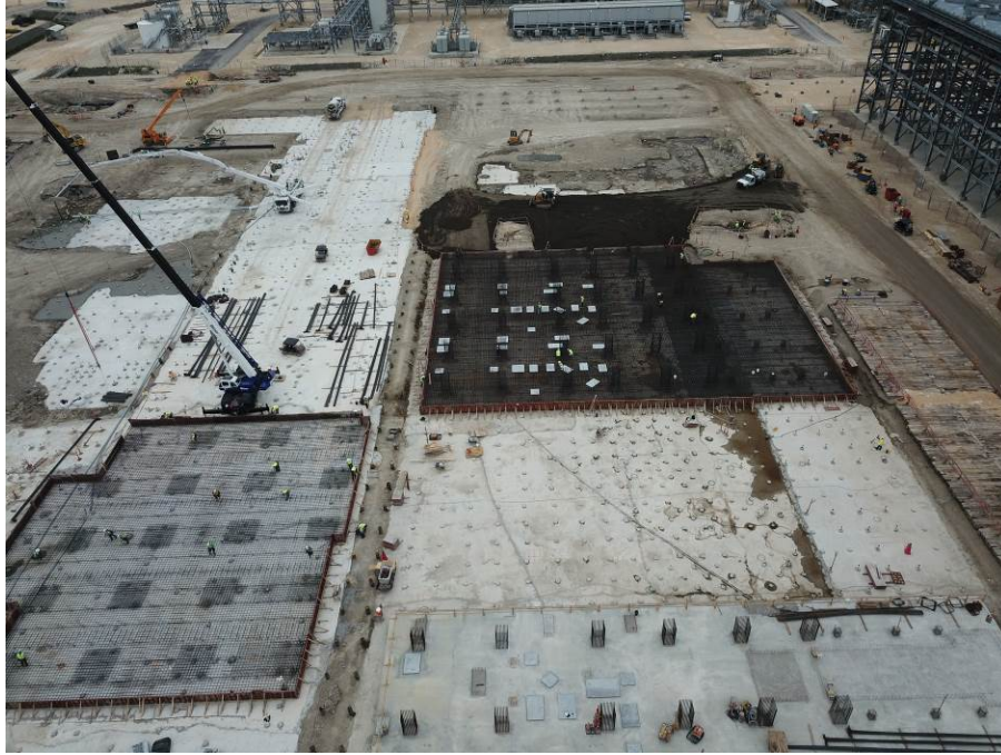
Train 6 – Aerial View
