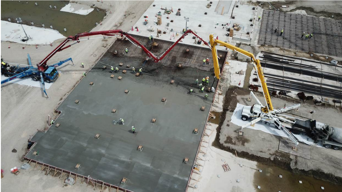
Concrete Base Slab at Section 1 of Cryo Area
