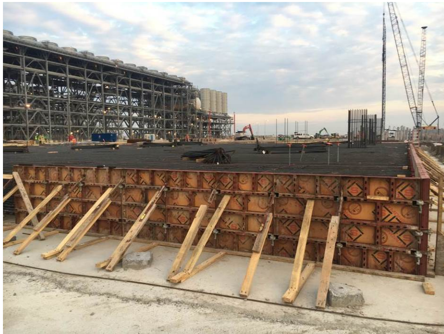
Train 6 – Propane Mat Rebar and Formwork Compressor Area
