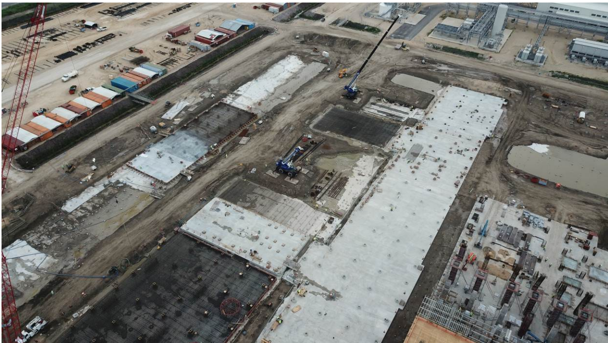
Concrete works across Train 6
