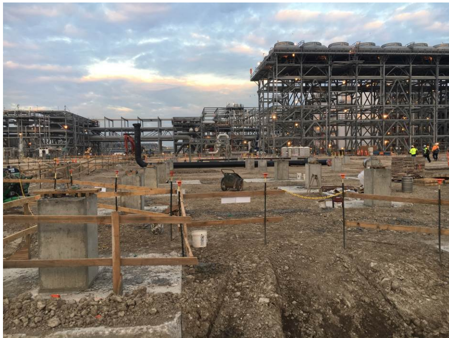
Train 6 – UG Firewater Pipe Staging in R10 Rack ready for Installation
